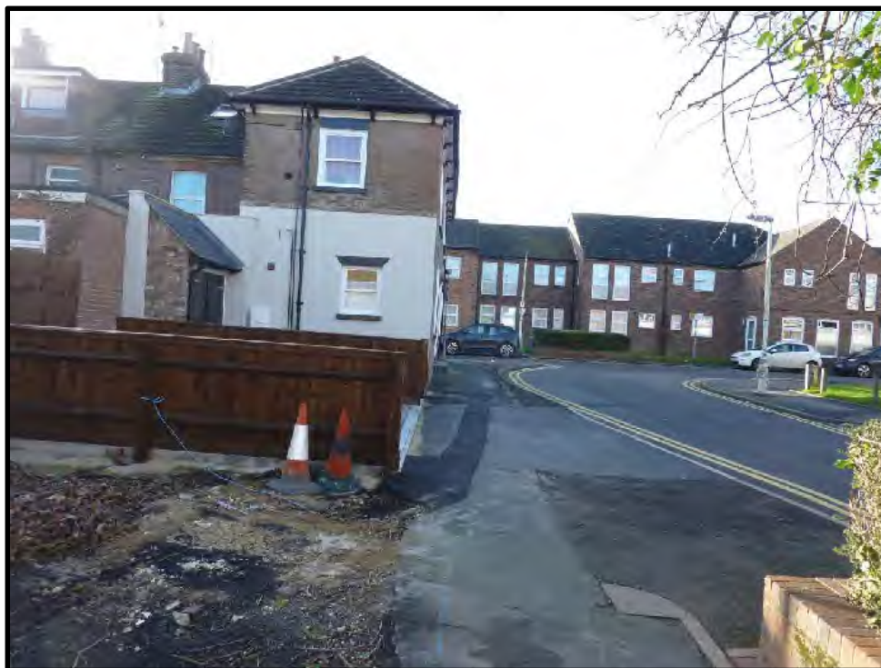
Plate 1: The PDA, from the north-east (21 Regent Street and 66-70 Edward Street in the background to the left)
