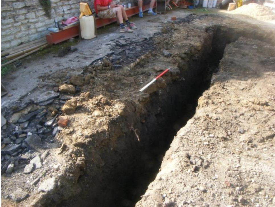
a) Alluvial layer beneath patio remains. Looking South. Scale 1m.
