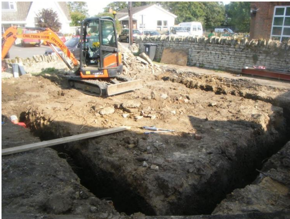
General view of garage foundations. Looking East.
