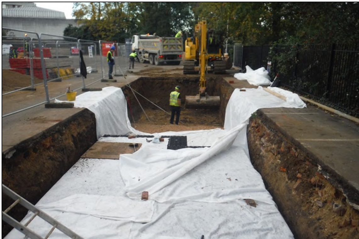
Image 6: Soakaway drainage under construction Looking west-south-west
