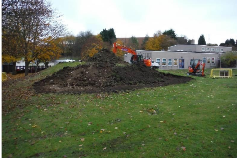
Excavation of the earth mound prior to the trial trenching
