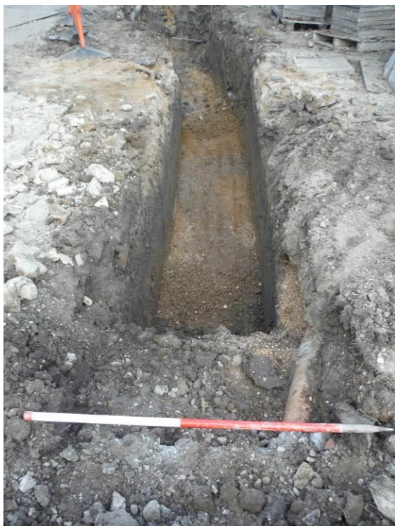
Infiltration Trench 1 from SW 1m scale
