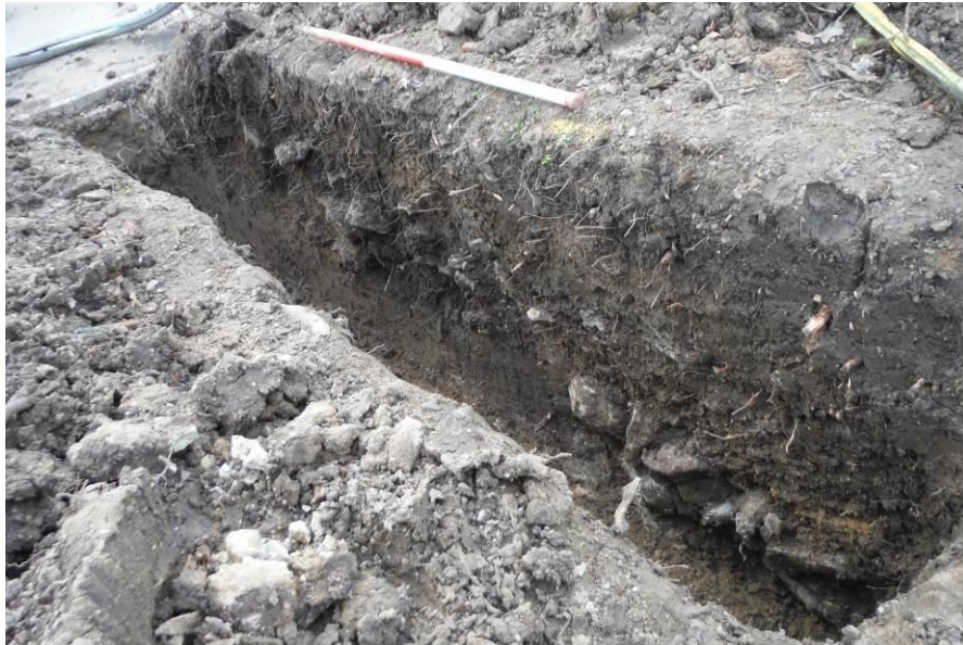
Section 2 – Water pipe trench from east 1m scale
