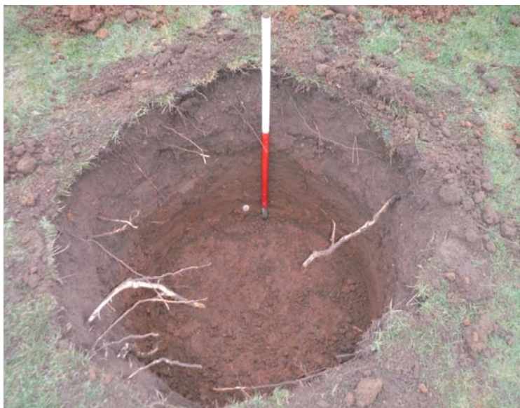
Foundation pad excavated by mechanical auger (1m scale)
