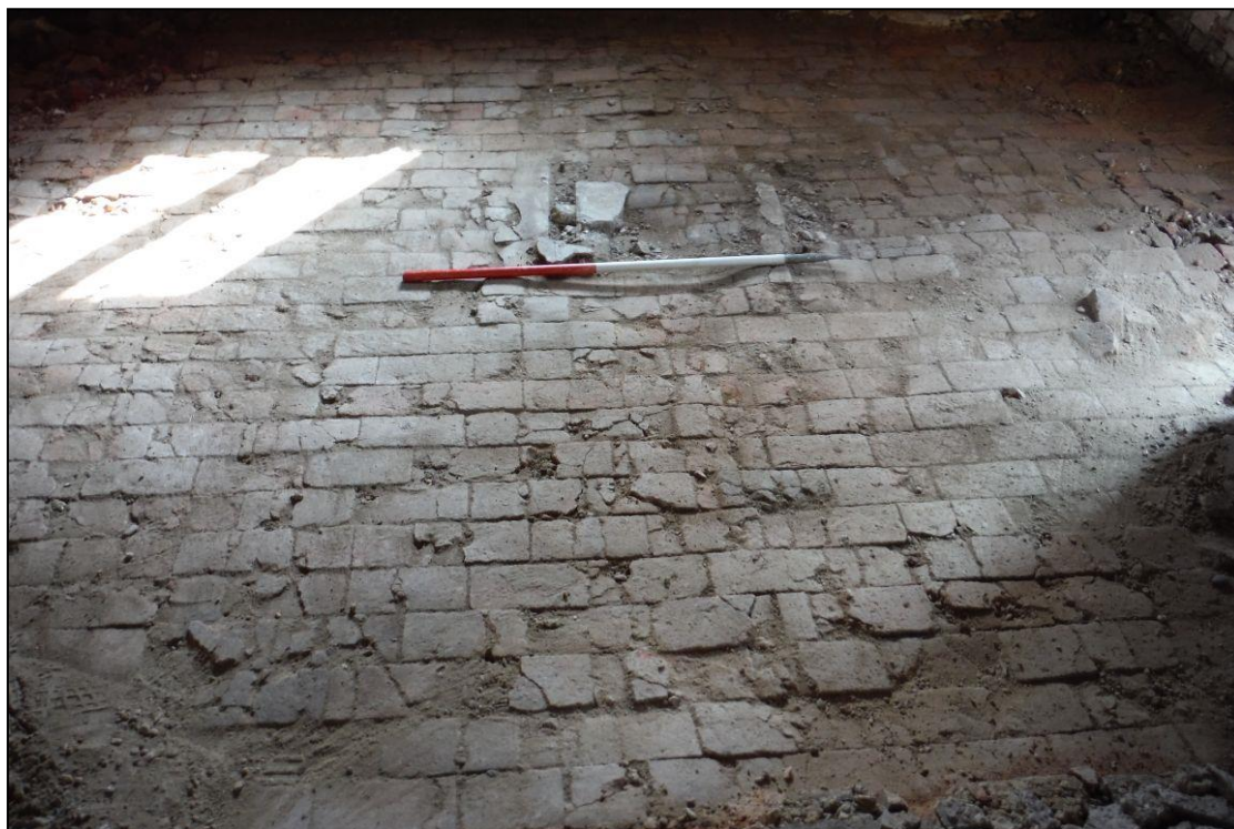
Image 5: Building 1, interior of south-west compartment
