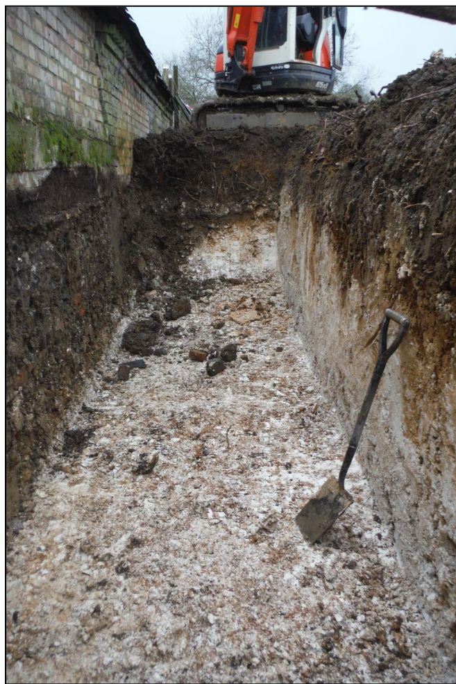
Image 3: Groundworks to rear of Building 3
