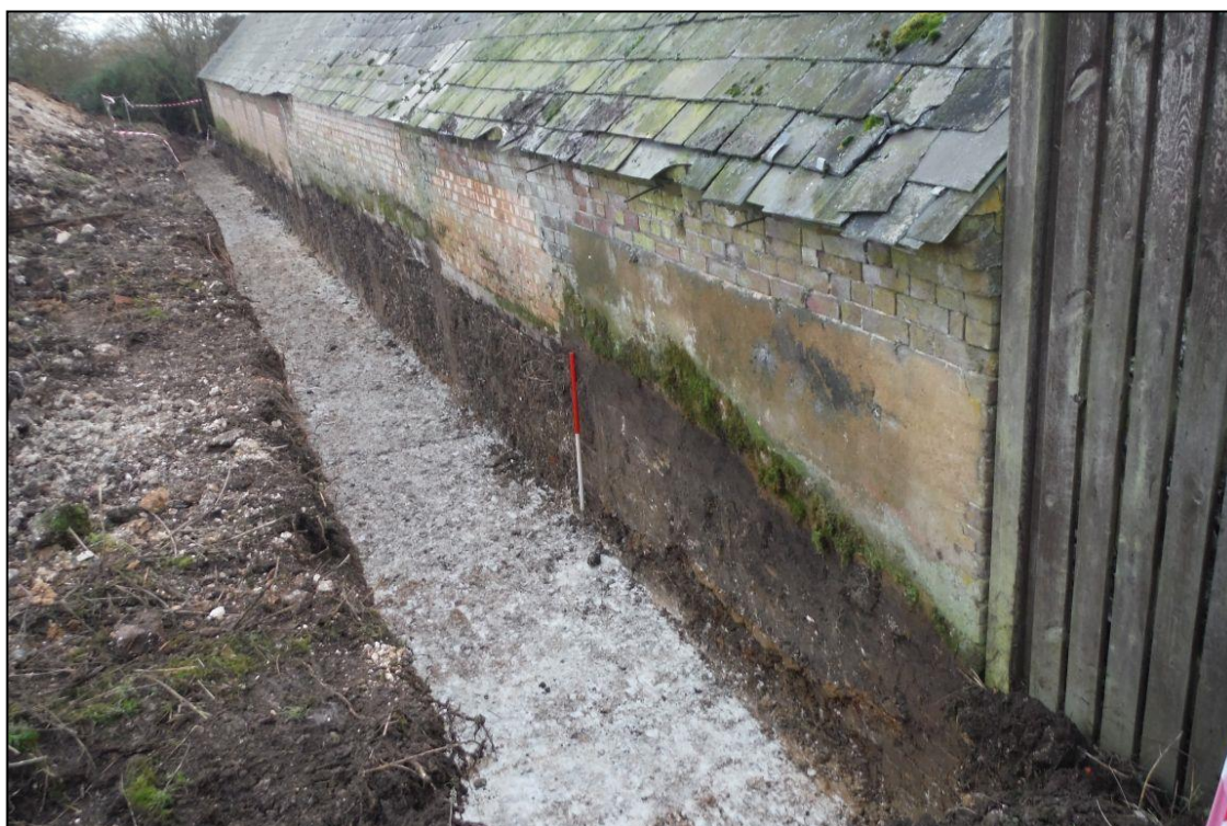
Image 2: Groundworks to rear of Building 3
