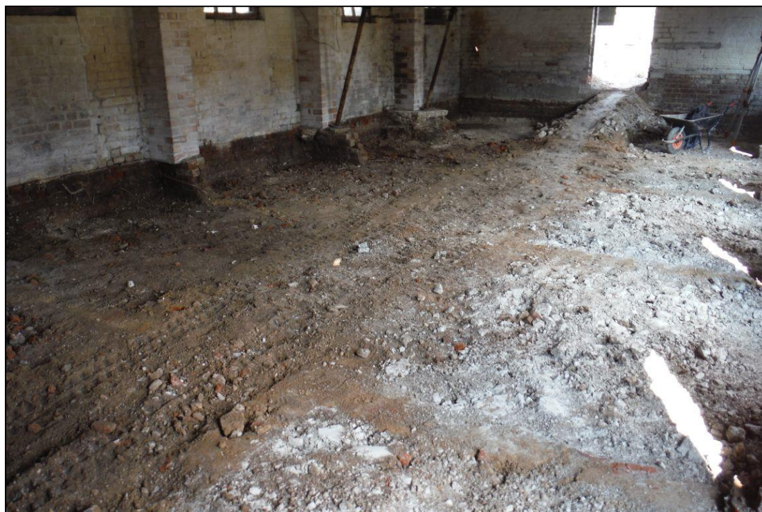
Image 4: Building 1, interior of main compartment
