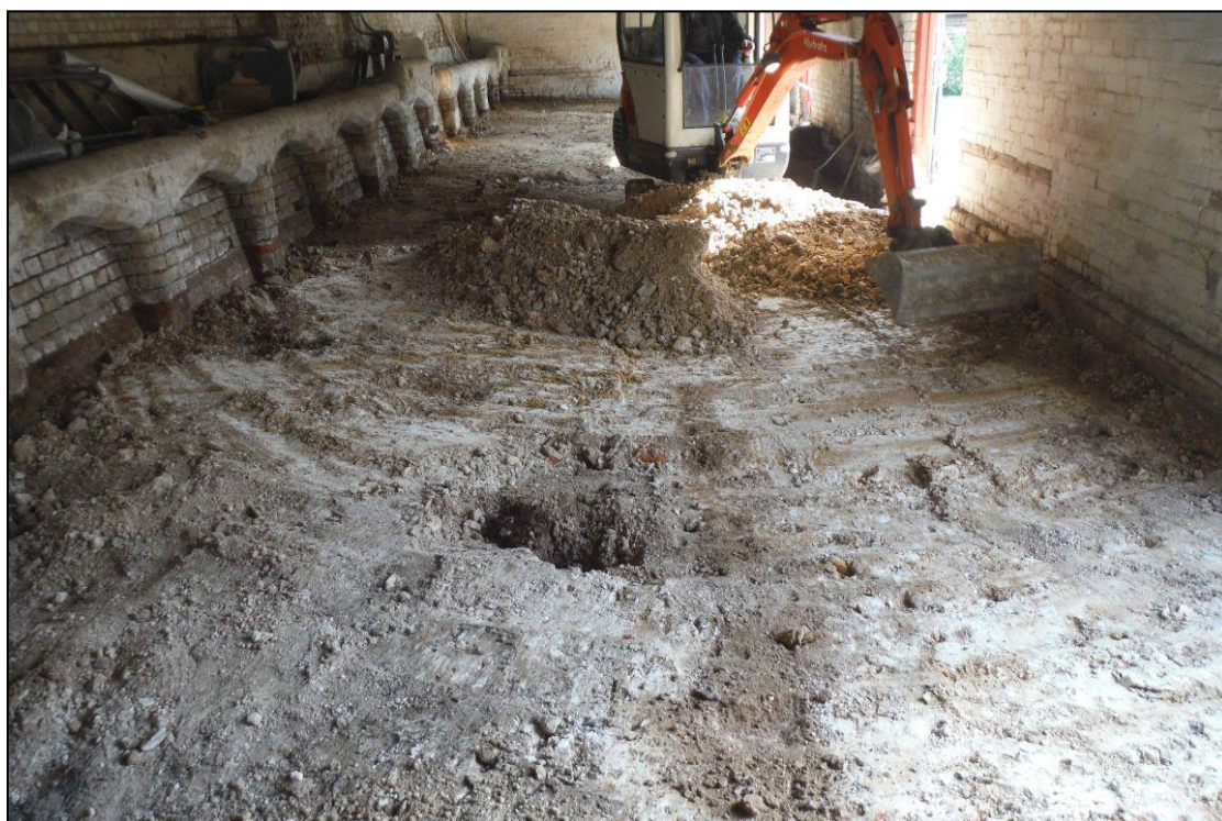
Image 6: Building 3 interior during groundworks
