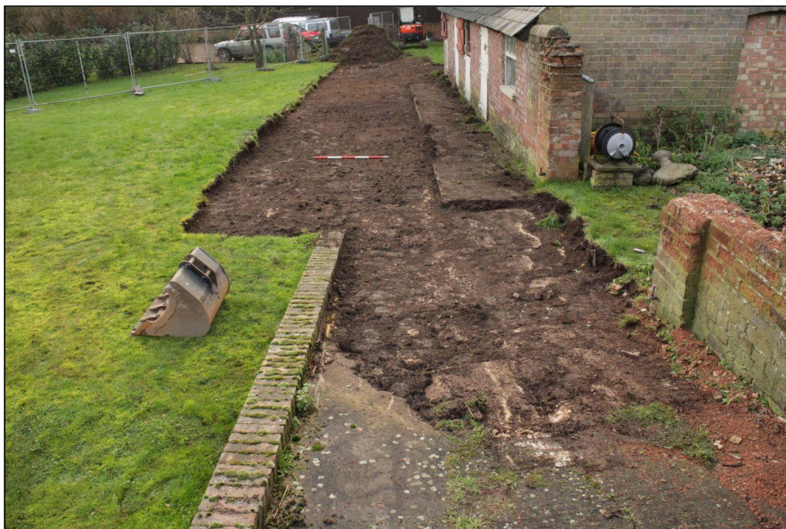
Image 1: Groundworks in front of Building 1
