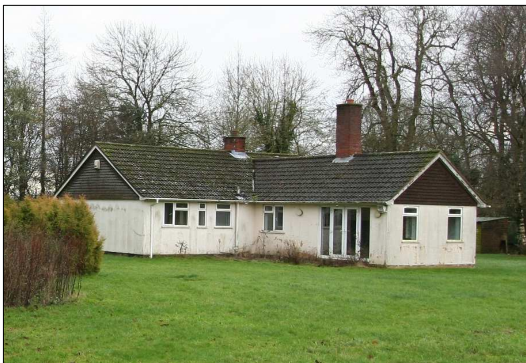
Figure 18: Existing bungalow in the PDA, rear elevation (Looking south-east)
