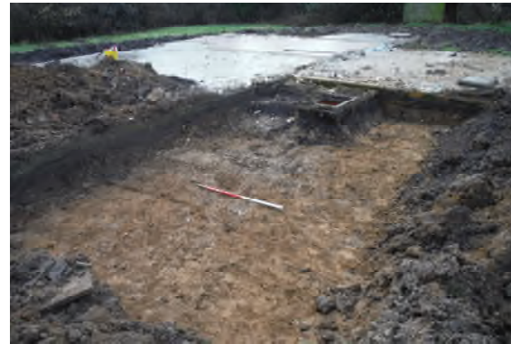
House trench showing manhole. Looking SE. Scale 1m
