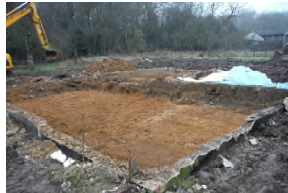
House trench, showing existing foundations. Looking SW.
