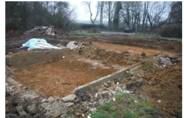
House trench, showing existing foundations. Looking NE.
