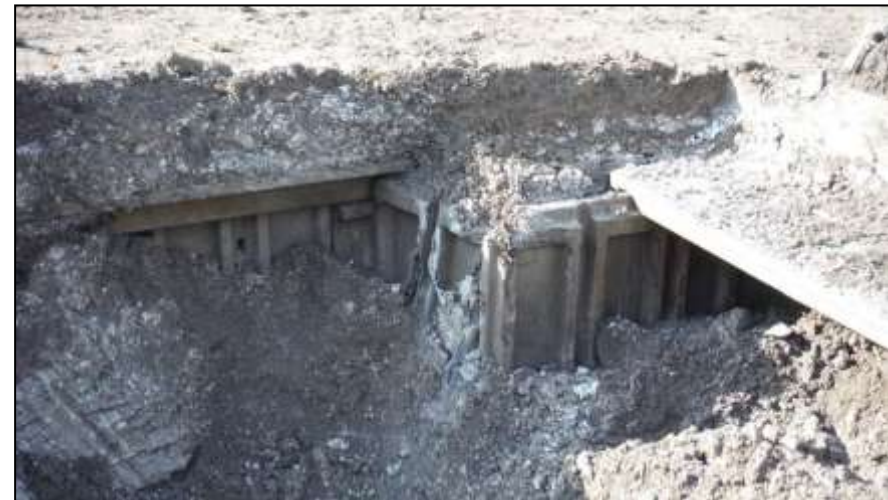
Plate 8: Wall and roof construction of the air raid shelter [1042], looking west
