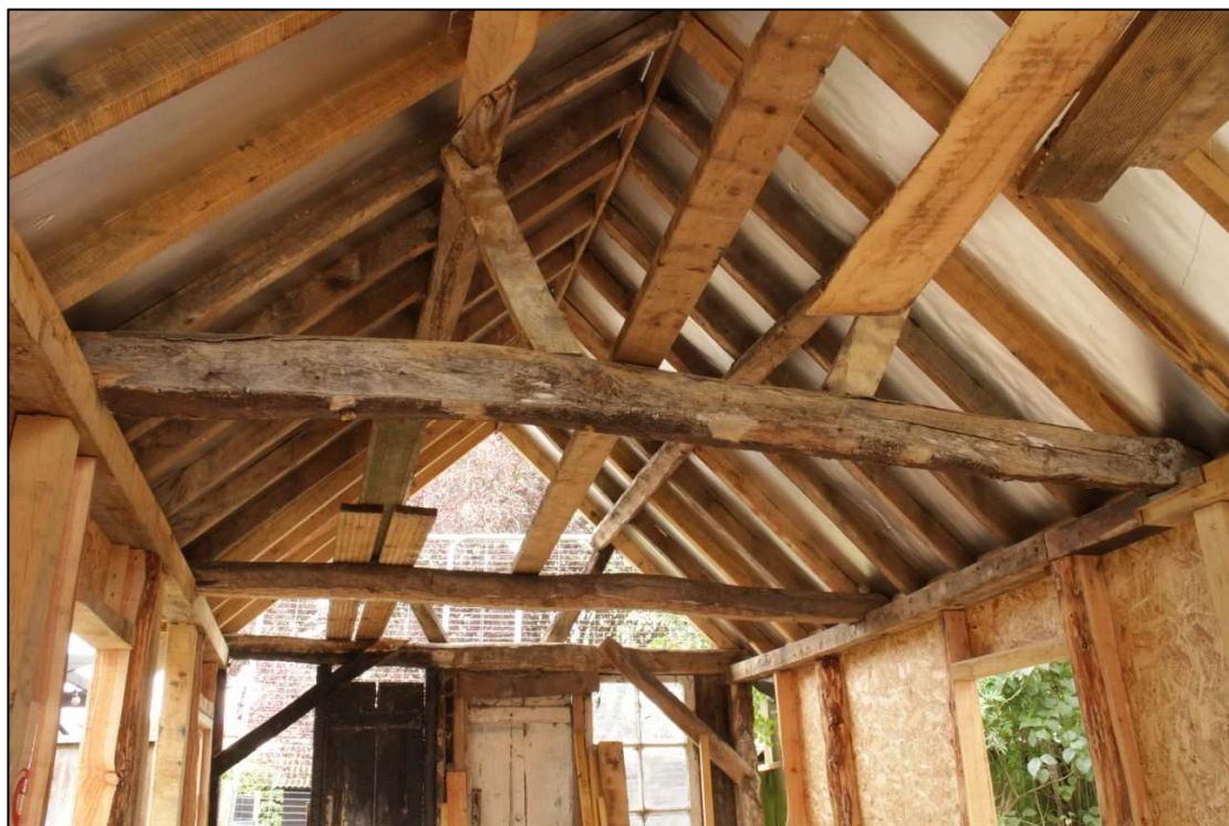
Image 9: Roof structure viewed looking northwards
