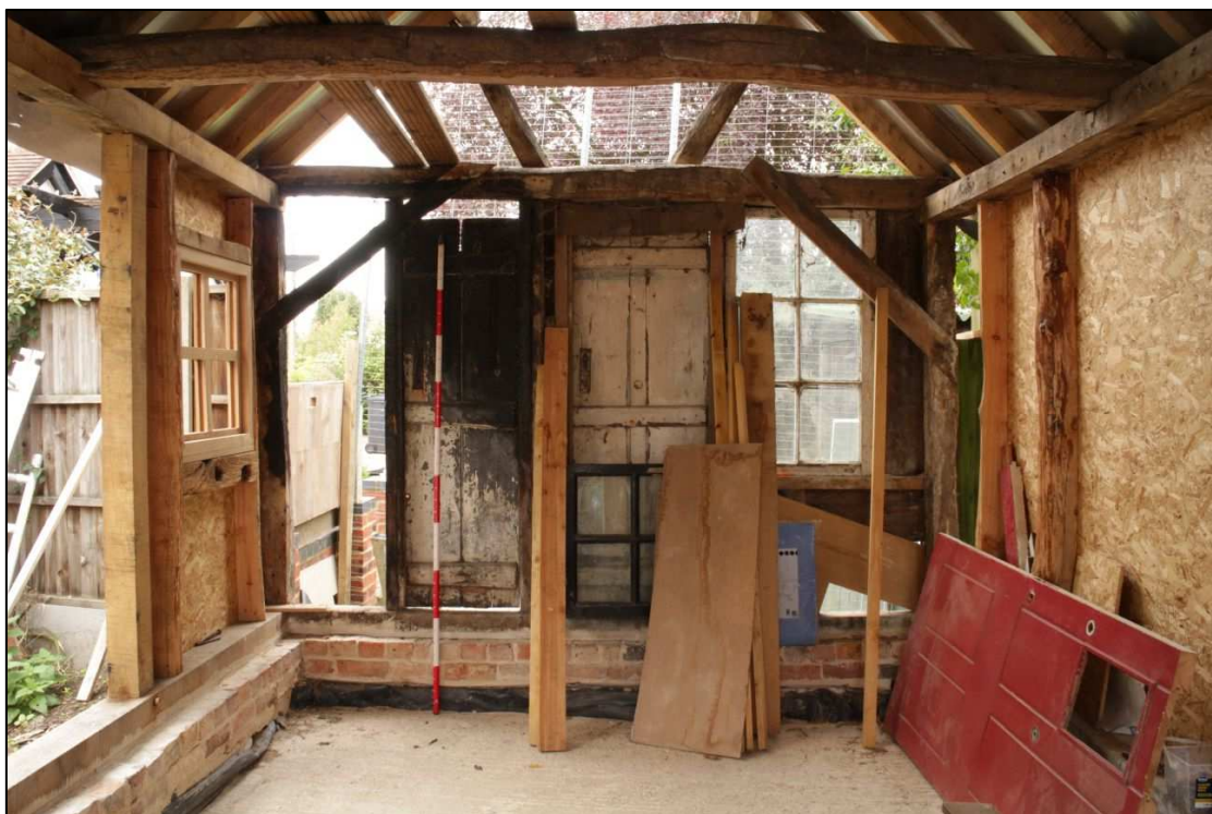
Image 3: Interior detail of north wall
