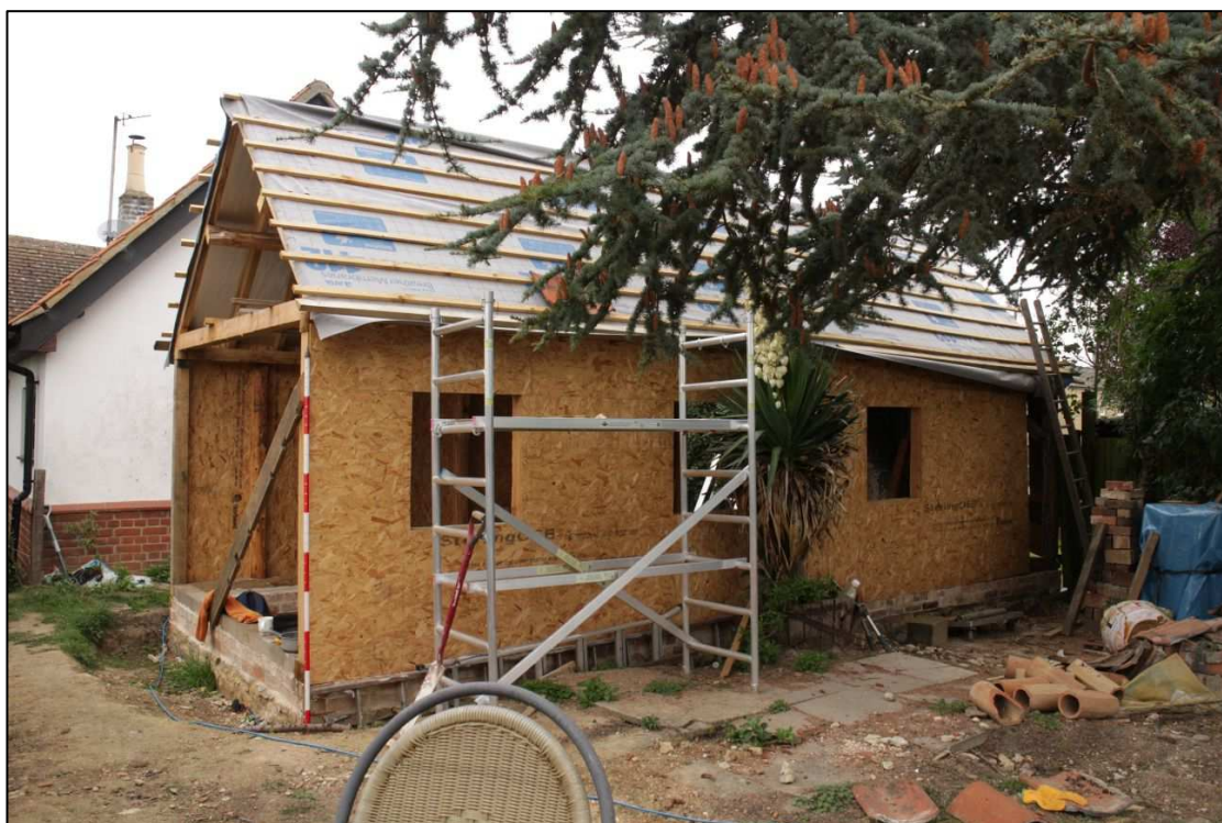
Image 1: Exterior of barn, looking north-west
