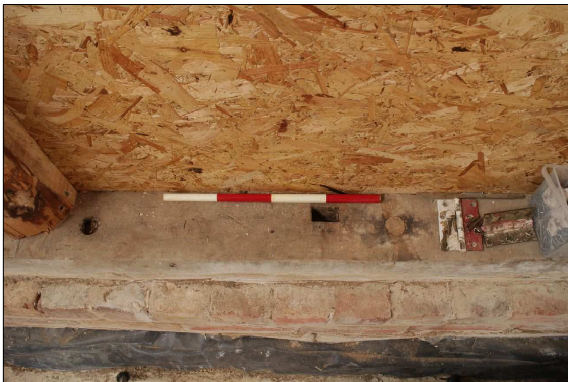
Image 5: Sill beam in east wall
