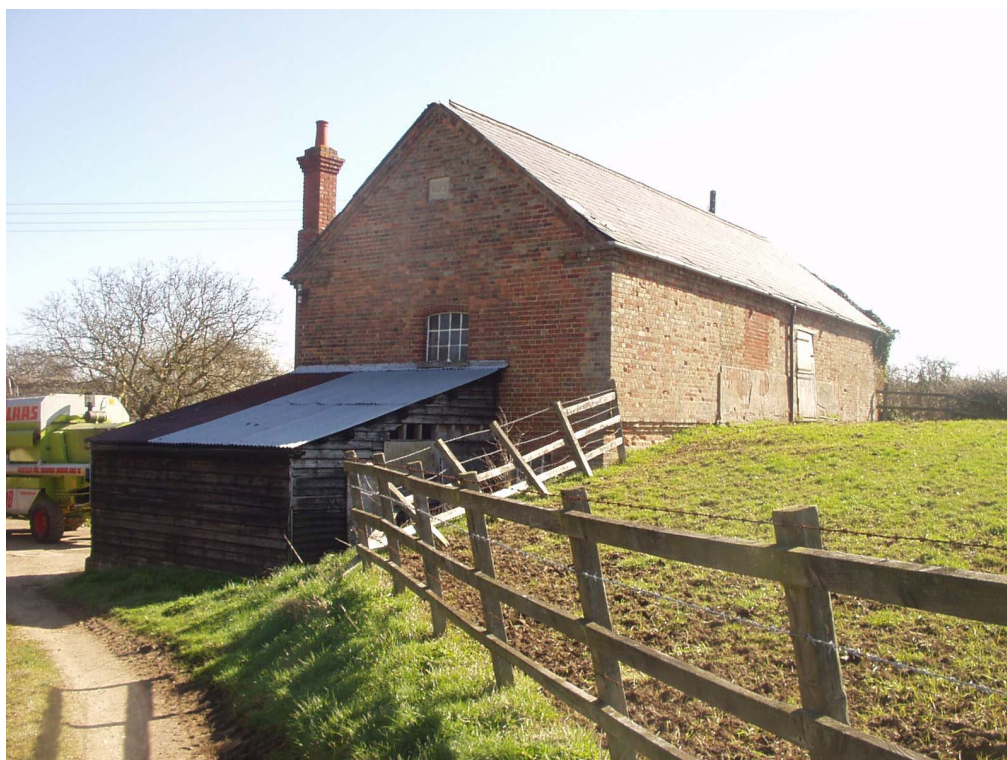
Image 5: Mill building, which was extended in the 1873 according to stone date tablet, with later ramp (D) to first floor associated with change in use.
