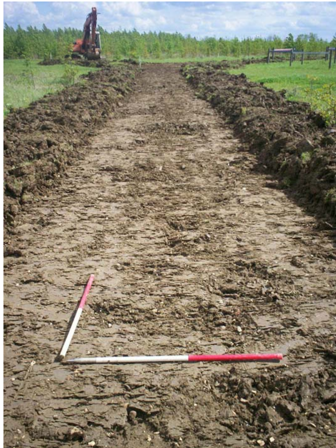
Photograph of road following removal of topsoil, looking east. 1m scales
