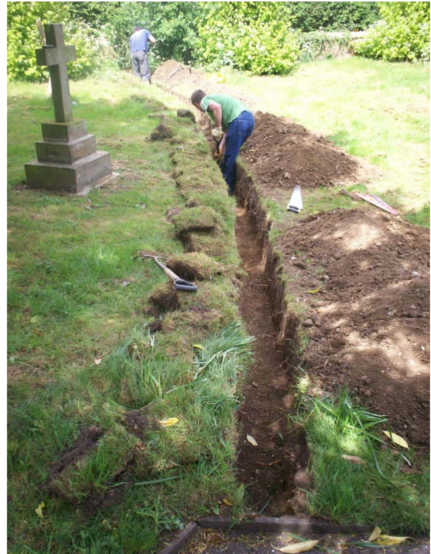
Figure 2: Excavation of the service trench
