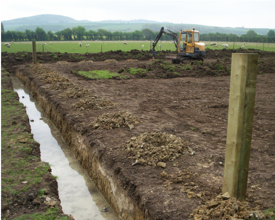
Figure 3: Soakaway trench and topsoil stripping for ménage
