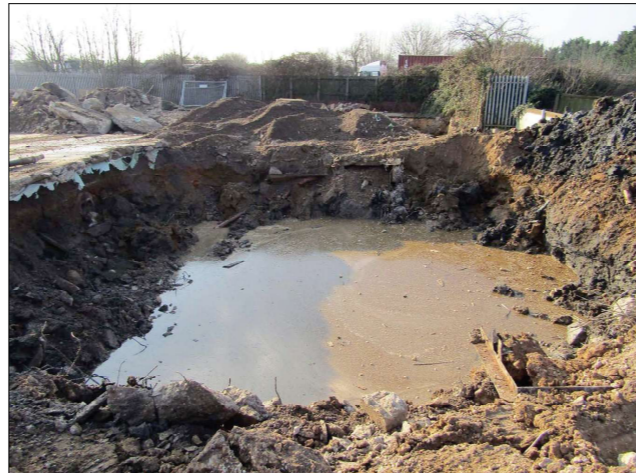
Photograph 5: Removal of tanks (area H)
