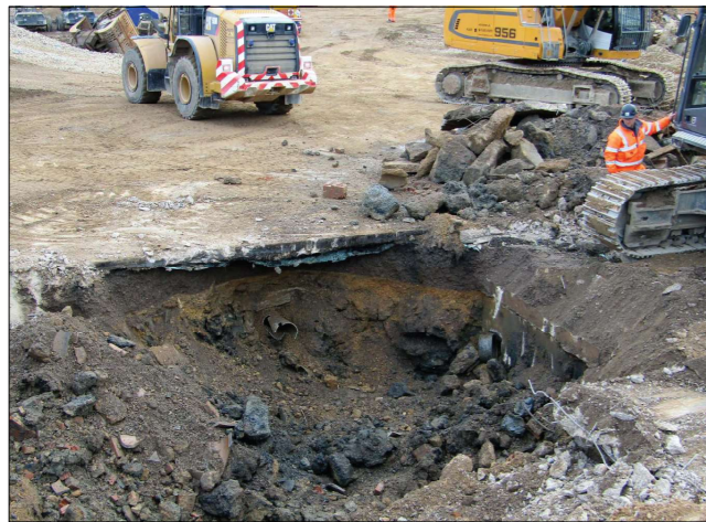
Photograph 4: Removal of tanks (area H)
