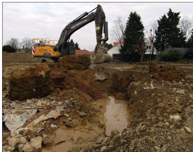
Photograph 7: Removal of concrete pads (area B)
