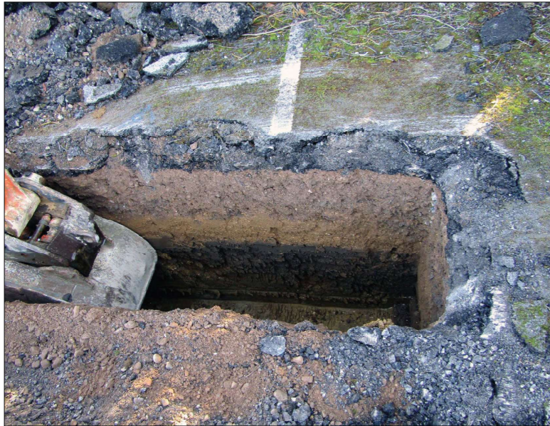
Photograph 1: TP1, looking east
