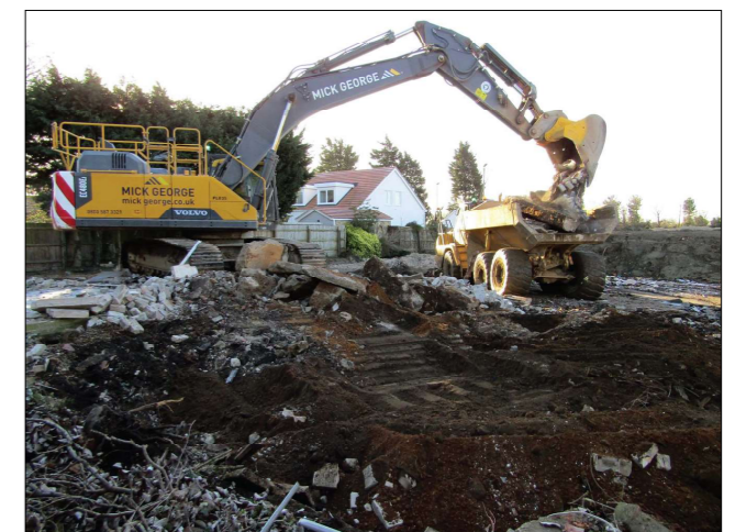
Photograph 9: Removal of building footings (area D)
