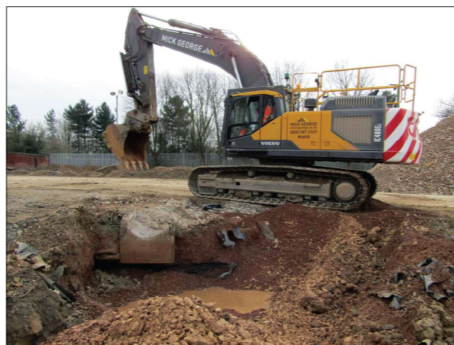
Photograph 8: Removal of drains (area B)
