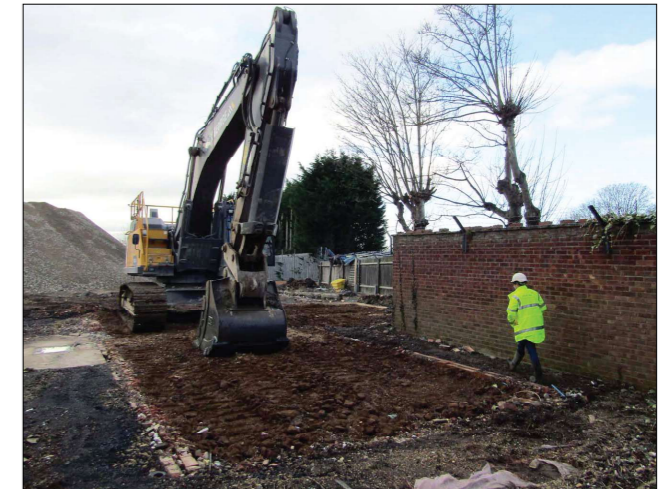
Photograph 6: Removal of building footings (area G)
