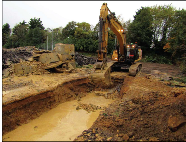
Photograph 1: Removal of drainage tanks (area A)
