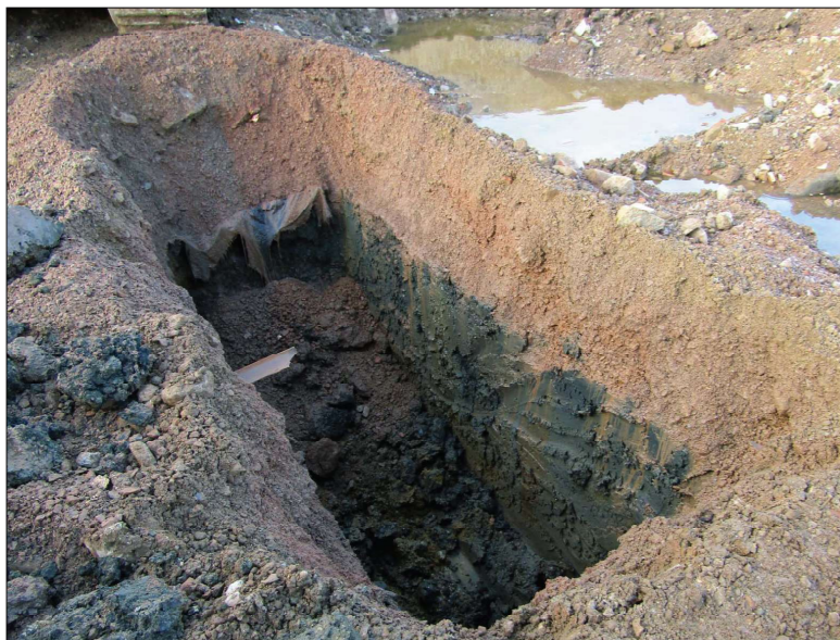
Photograph 4: TP32, looking north-east
