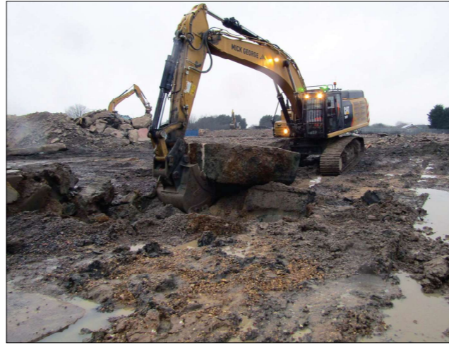
Photograph 2: Removal of concrete pads (area C)
