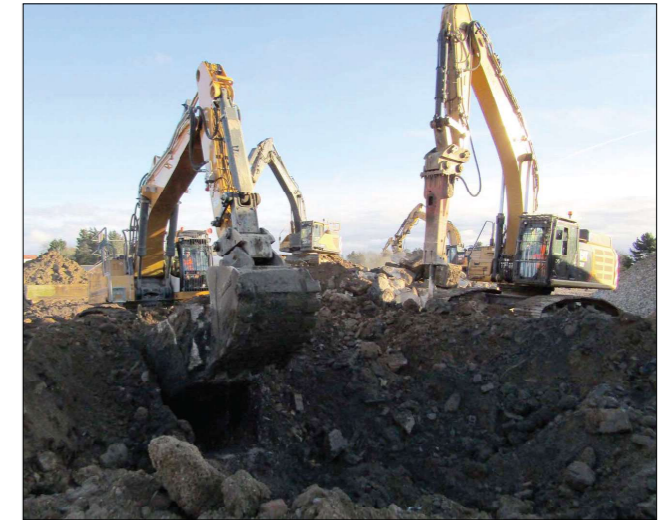
Photograph 3: Removal of concrete pads (area E)
