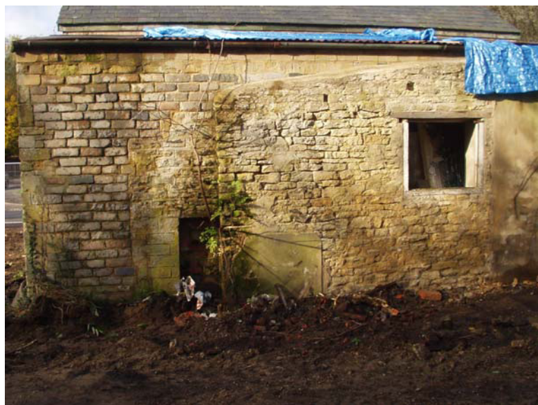
Photograph 1: Eastern elevation of northern outbuilding, showing incorporation of earlier limestone building.
