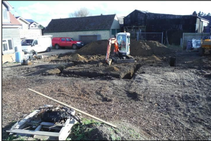
Plate 5: General view, looking south
