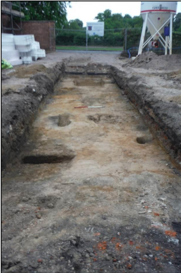
Trench 1 – looking east (1m scale)
