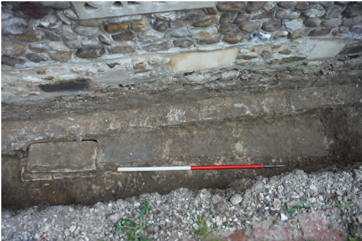
Plate 2: Trench 2 – burial vault (204) with stone capping (205) (1m scale)
