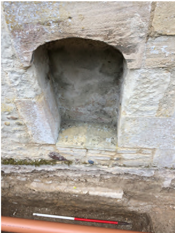
Plate 13: Trench 6 – side view of remnant of clunch stone floor (613) of demolished chapel (20cm scale)
