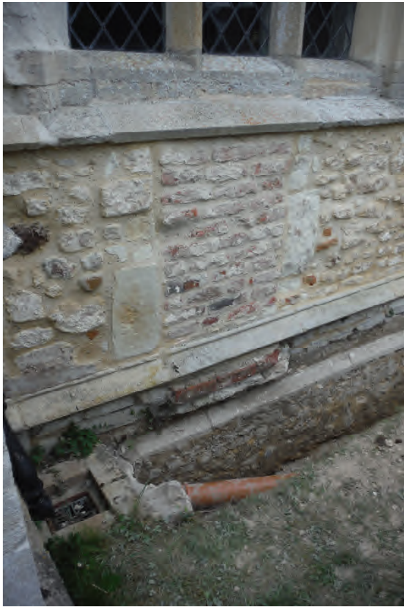
Plate 1: Trench 1 – chancel foundation (102) and bricked-up opening
