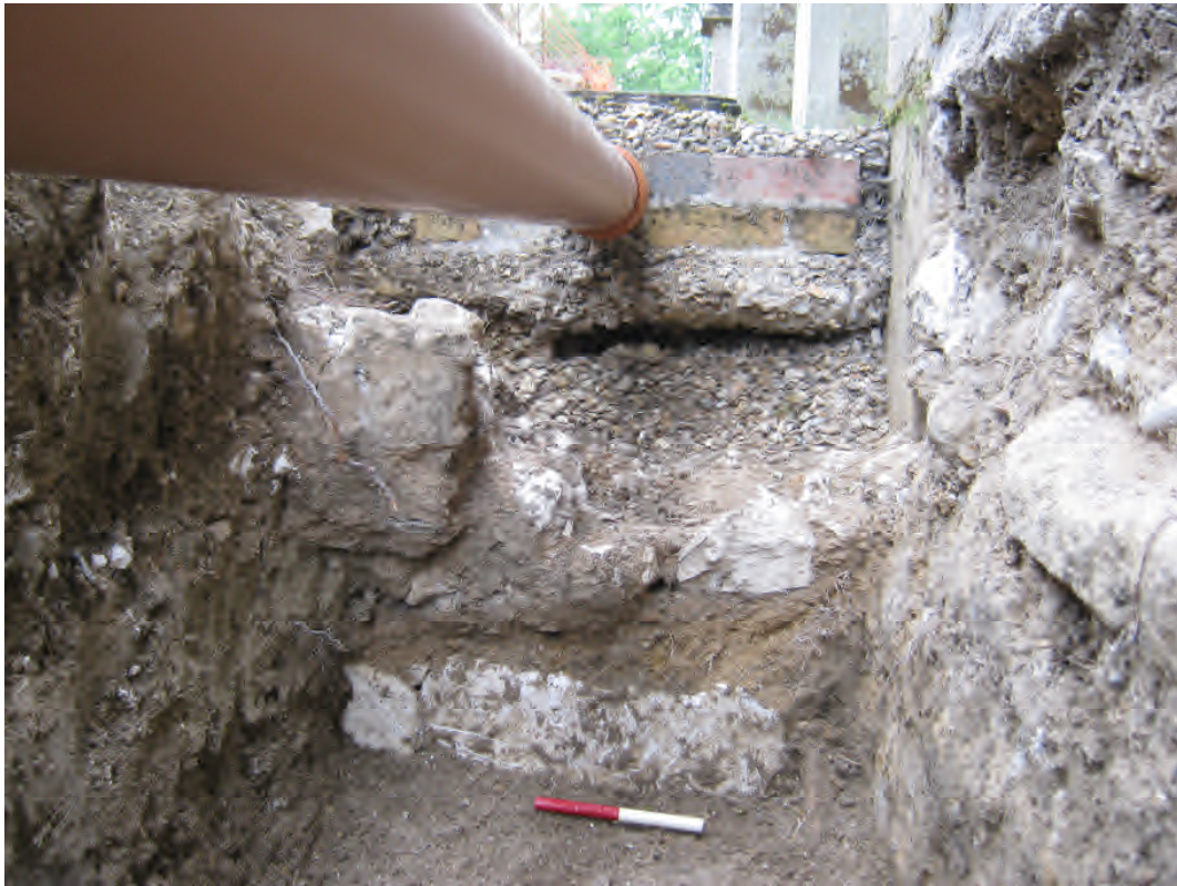
Plate 11: Trench 6 – side view of eastern arm of demolished chapel foundations (611) (20cm scale)
