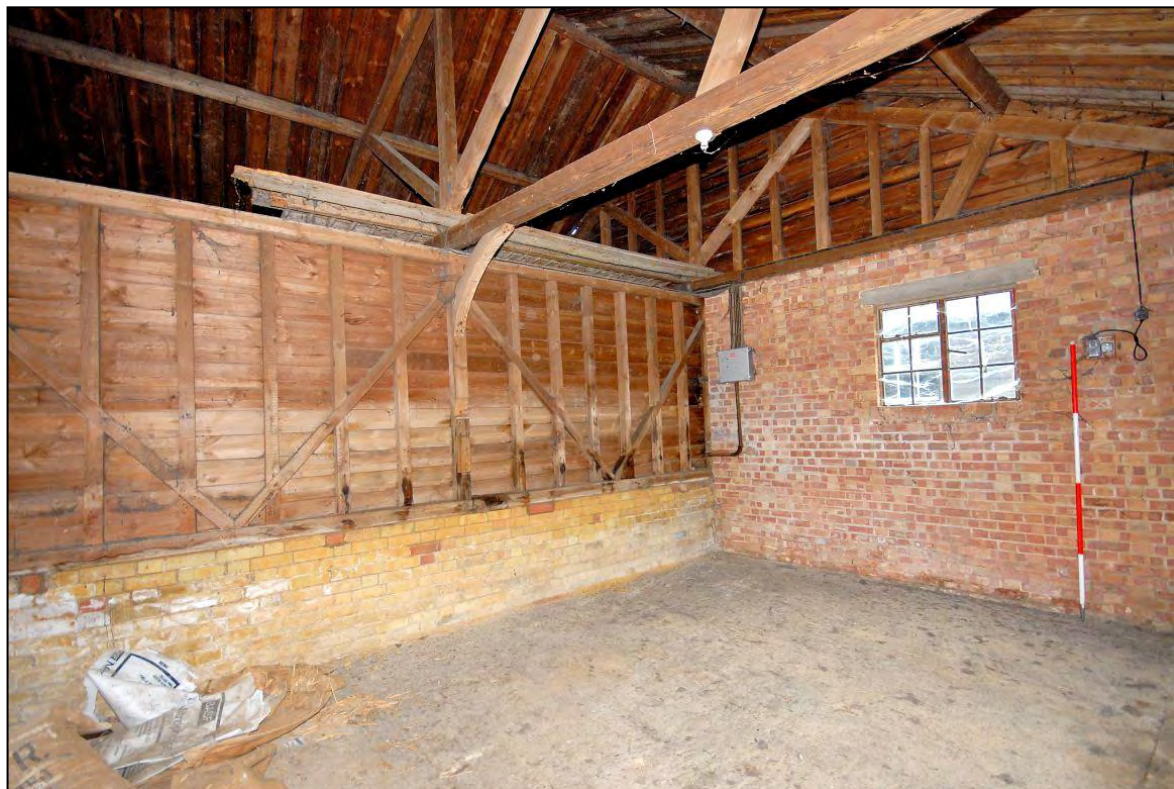
Image 26: Shelter sheds, north shed, looking south-west
