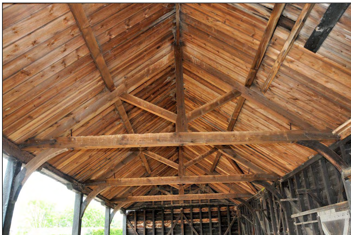
Image 20: Cart shed, looking south, roof
