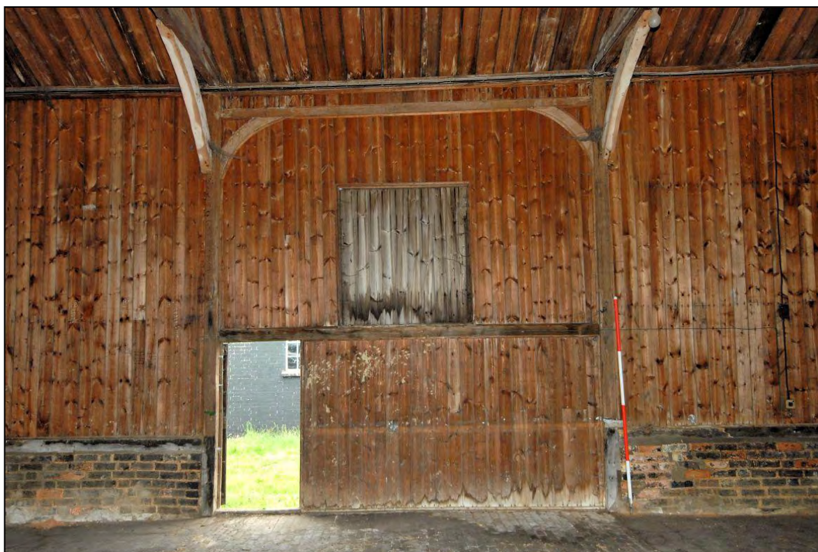
Image 6: Barn, central bay in north wall
