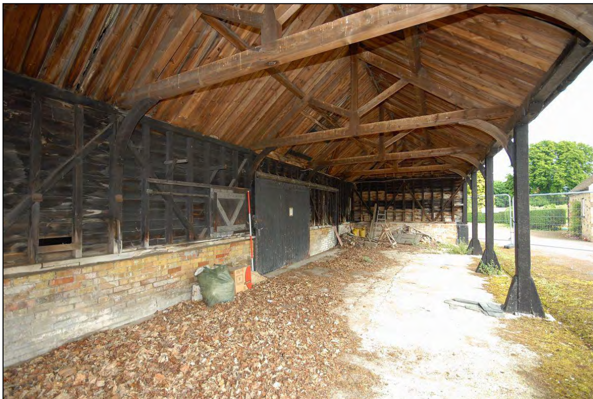
Image 19: Cart shed, looking north
