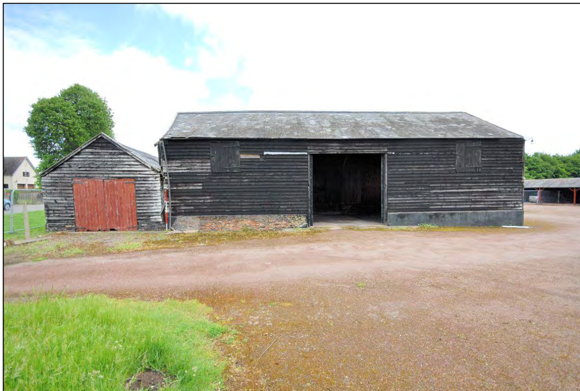
Image 3: Barn, south elevation
