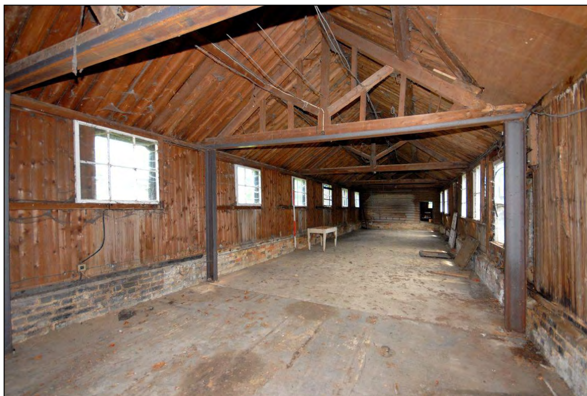
Image 12: West range, south compartment, looking north
