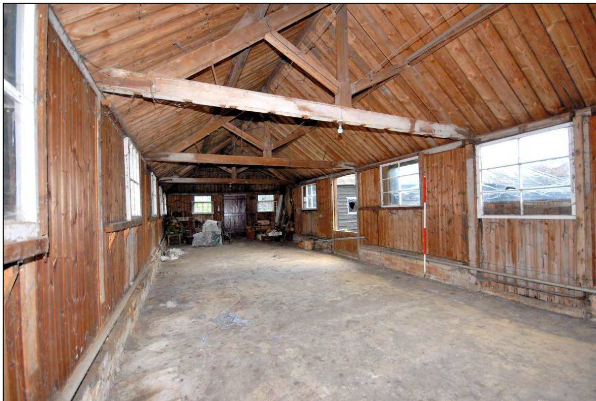
Image 15: West range, north compartment, looking north
