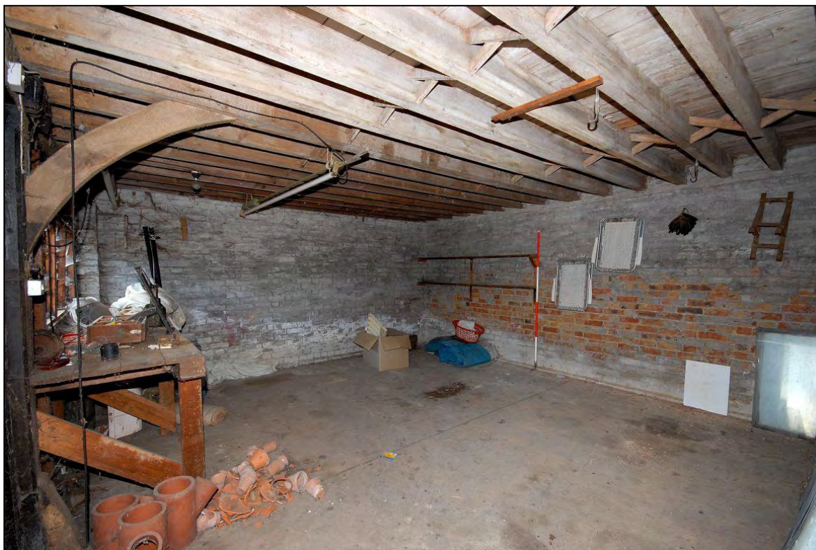
Image 29: Garage, north compartment, looking north-east
