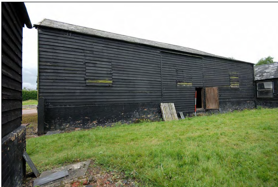
Image 4: Barn, north elevation
