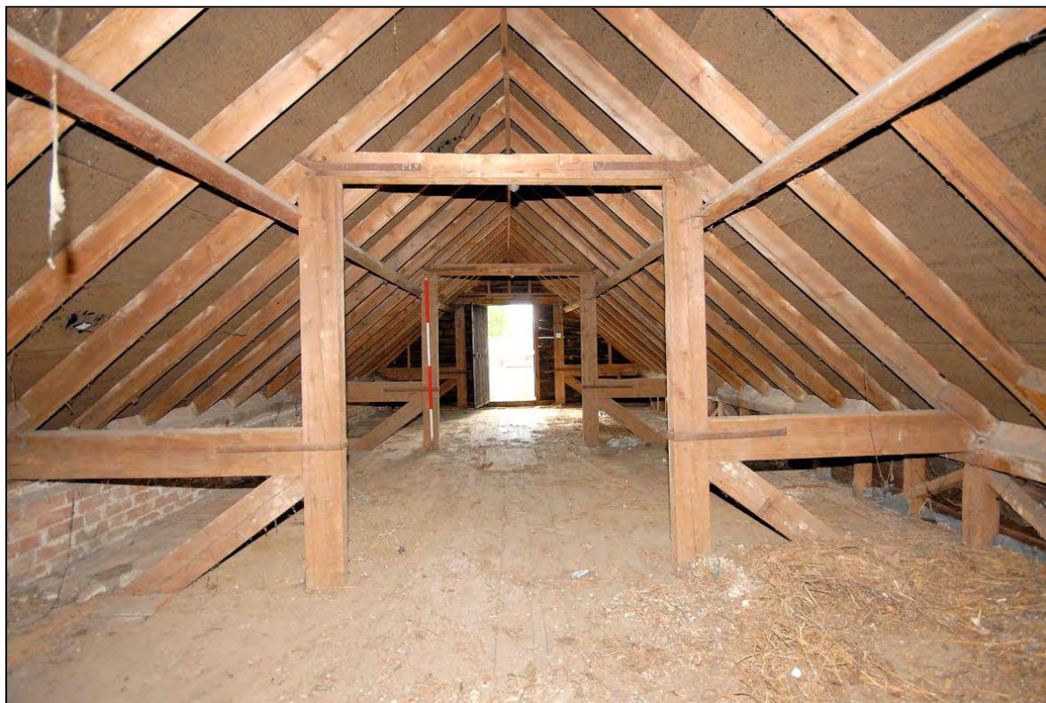
Image 30: Loft above garage, looking south
