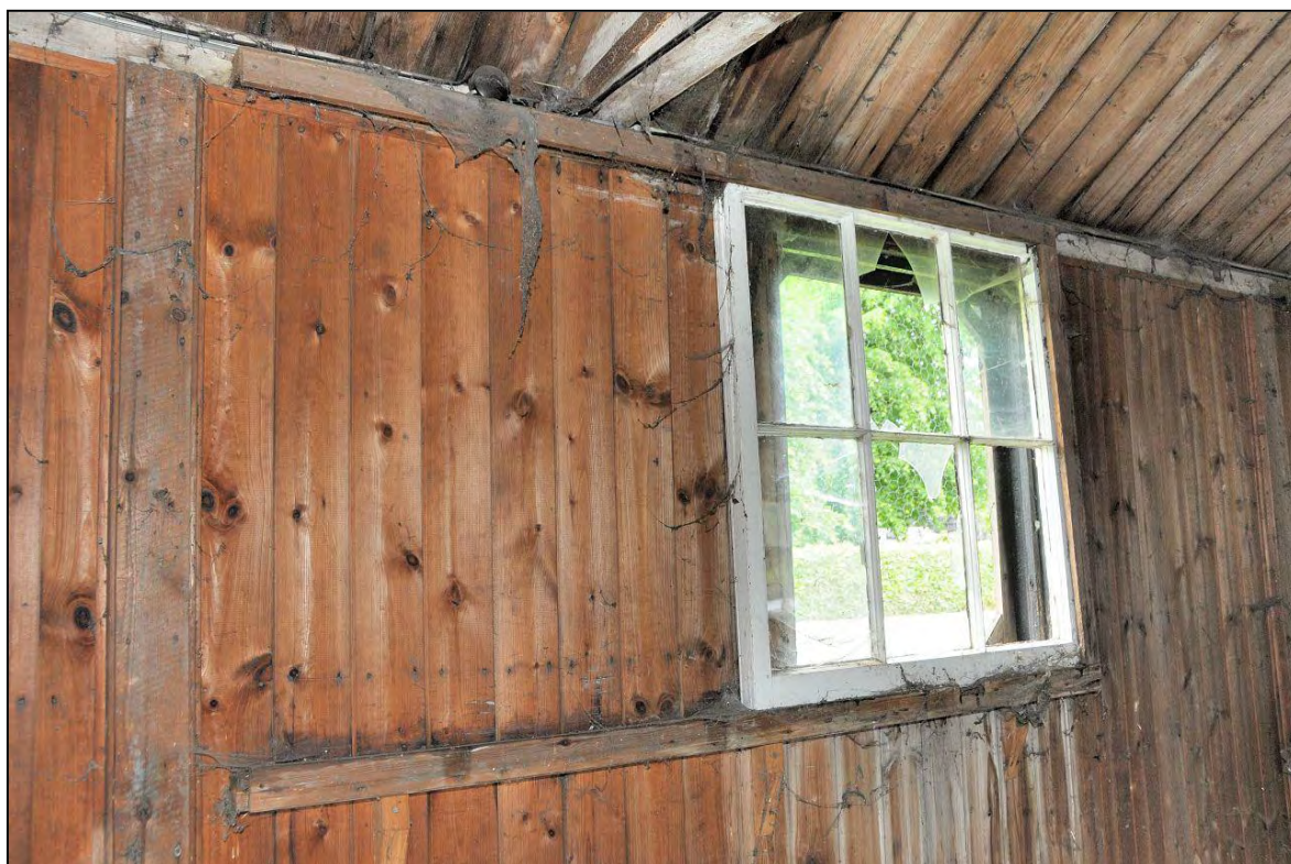
Image 17: West range, detail of sliding window in west wall
