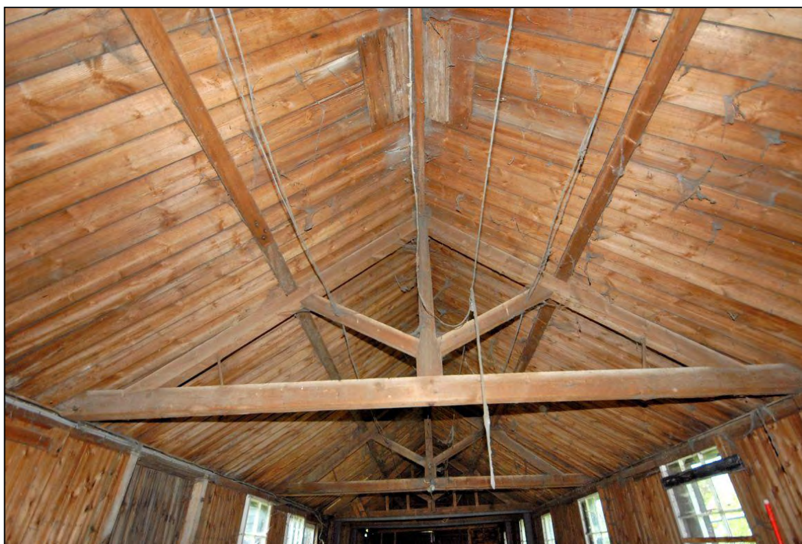
Image 14: West range, south compartment, roof Shows fourth truss from south end
