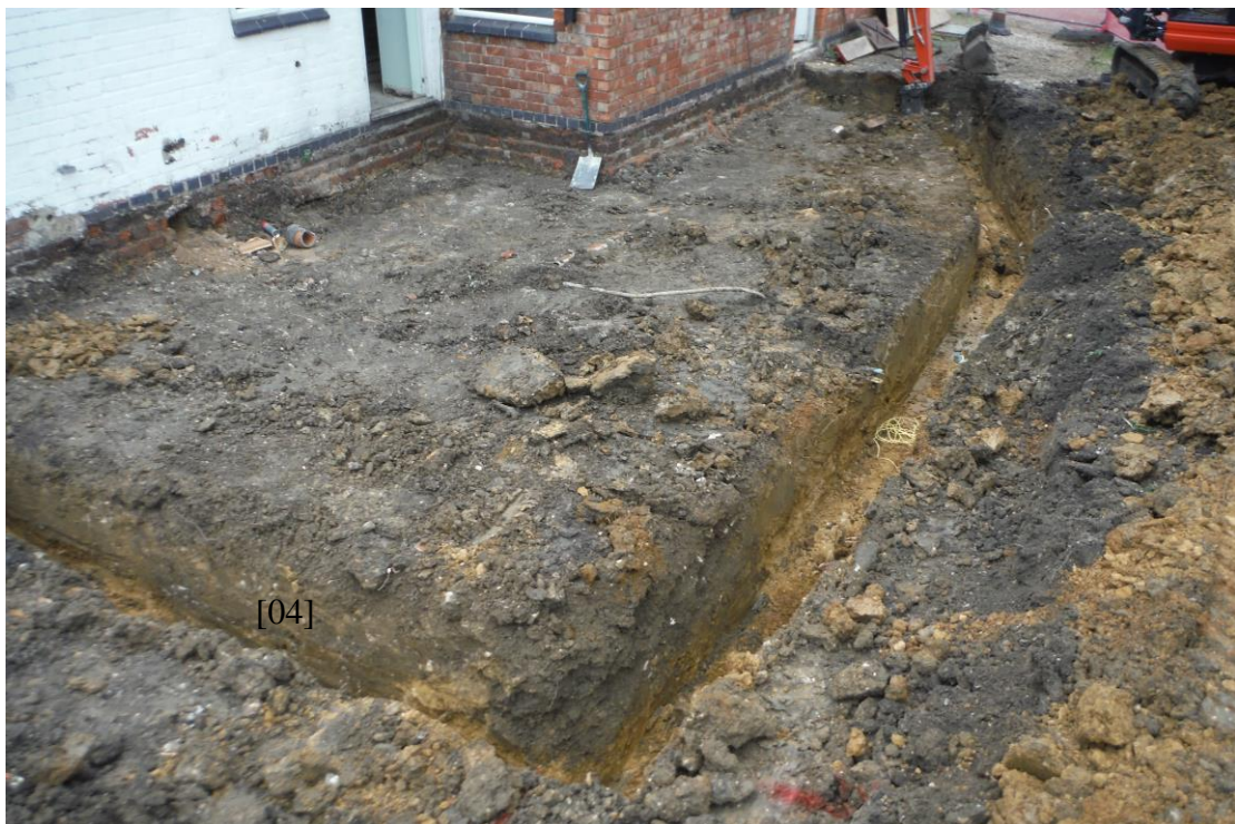
Image 2: General view of area looking from the SE, after the footing trenches had been excavated to formation level. Pit [04] is visible in the foreground (labelled).
