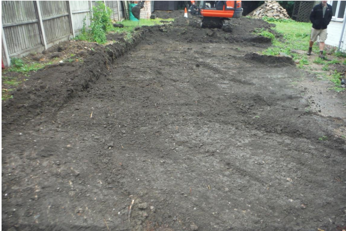
Image 1: General view of area looking northwards, during initial strip of topsoil (01)
