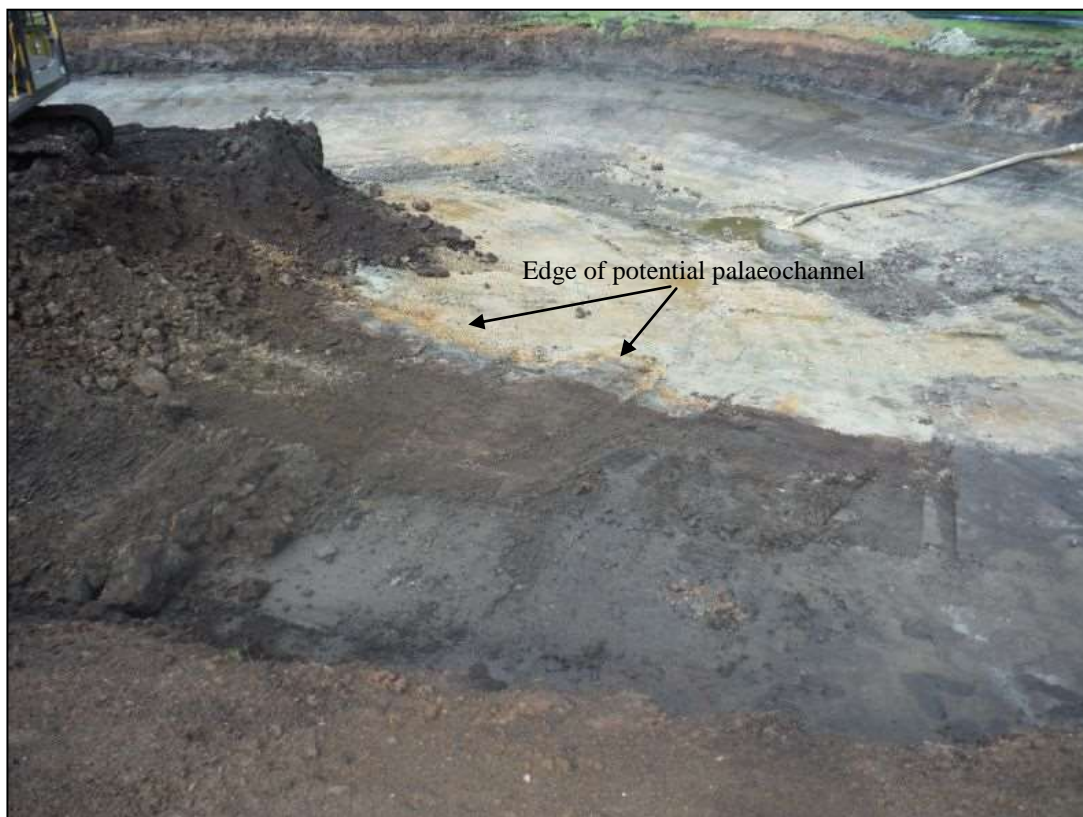
Plate 8: Edge of the potential palaeochannel, looking north
