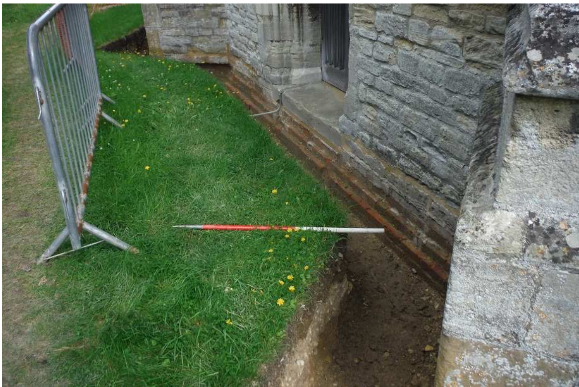
Plate 15: Trench 5 – west-facing tower foundation (504) (1m scale)
