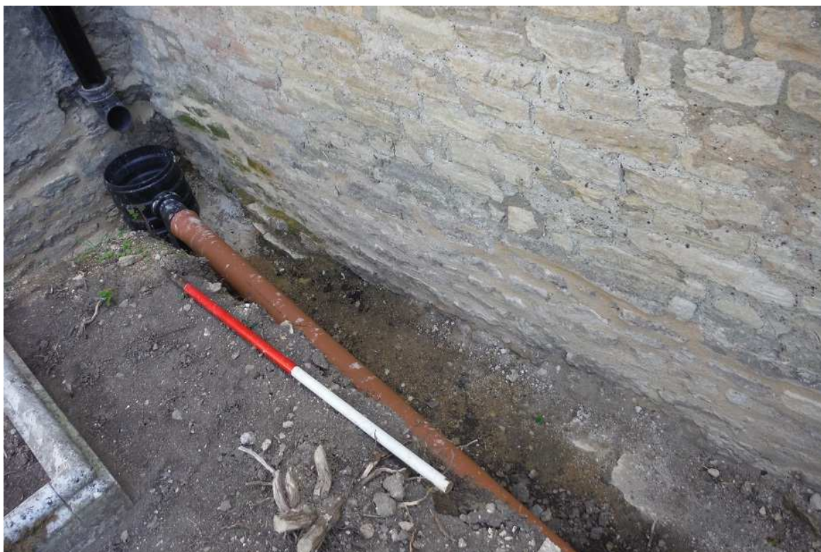
Plate 1: Trench 1 – south porch, west-facing foundation (104) (1m scale)
