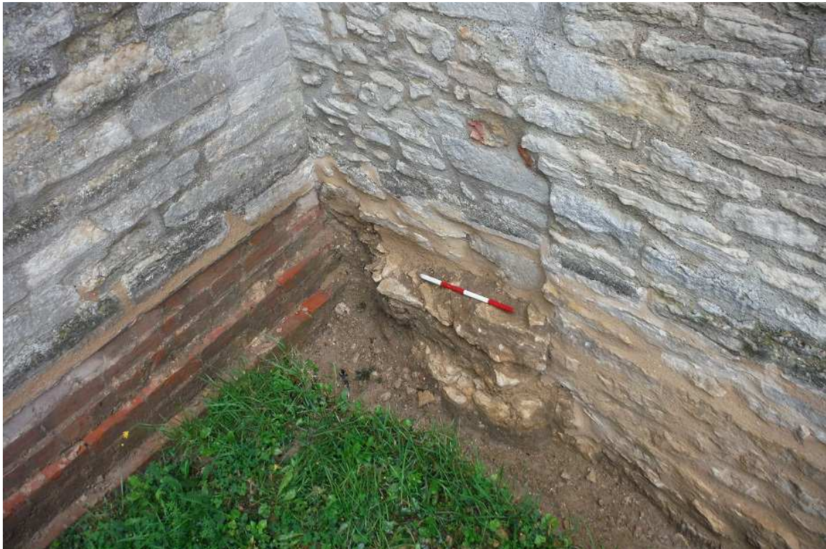
Plate 6: Trench 2 – south aisle, nave foundation remnant (207) (40cm scale)
