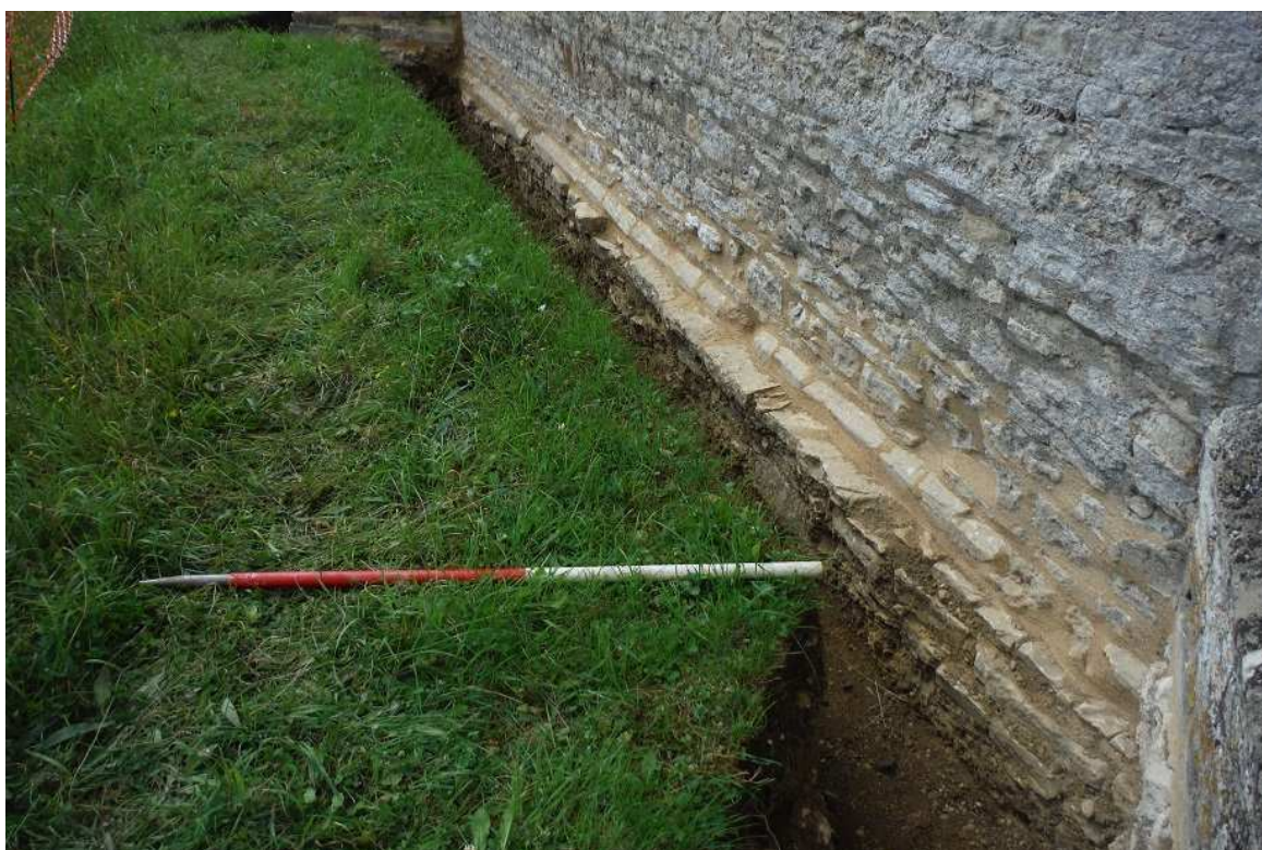
Plate 9: Trench 3 – east-facing chancel foundation (304) (1m scale)
