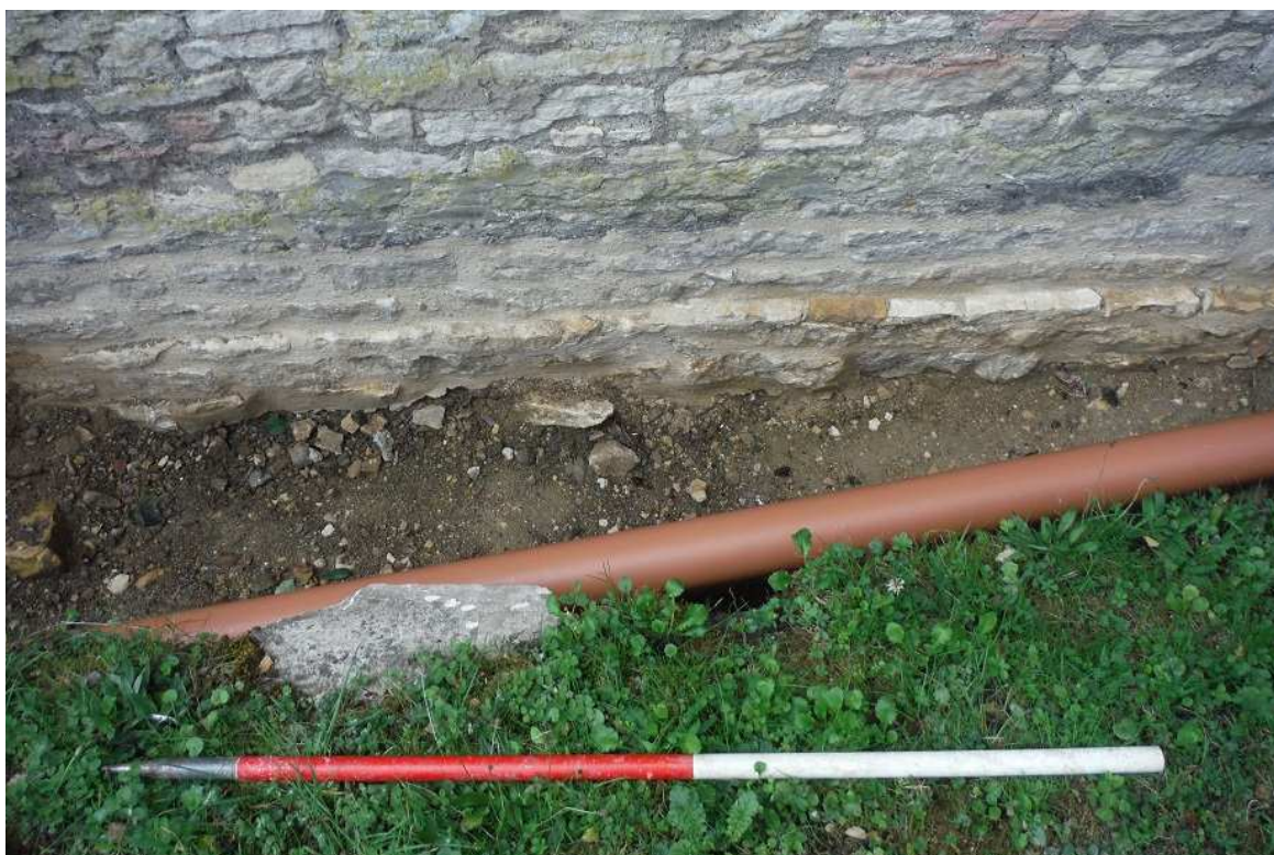
Plate 2: Trench 1 – south porch, west-facing foundation (104) (1m scale)
