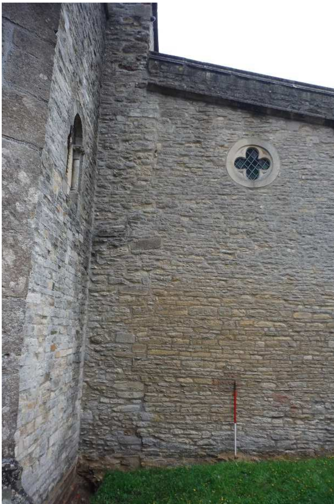
Plate 7: Trench 2 – south aisle with surviving nave wall segment (scale 1m)
