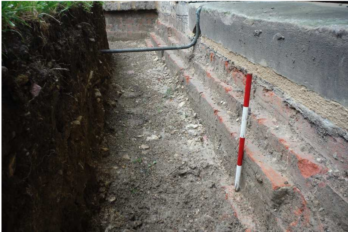
Plate 16: Trench 5 – close-up of west-facing tower foundation (504) (40cm scale)
