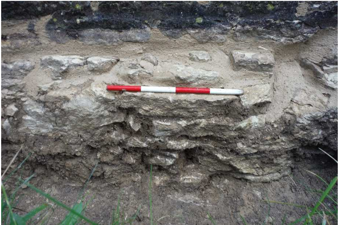
Plate 13: Trench 4 – close-up of north-facing north aisle foundation (405) (40cm scale)
