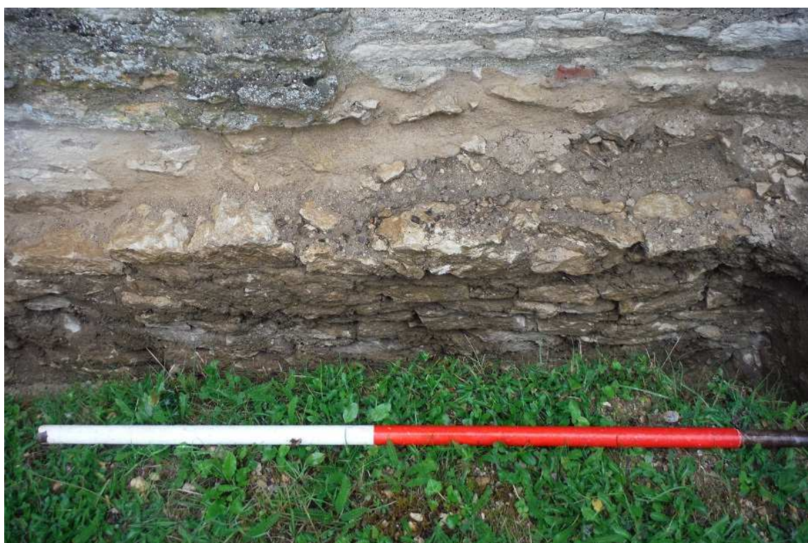
Plate 4: Trench 2 – south aisle, south-facing foundation (204), further to the east (1m scale)
