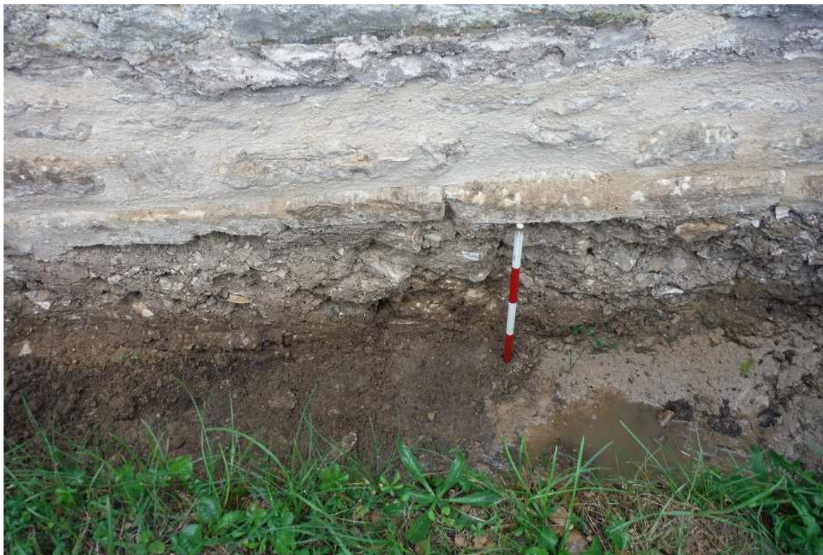
Plate 8: Trench 3 – south-facing chancel foundation (304) (40cm scale)
