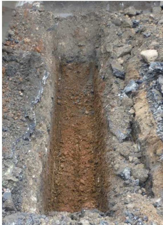
Image 8: Geotechnical Trench 4, looking NE
