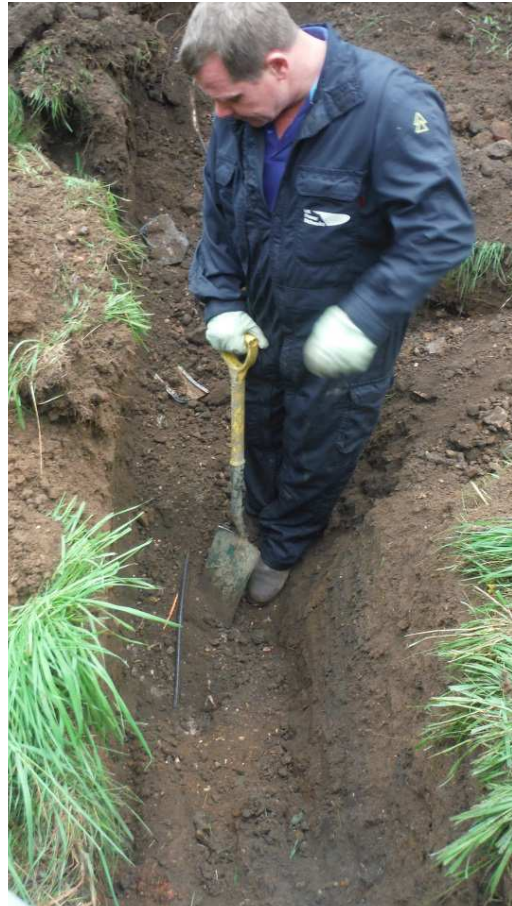
Image 6: Geotechnical Trench 3, looking SE
