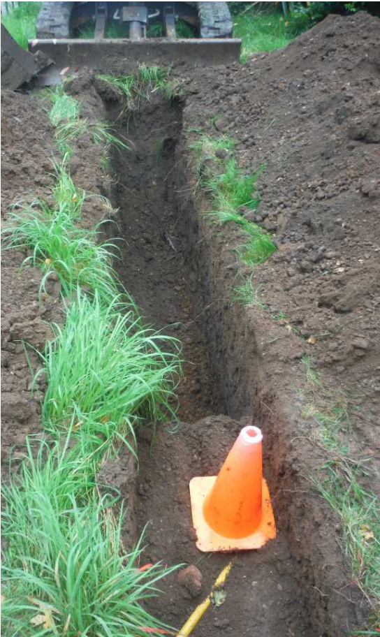
Image 5: Geotechnical Trench 3, looking east
