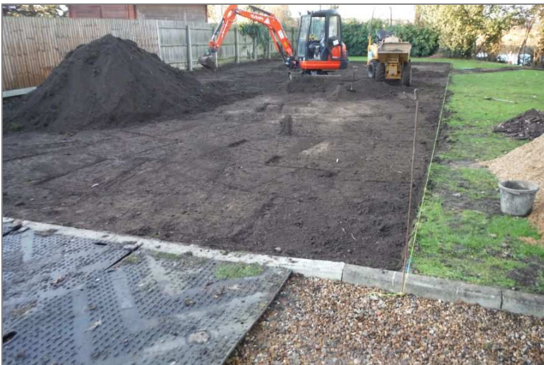
Plate 2: Site strip in progress, looking north-west from the existing car park
