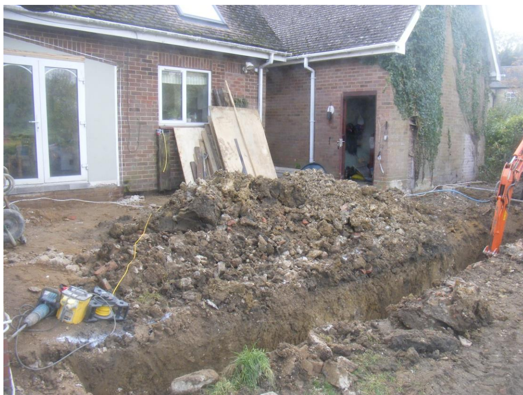
Image 3: General view of northern extension, with footing trench under excavation
