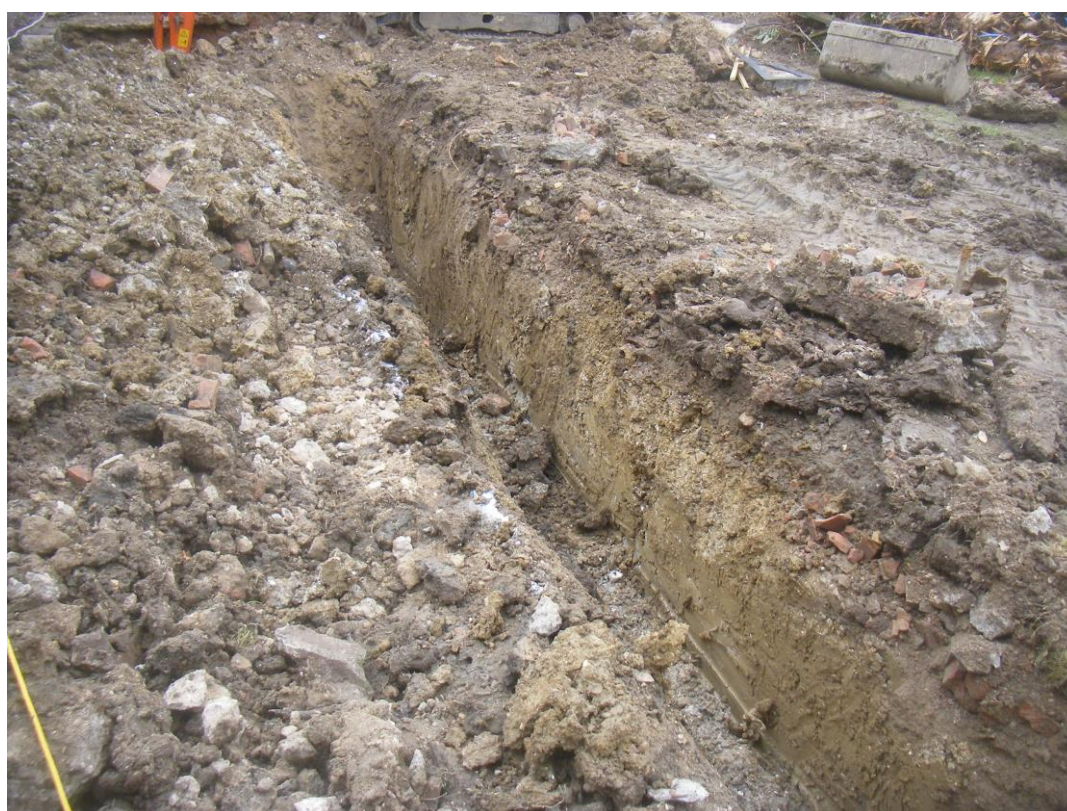
Image 4: General view of section of footing trench, showing truncated soil profile
