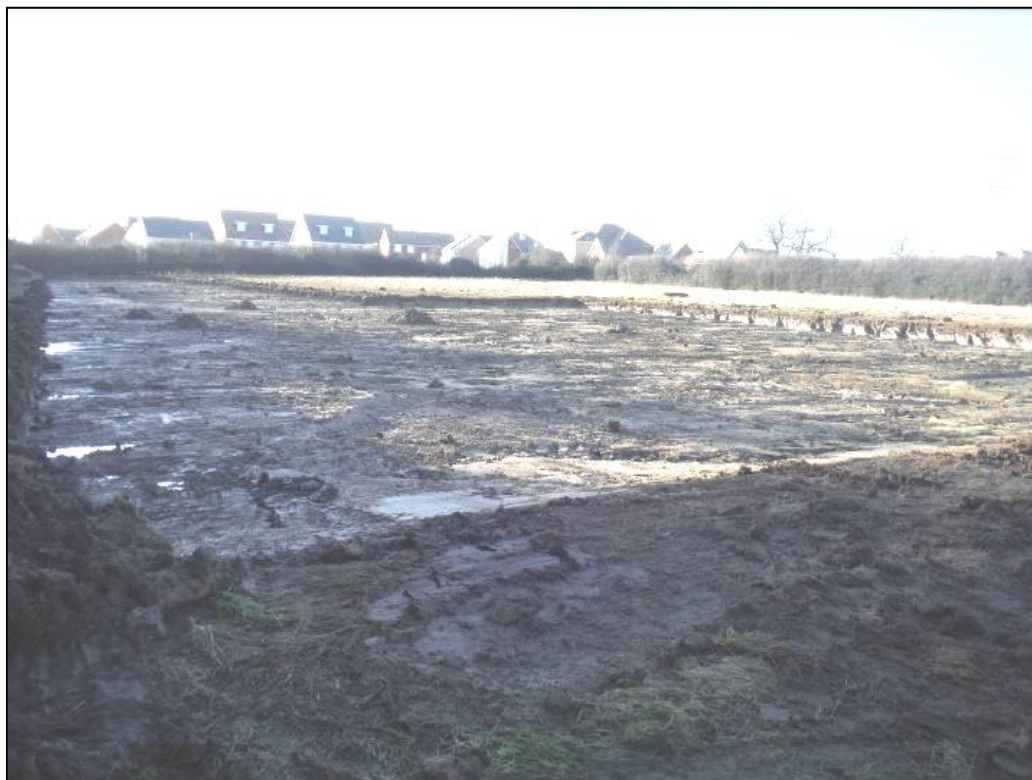
Plate 6: View of the excavation area from the east corner (looking south-west)
