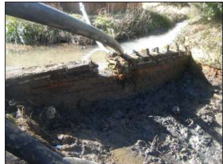
Plate 6: Bath House pond weir, looking west
