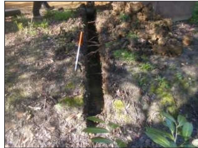
Plate 24: Drainage pipe trench within the Graeco-Roman Alters round, looking south west
