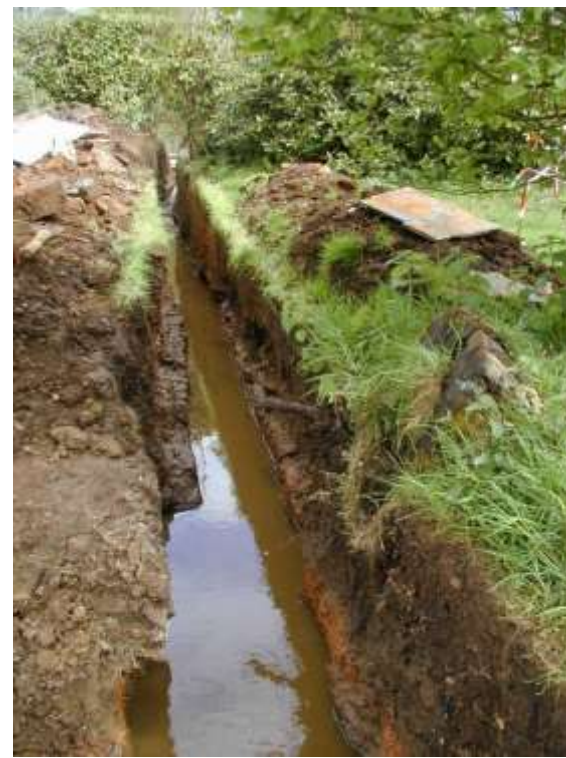
Drain revealed in 2003, looking towards path and orangery
