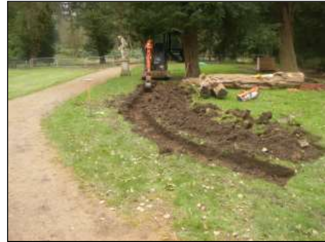
Plate 23: Excavation of Yew hedge trench, west of Ladies Lake, looking south
