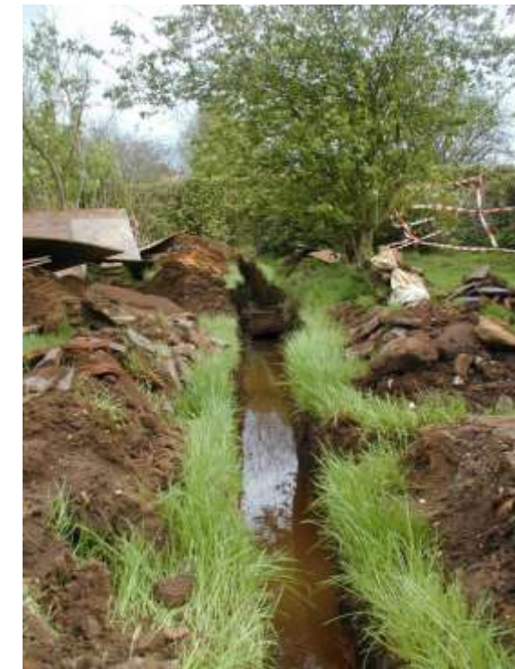
Drain revealed in 2003, looking towards path and orangery
