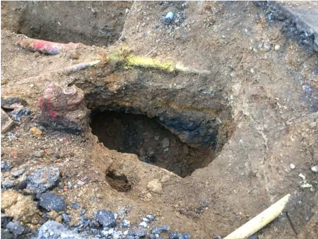
Figure 3: The original excavation, 1st December 2017, looking south
