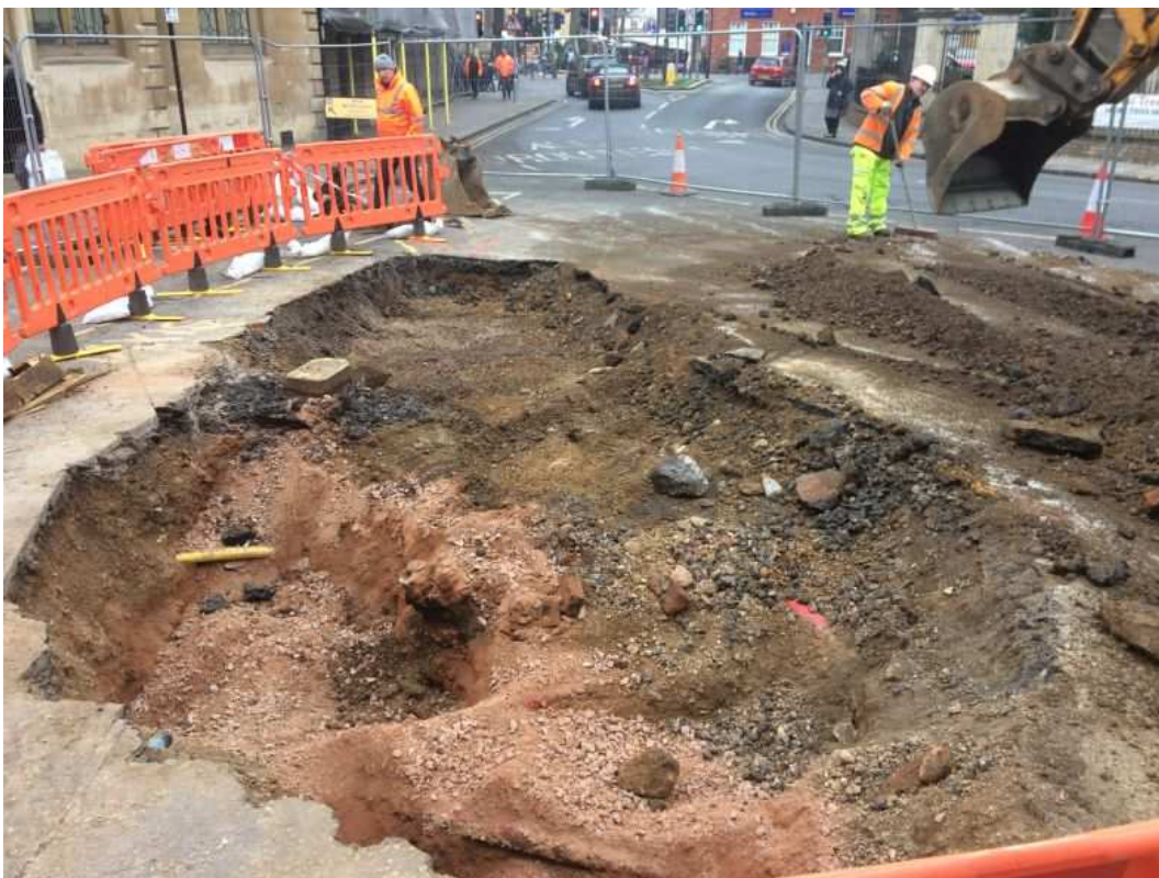
Figure 4: Extended excavation in progress, 6th December 2017, looking north
