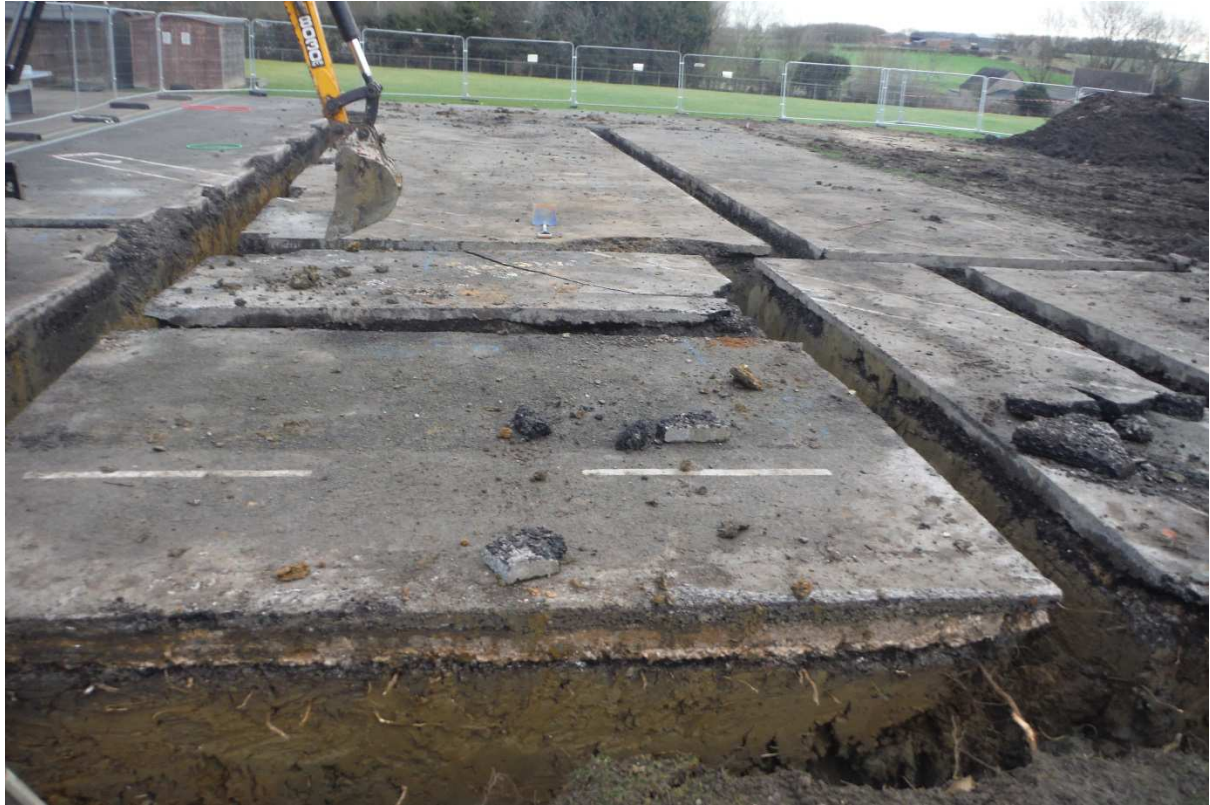
Image 1: General view of footing trenches, looking westwards
