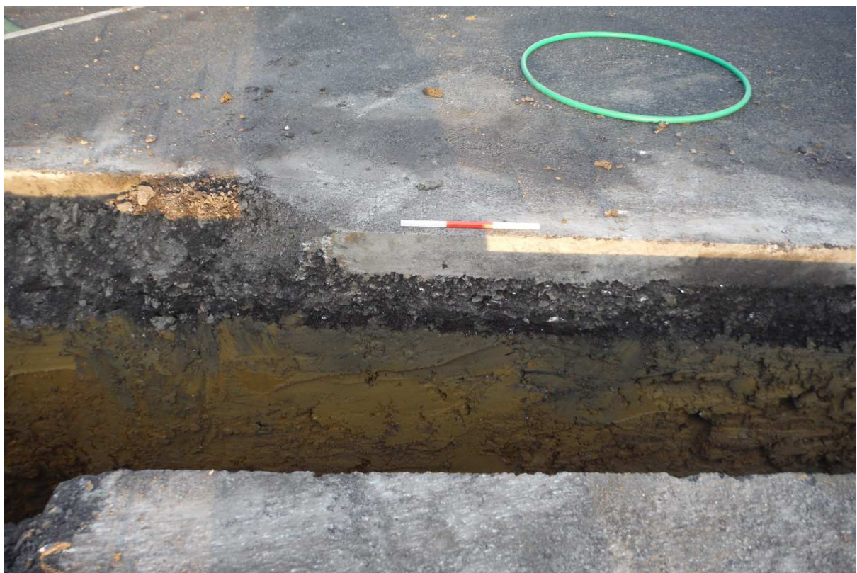
Image 2: Typical soil profile revealed by excavation of the footing trenches, showing areas of darker material incorporating tarmac sub-strata. Scale 30cm in 10cm divisions.
