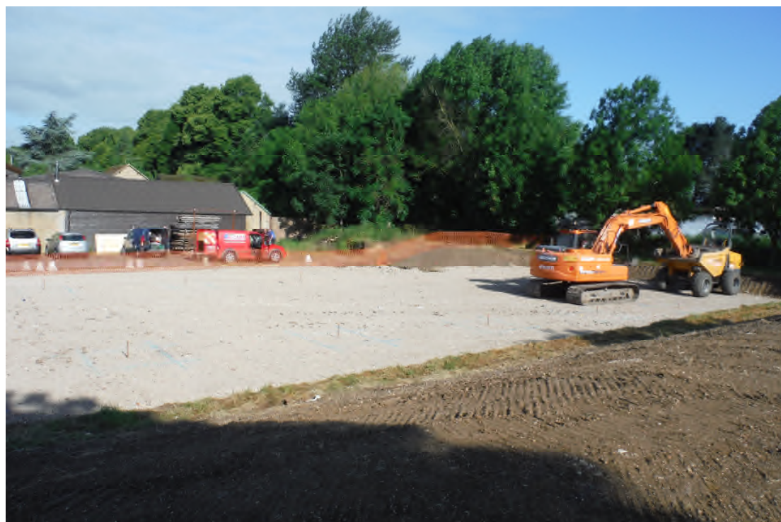
Image 4: Stone spread (8) within the building footprint
