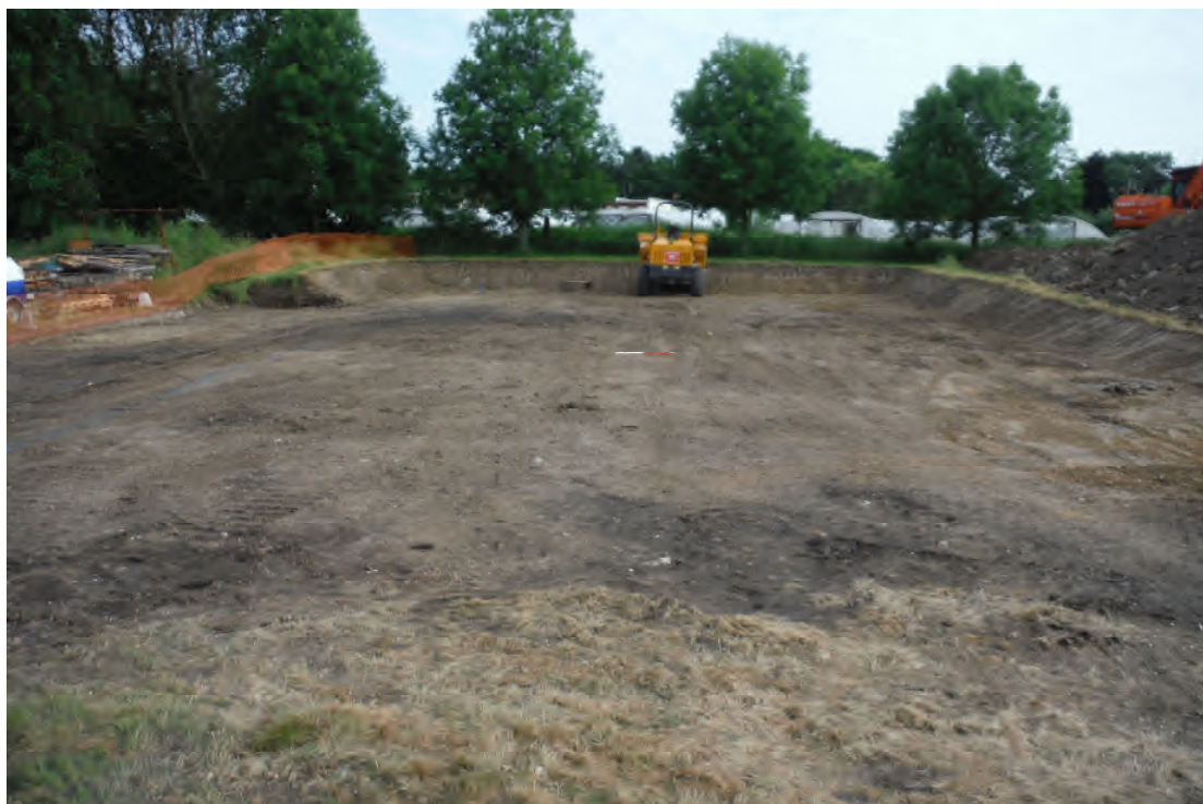
Image 3: General view of the building footprint stripped to the formation level, which is within made-ground deposit (2) (scale 1m in 50cm divisions)
