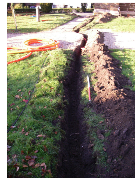
Southern cable trench: looking north
