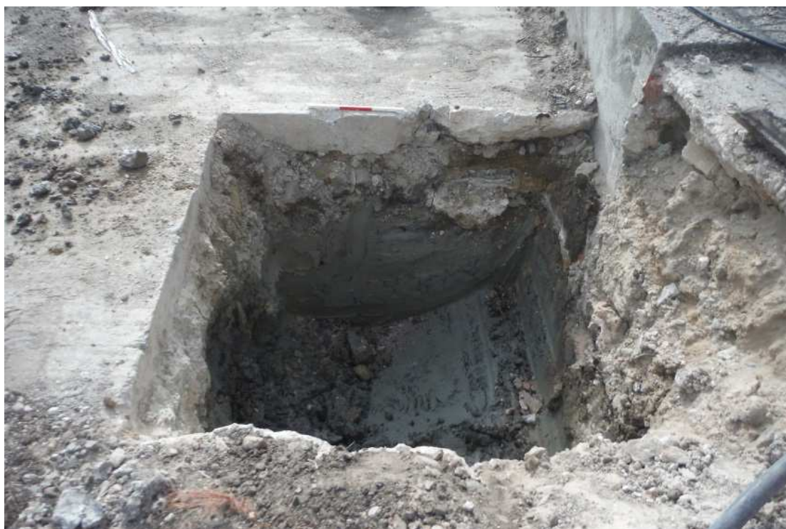
Image 1: Pit 2, looking east (scale 0.3m in 10cm divisions)
