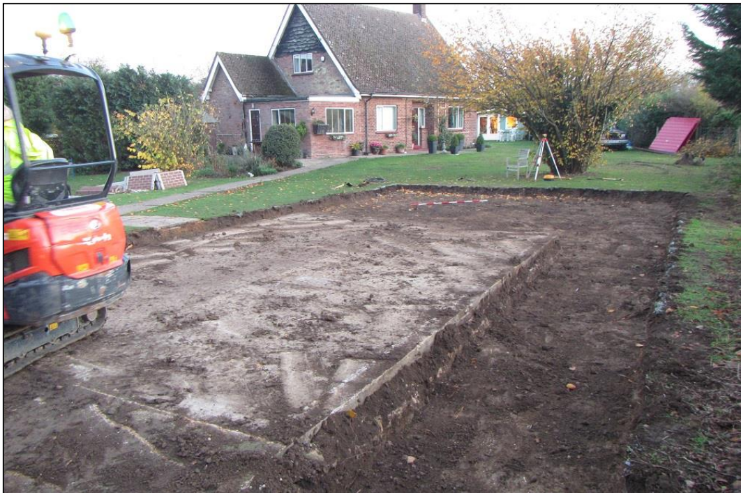
Image 2: View of trench and retained slab, looking south-east (Scale 2m)
