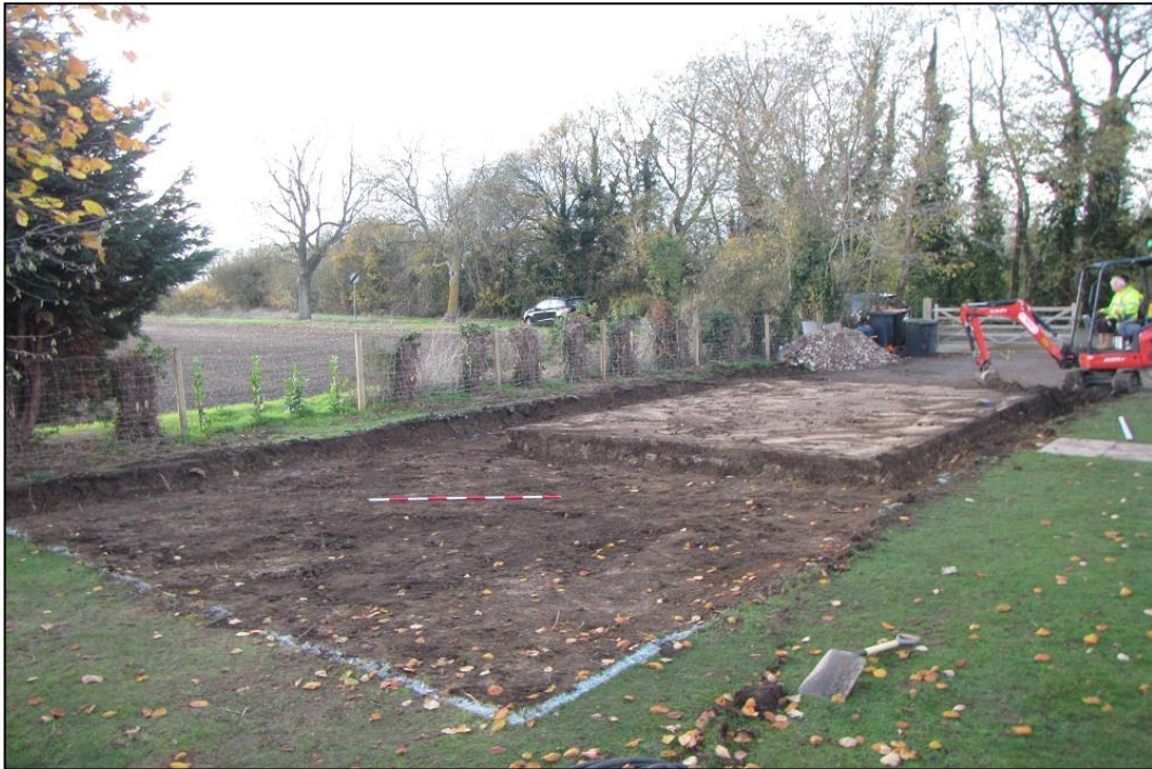
Image 1: View of the trench and retained slab, looking north-west (Scale 2m)
