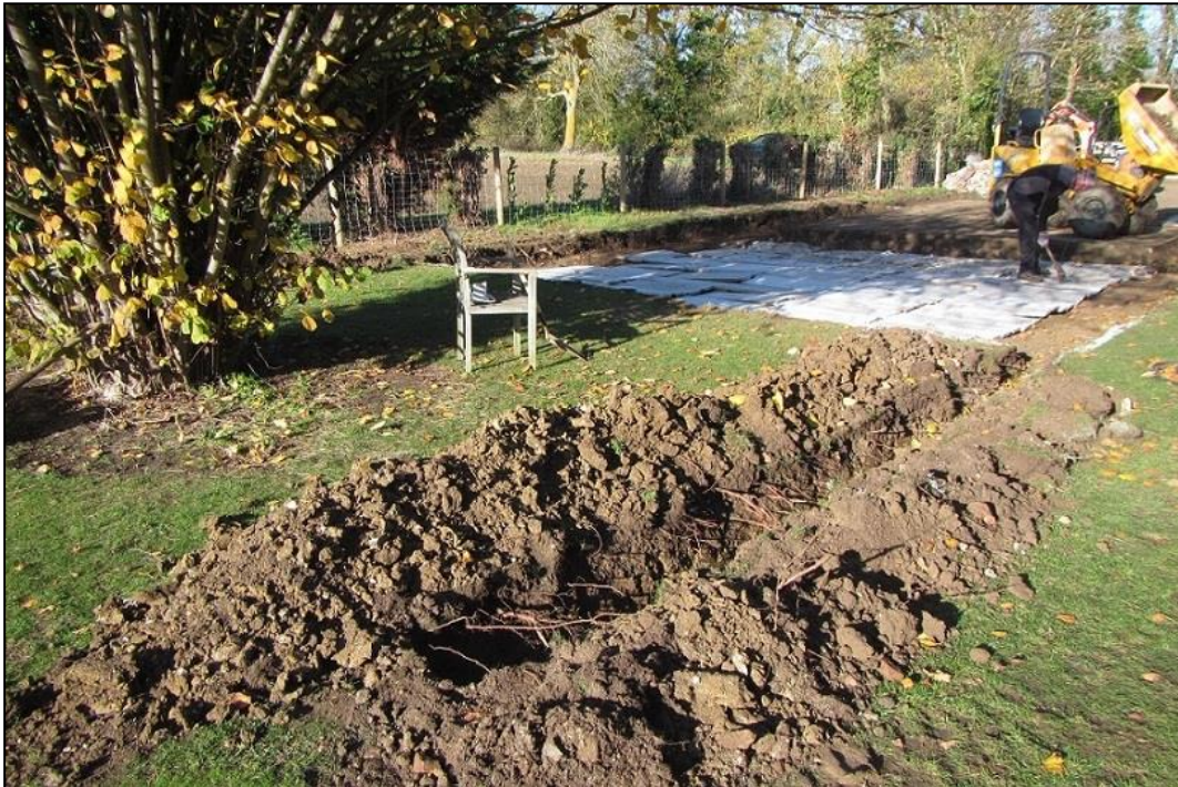
Image 3: Drainage trench extending from south-east corner of foundation, looking north-west
