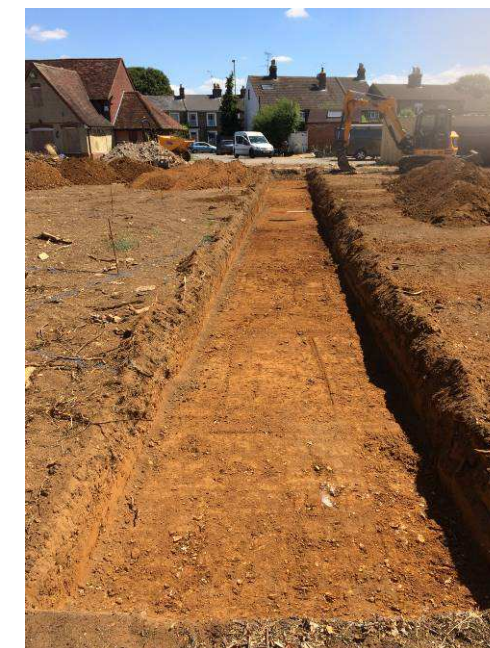
Trench 3 looking SE
