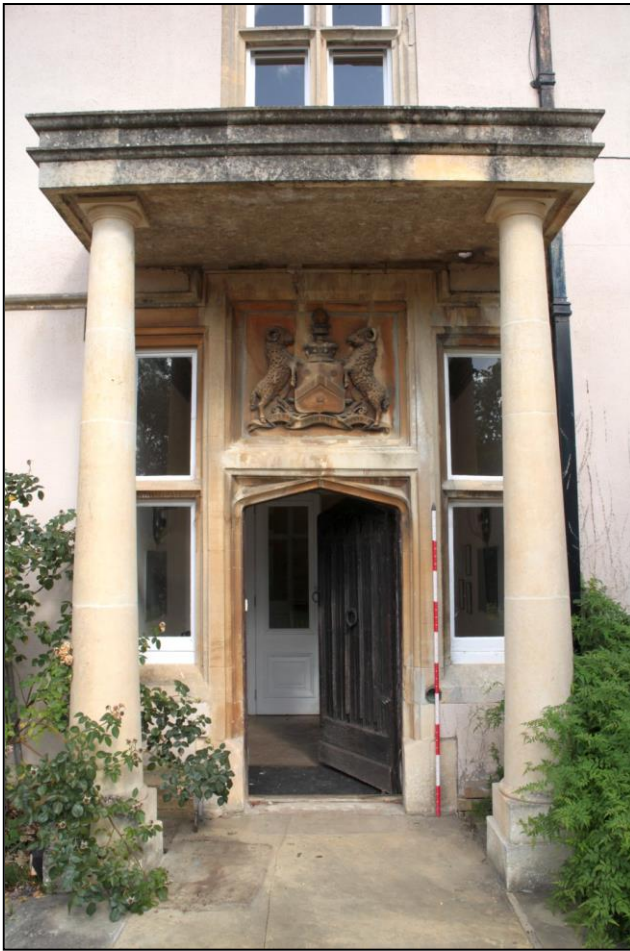
Image 3: South elevation: detail of main entrance
