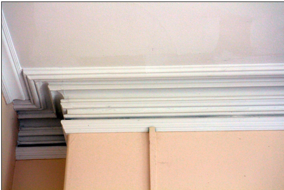
Image 21: Bedroom 18: detail of cornice
