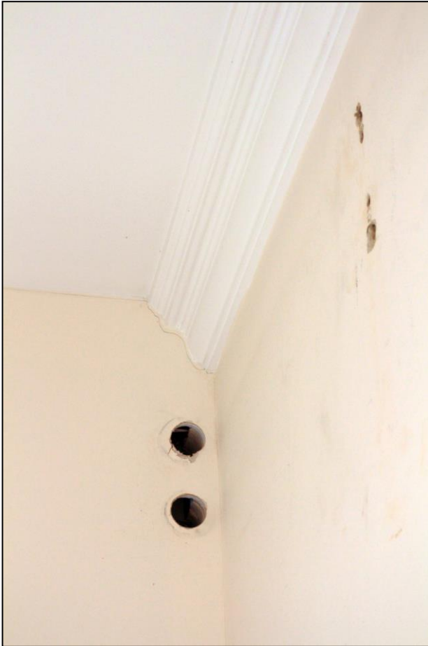
Image 36: Corridor adjacent to rooms 16 and 17
