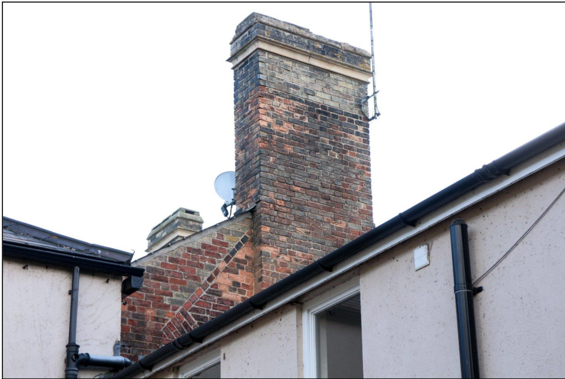
Image 11: Chimney and gable detail
