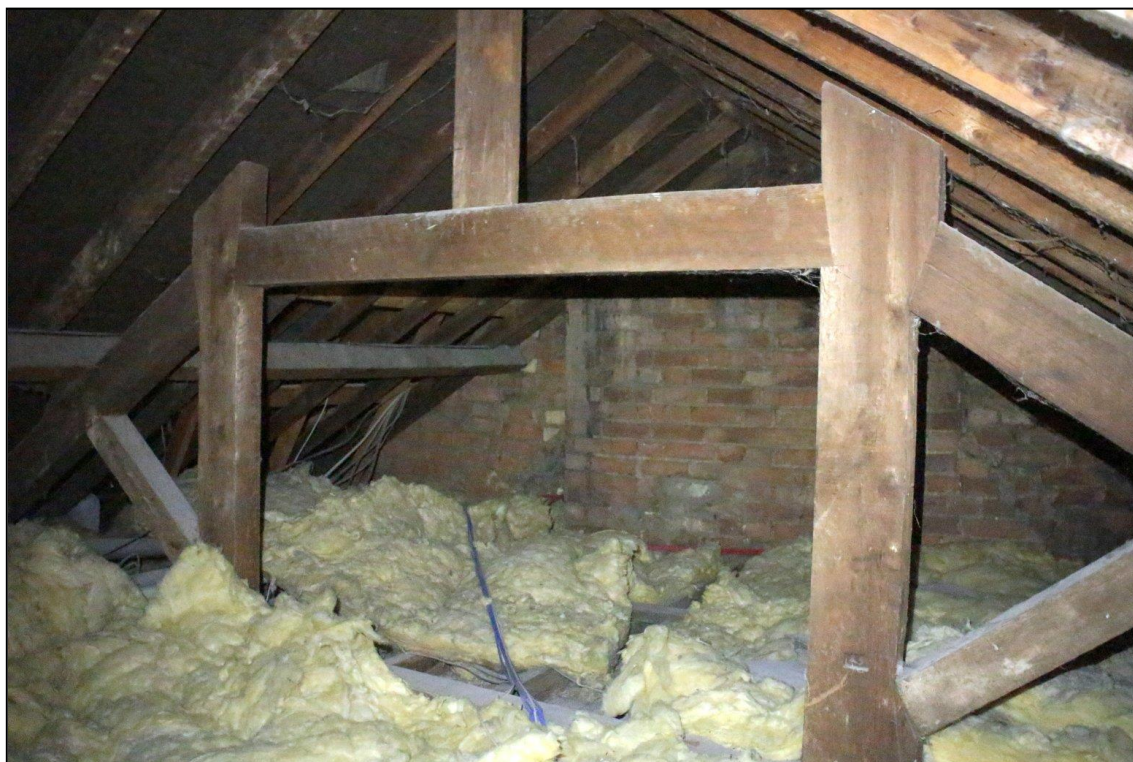
Image 41: Roof space above bedroom 26
