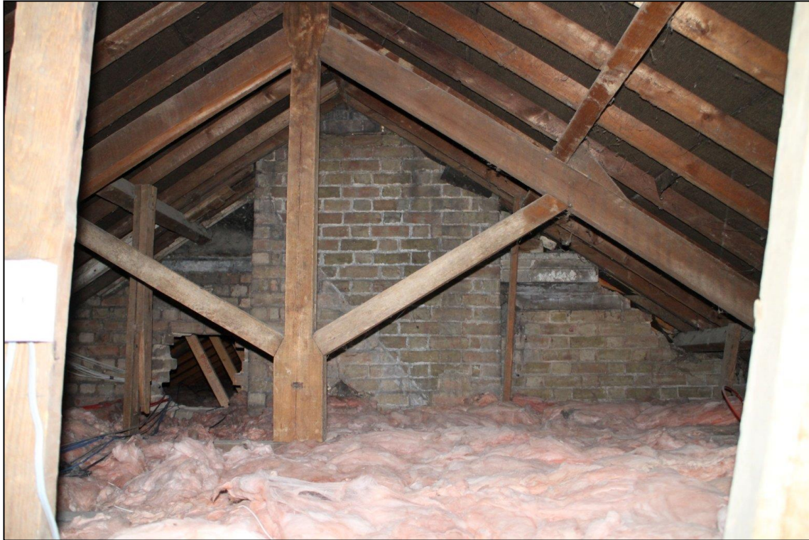
Image 29: Roof space above bedrooms 6, 7 and 8
