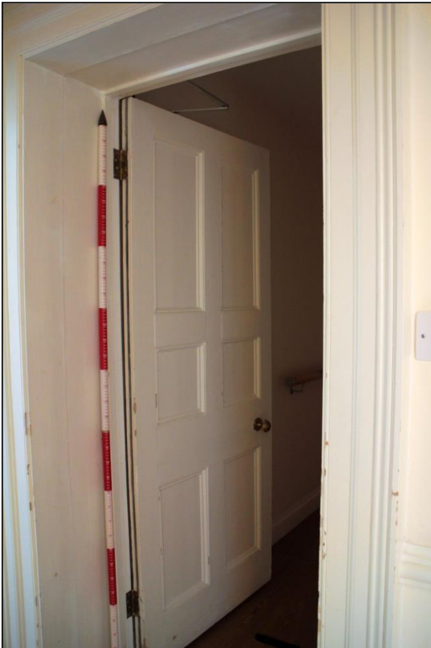
Image 24: Corridor adjacent to Room 20 Shows 19th century door case and six-panel door
