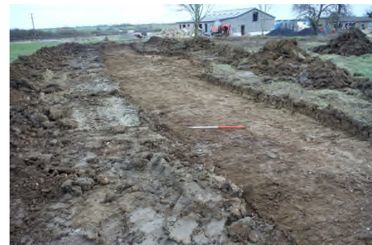
Image 3: External dump (2) and passing bay at E extent of strip; looking SE. Scale 1m.
