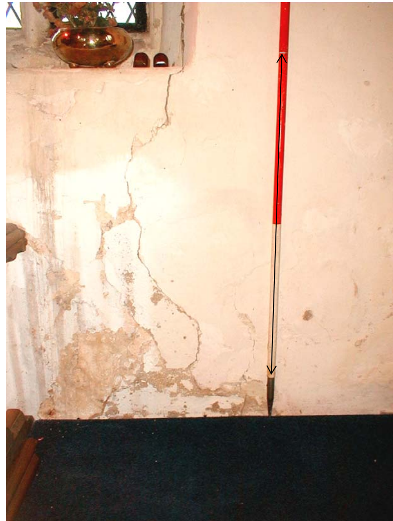
Figure 4: Photographs illustrating interior damage to north wall of chancel (arrowed lines = 1.00m).
