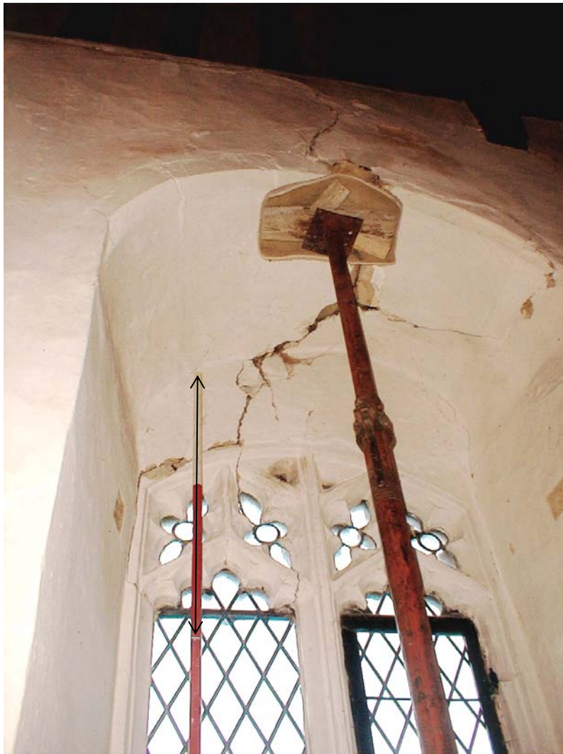
Figure 4: Photographs illustrating interior damage to north wall of chancel (arrowed lines = 1.00m).
