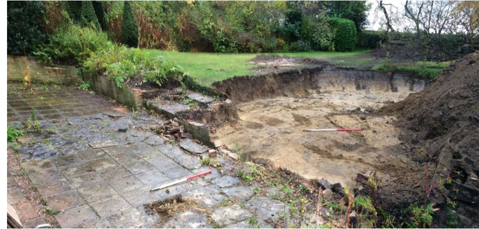
SW trench prior to removal of patio, looking south (scale 1m)
