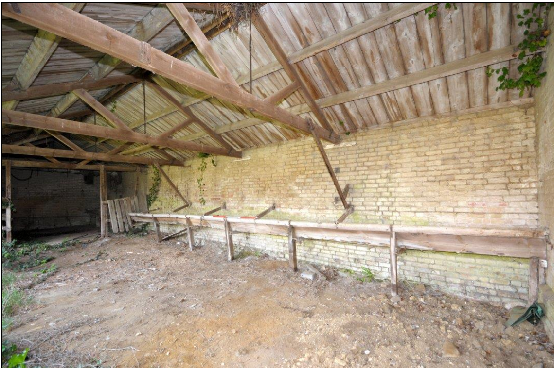
Image 24: East range: C6, looking north-east
