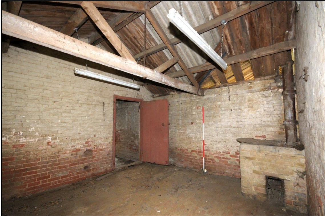
Image 29: East range: C9, looking south-west
