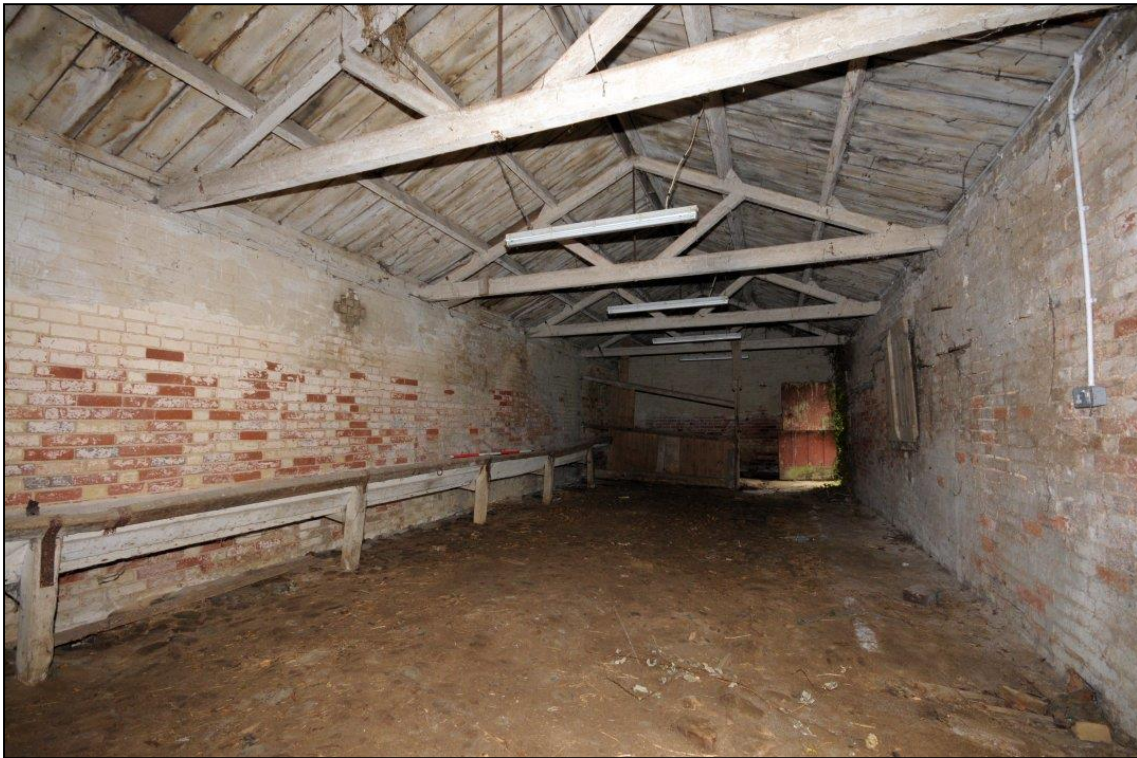
Image 9: South range: C2, looking west
