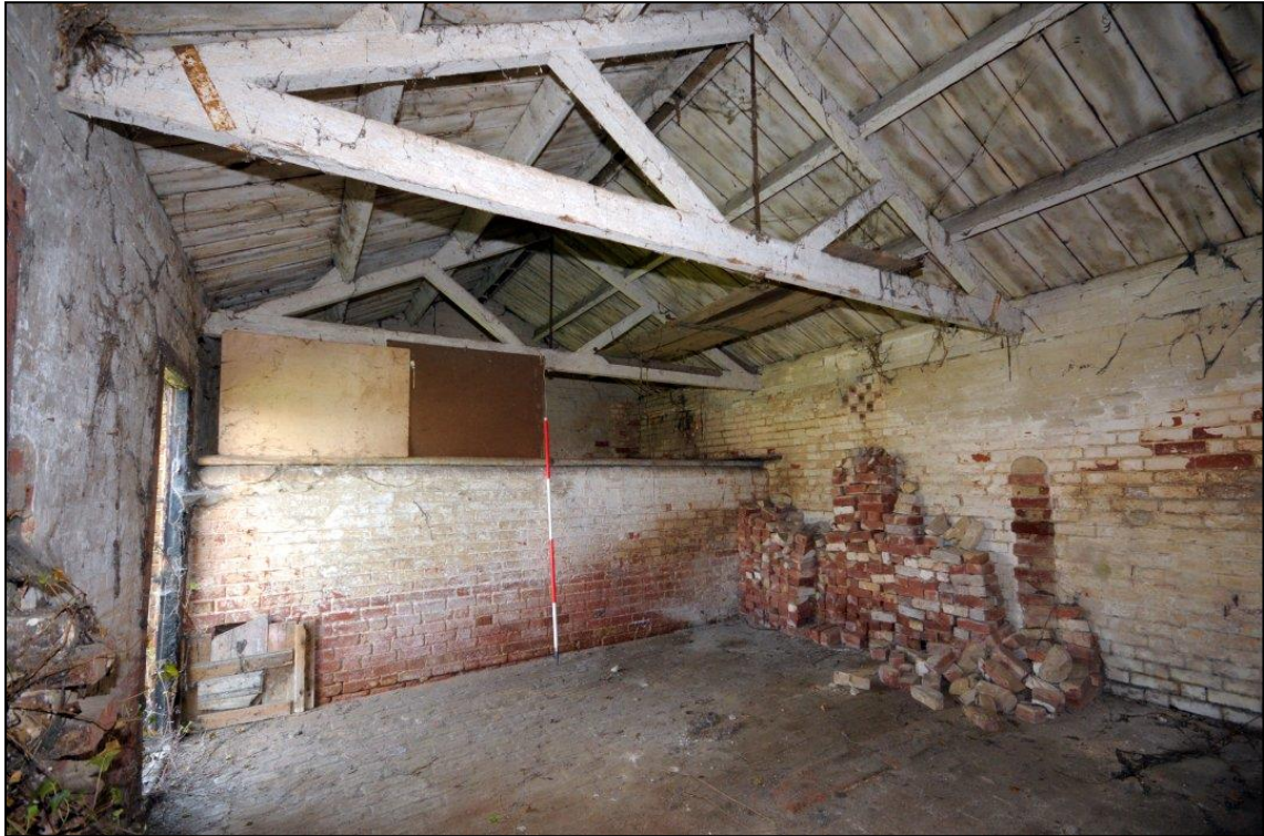
Image 27: East range: C7, looking north-east
