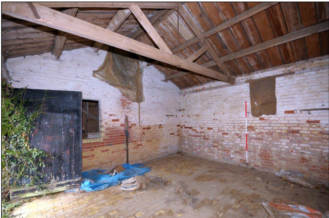
Image 14: South range: C4, looking south-east
