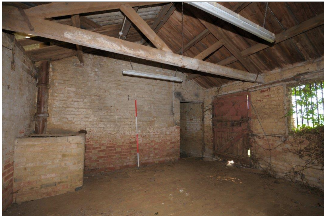
Image 30: East range: C9, looking north-east
