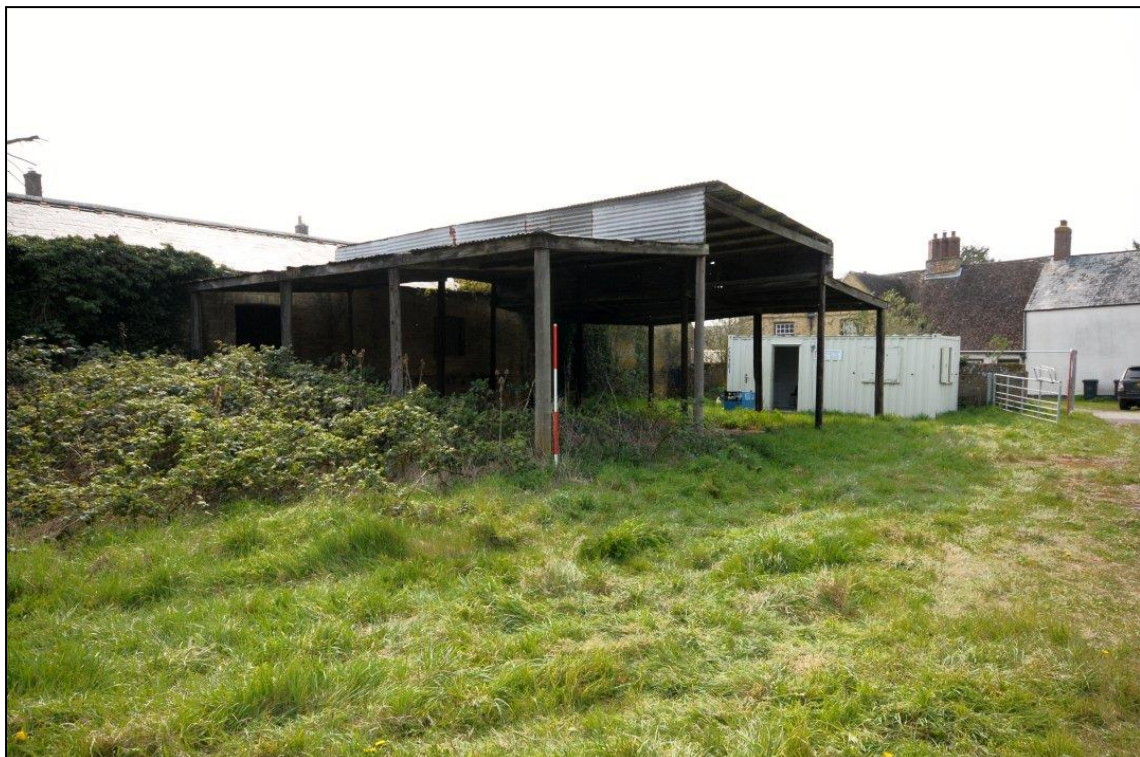
Image 6: South range: courtyard elevation, looking south-west
