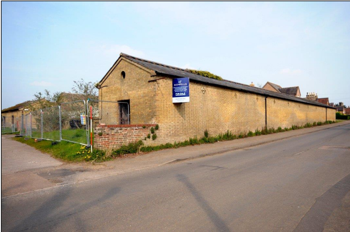
Image 3: South range: exterior elevation, looking north-east
