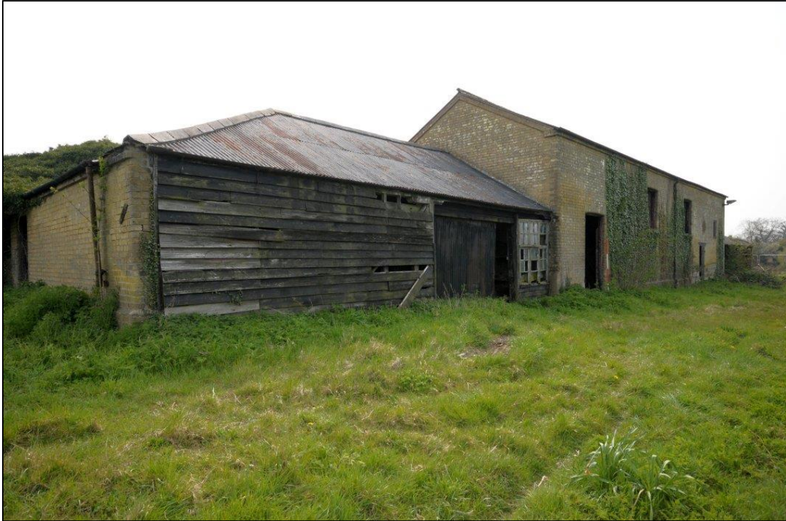
Image 33: North range, external elevation, looking south-west Showing compartment C10 in foreground
