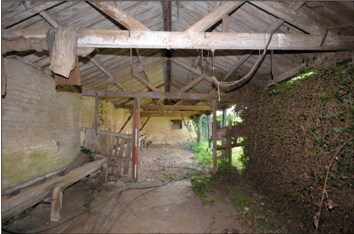
Image 25: East range: C6, looking south
