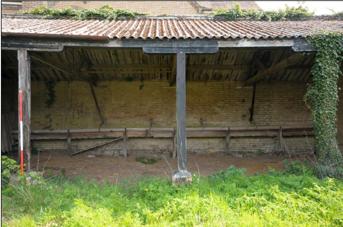
Image 23: East range, courtyard elevation: detail of C6
