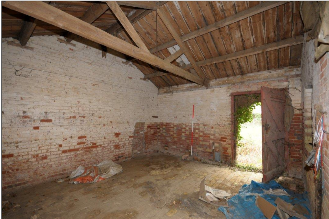
Image 15: South range: C4, looking north-west (Scale 2m)
