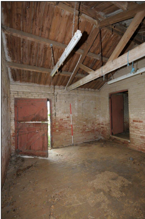
Image 28: East range: C8, looking north-west
