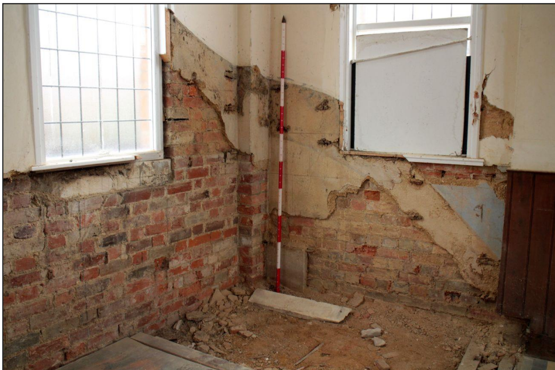
Image 16: Chapel, detail of south-east corner
