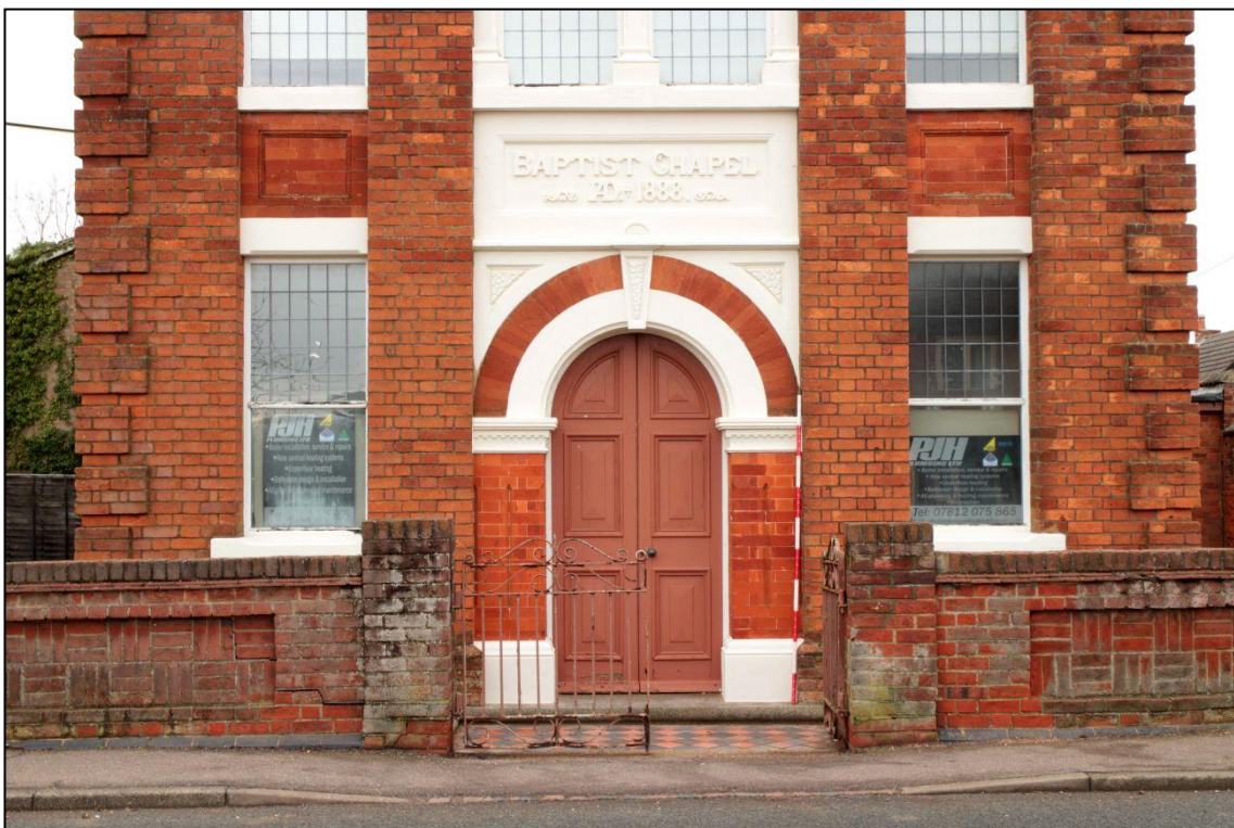
Image 6: South elevation, detail
