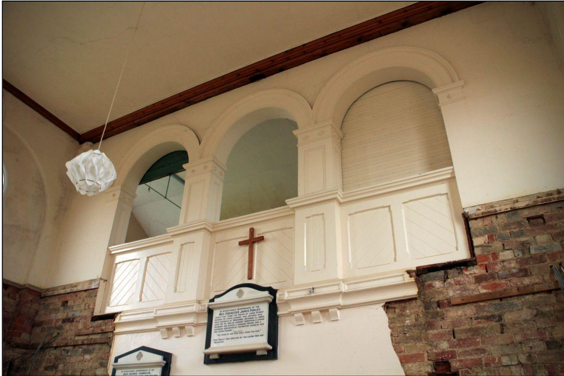
Image 15: Chapel, detail of north wall
