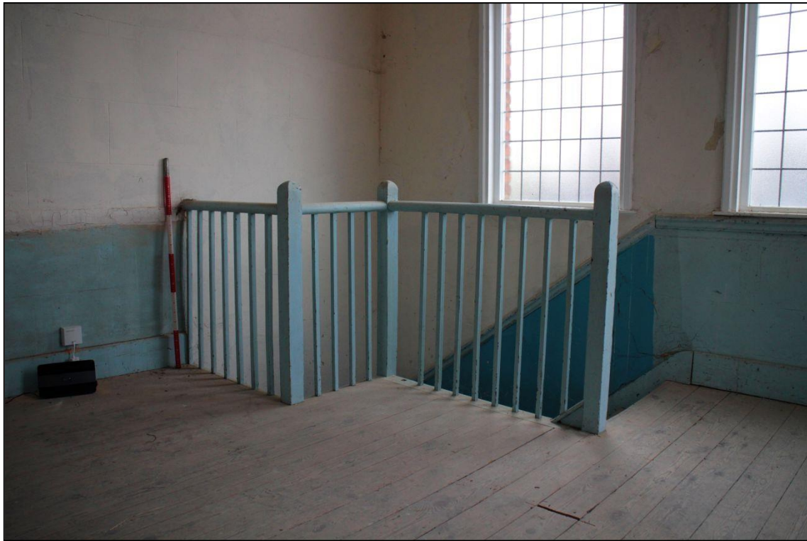
Image 35: Upper School Room, detail of stairs
