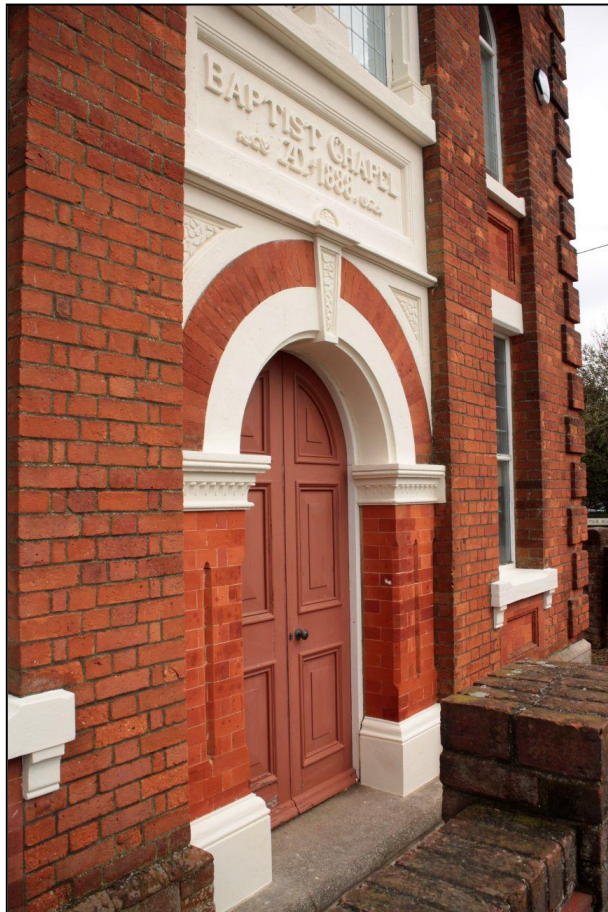
Image 7: South elevation, detail (oblique)
