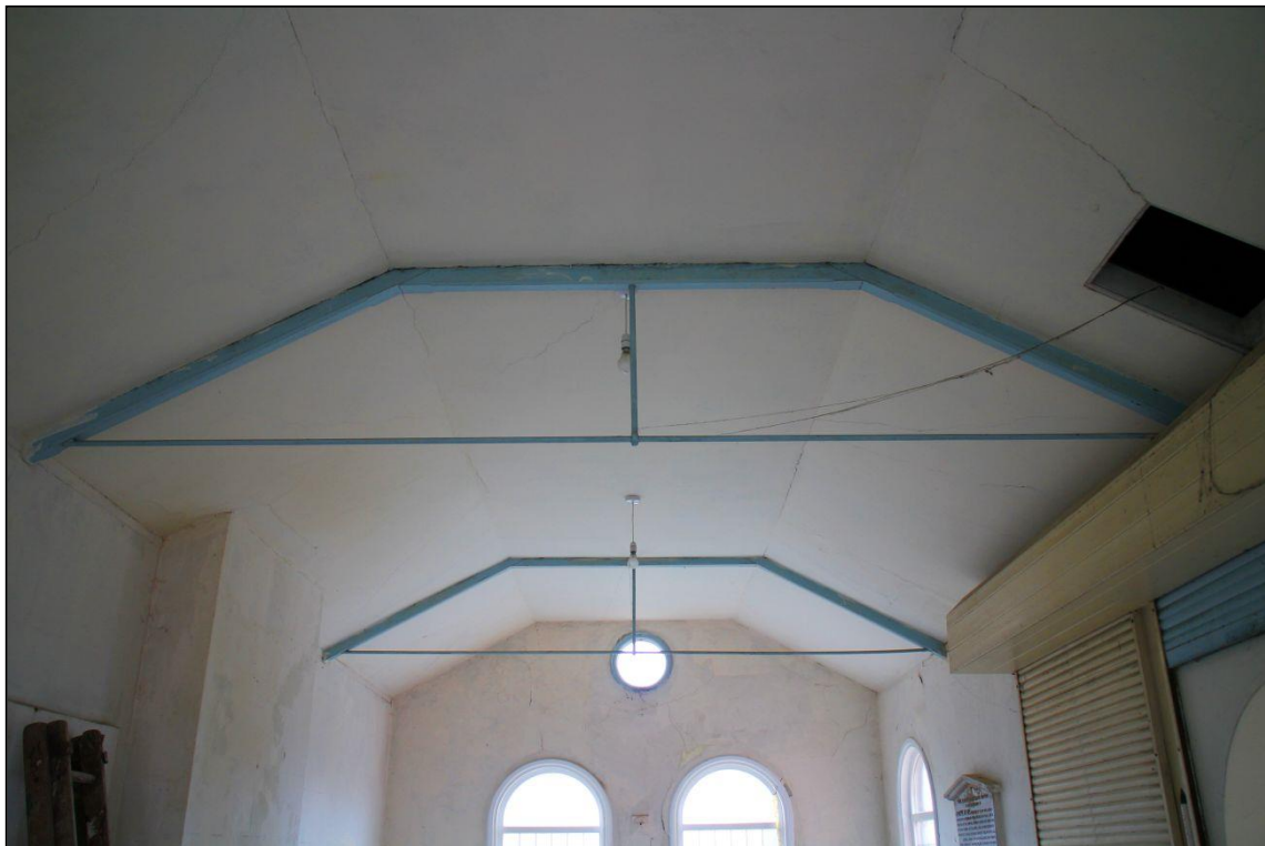
Image 34: Upper School Room, ceiling Looking east showing roof trusses with metal ties
