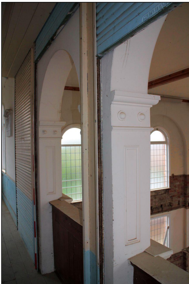
Image 37: Upper School Room, detail of arched openings
