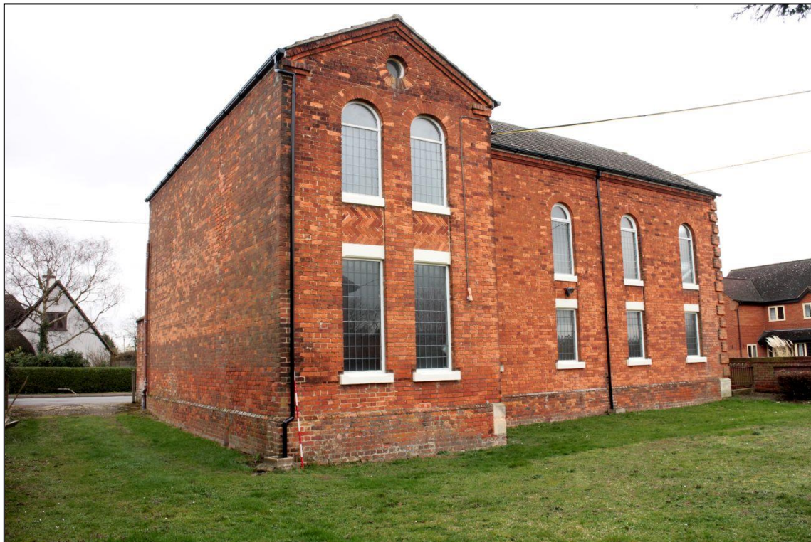
Image 4: Exterior from the north-west
