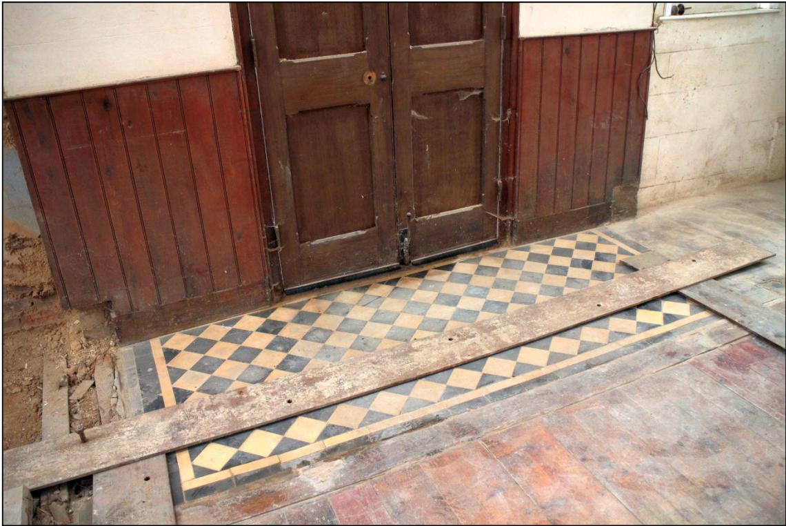
Image 17: Chapel, detail of front entrance
