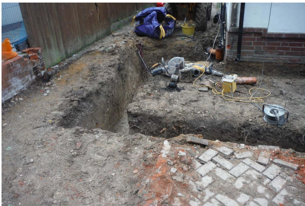
Foundation trenches at the southern end of the extension
