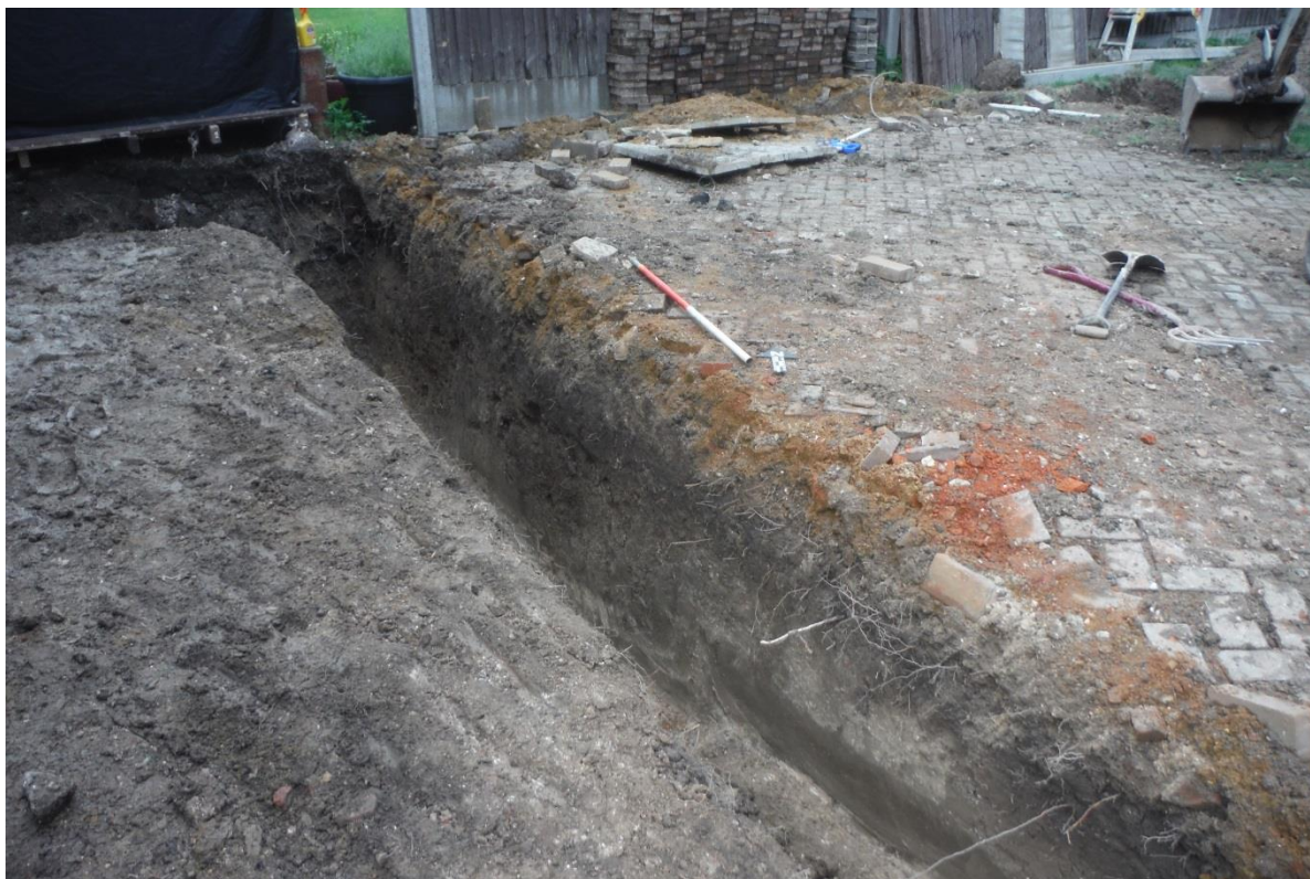
The eastern-most foundation trench (1m scale)
