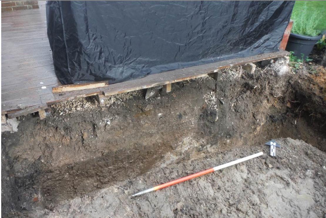
SE-facing section of northern-most foundation trench (1m scale)
