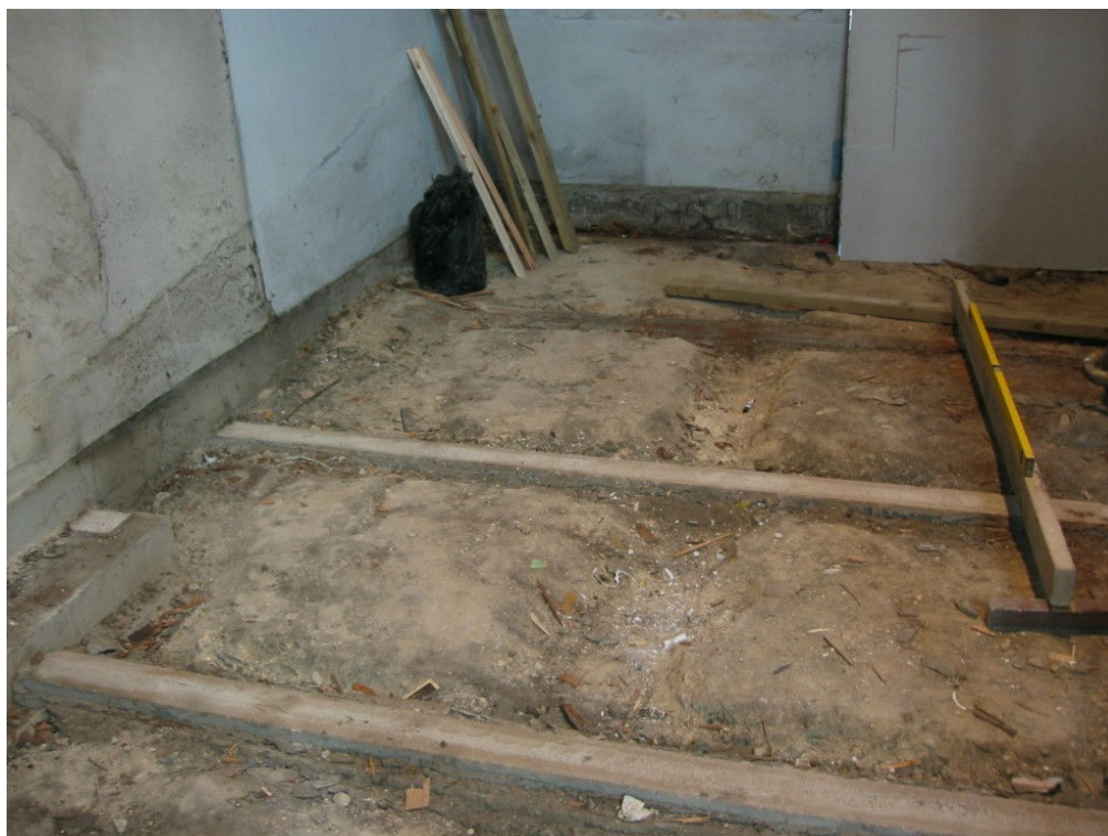
Stone base beneath tower floor
