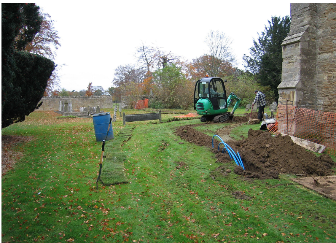
Excavation of the water main trench in progress
