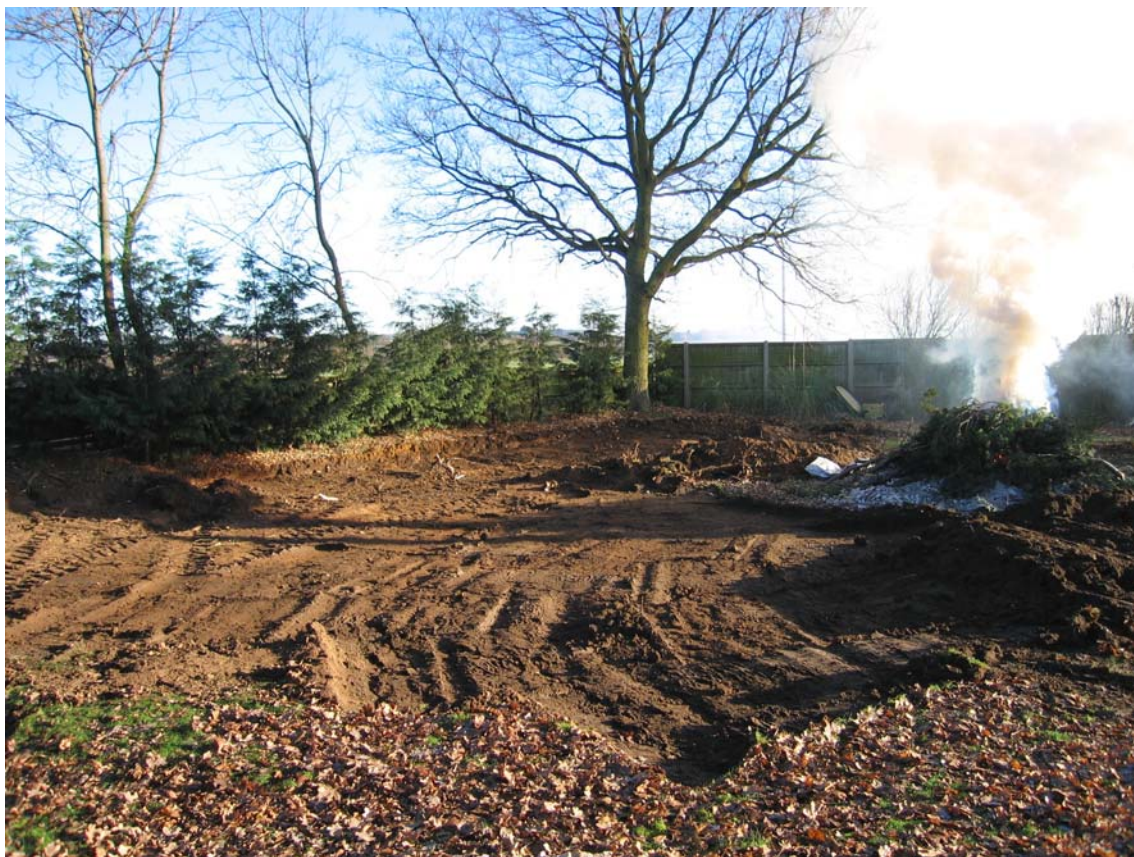
Figure 2: Northern end of site during ground-works
