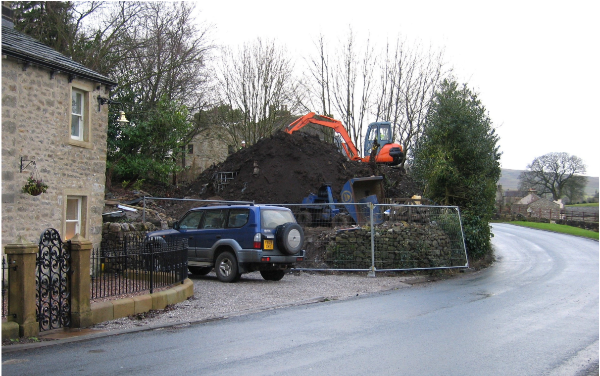
Photograph 3: Machining of Trench 2
