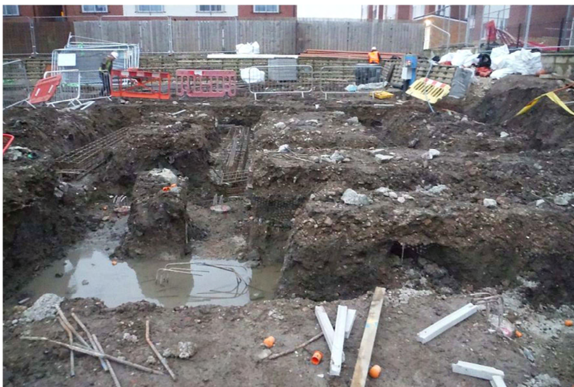
Photograph 17: Foundation trenches at the west end of the north wing, looking south-west; all exposed deposits comprise made ground, containing soil, brick rubble and other modern inclusions
