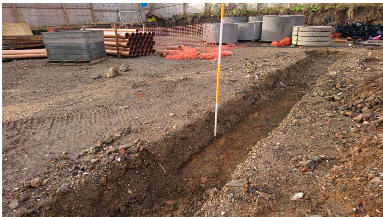
Photograph 8: Service trench north of south wing, looking south-west; top of natural sand and gravel at c.28.2m AOD
