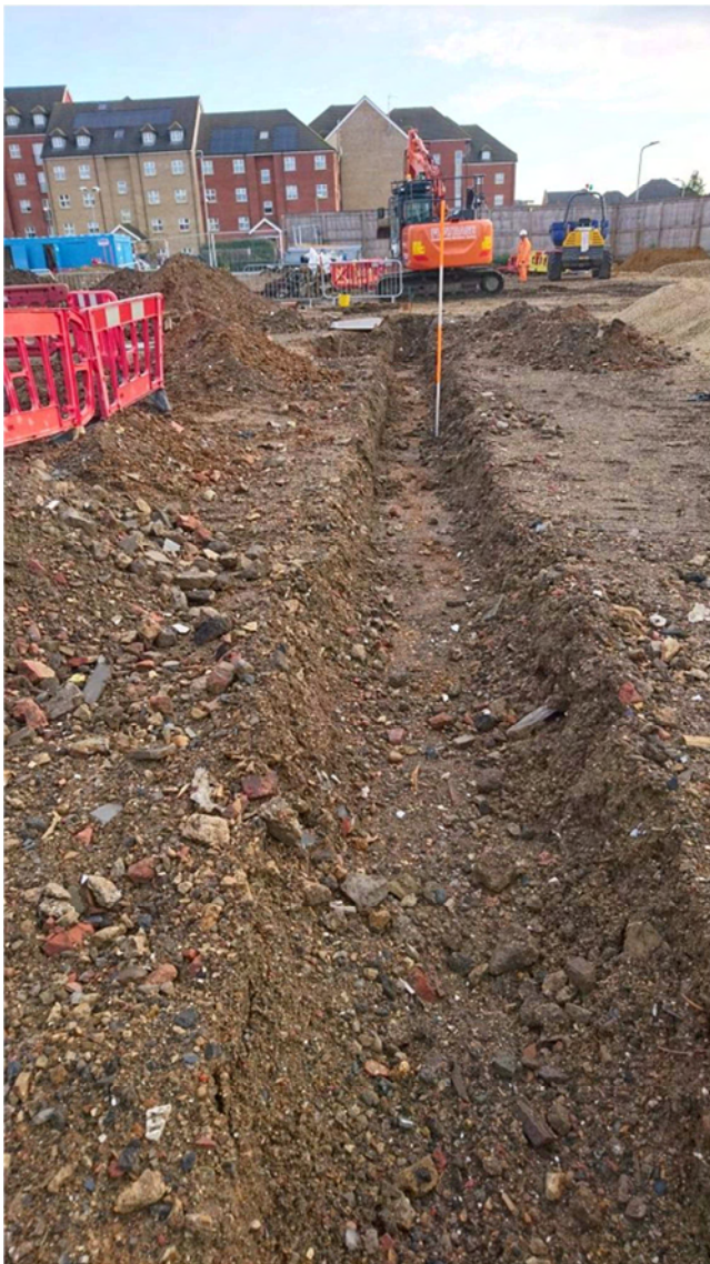
Photograph 9: Service trench, looking north-east.
