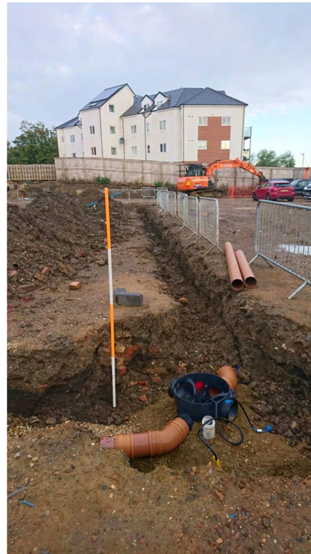
Photograph 10: Service trench in made ground, looking north-west
