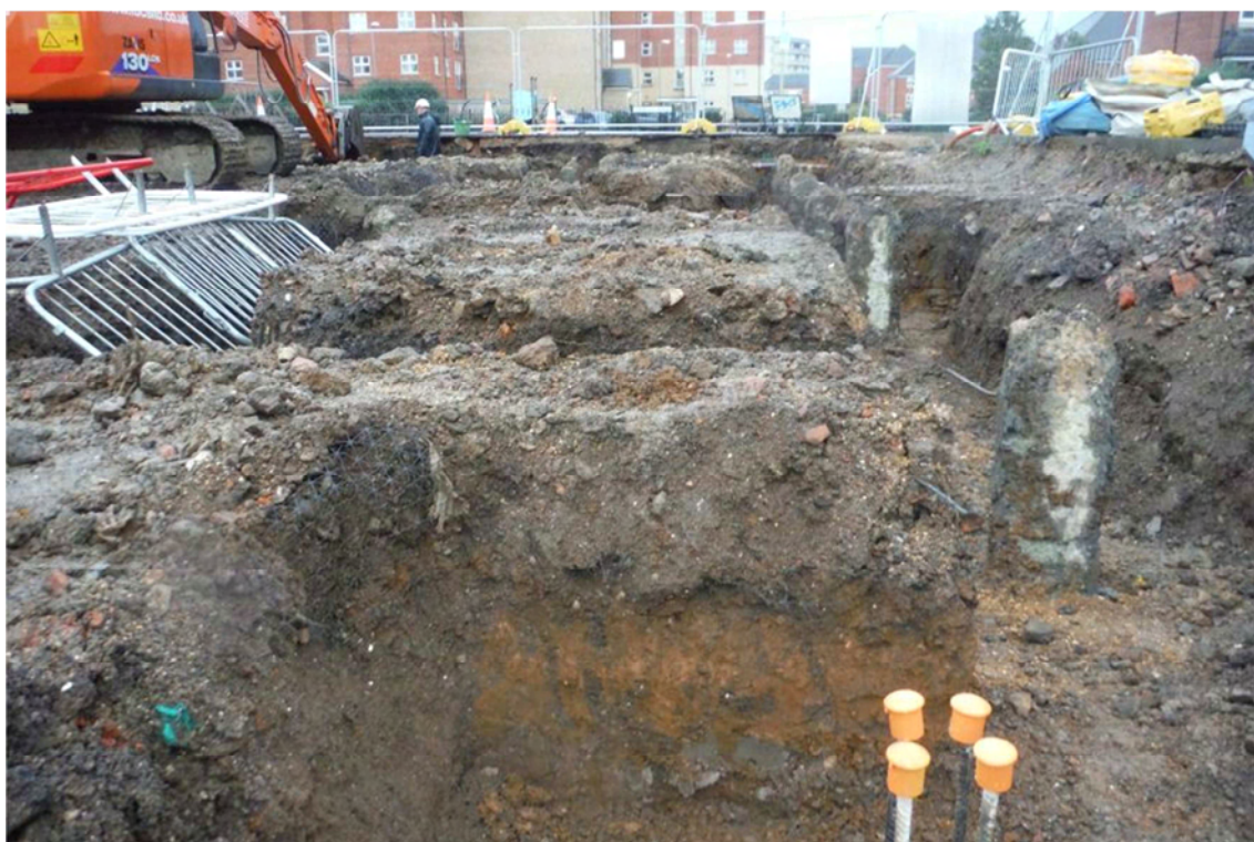
Photograph 2: South wing, looking along south-east side, some natural geology surviving at c.28.2m AOD (centre) but largely truncated to c.27.8m AOD (right)
