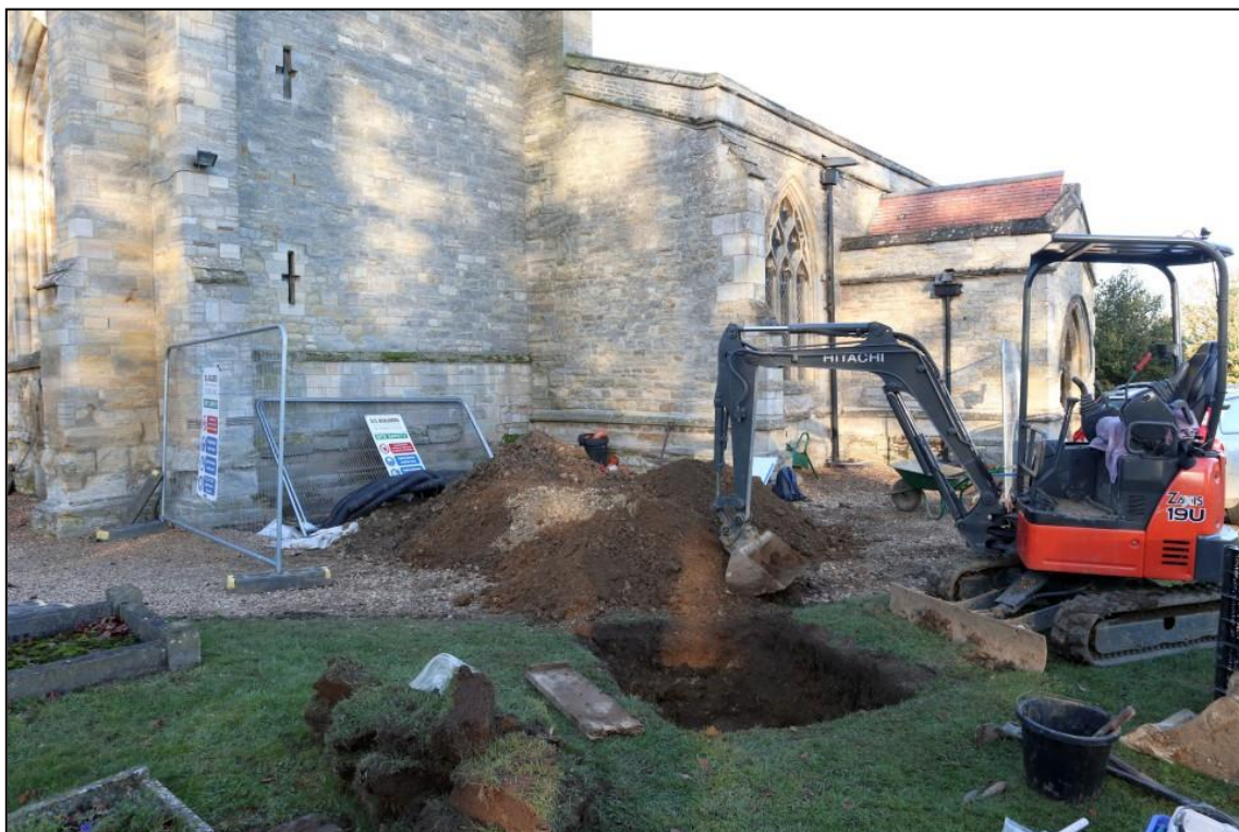
Image 27: Trench 4. Looking north-east
