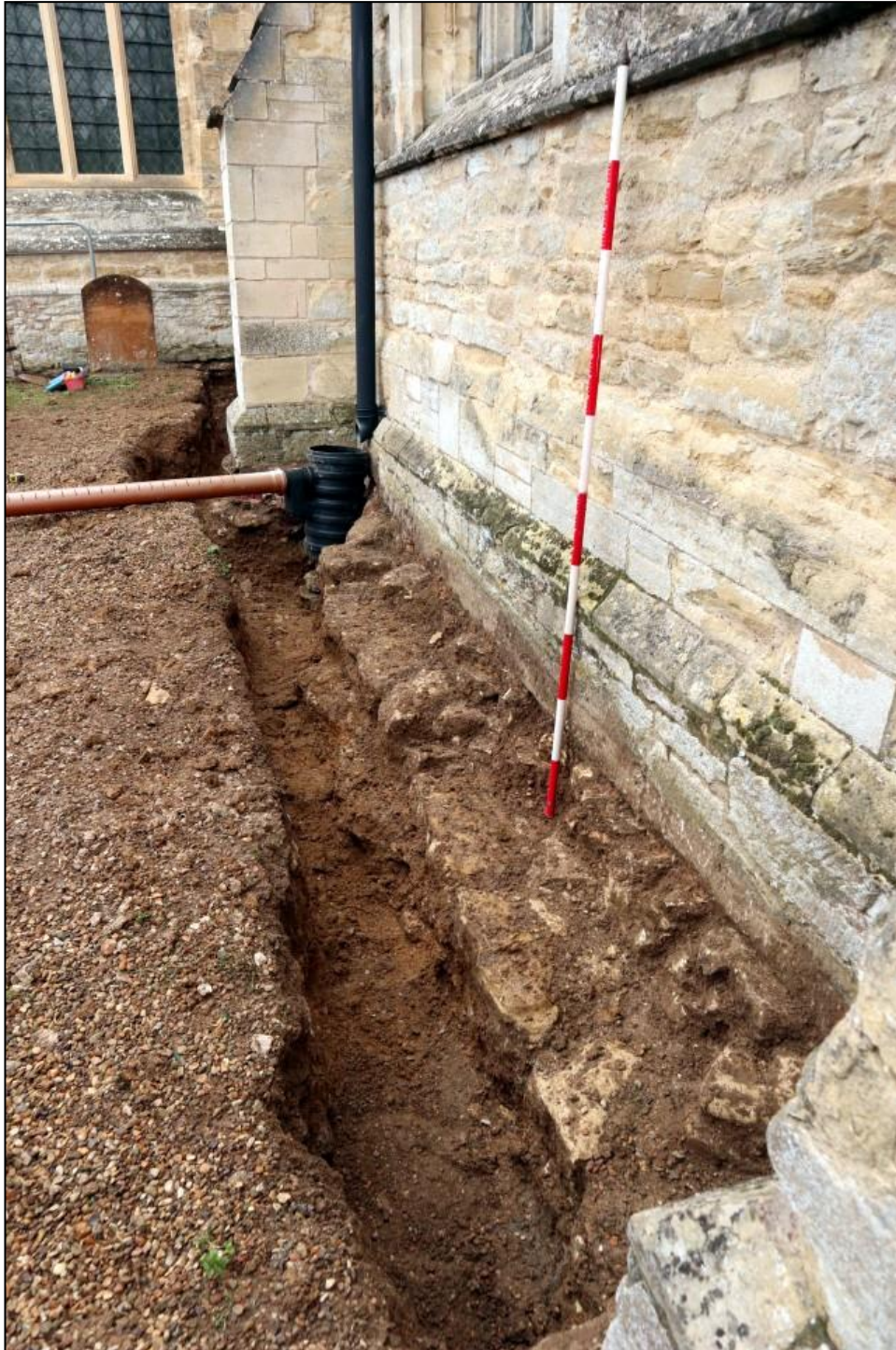
Image 19: Trench 1. Chancel, looking west
