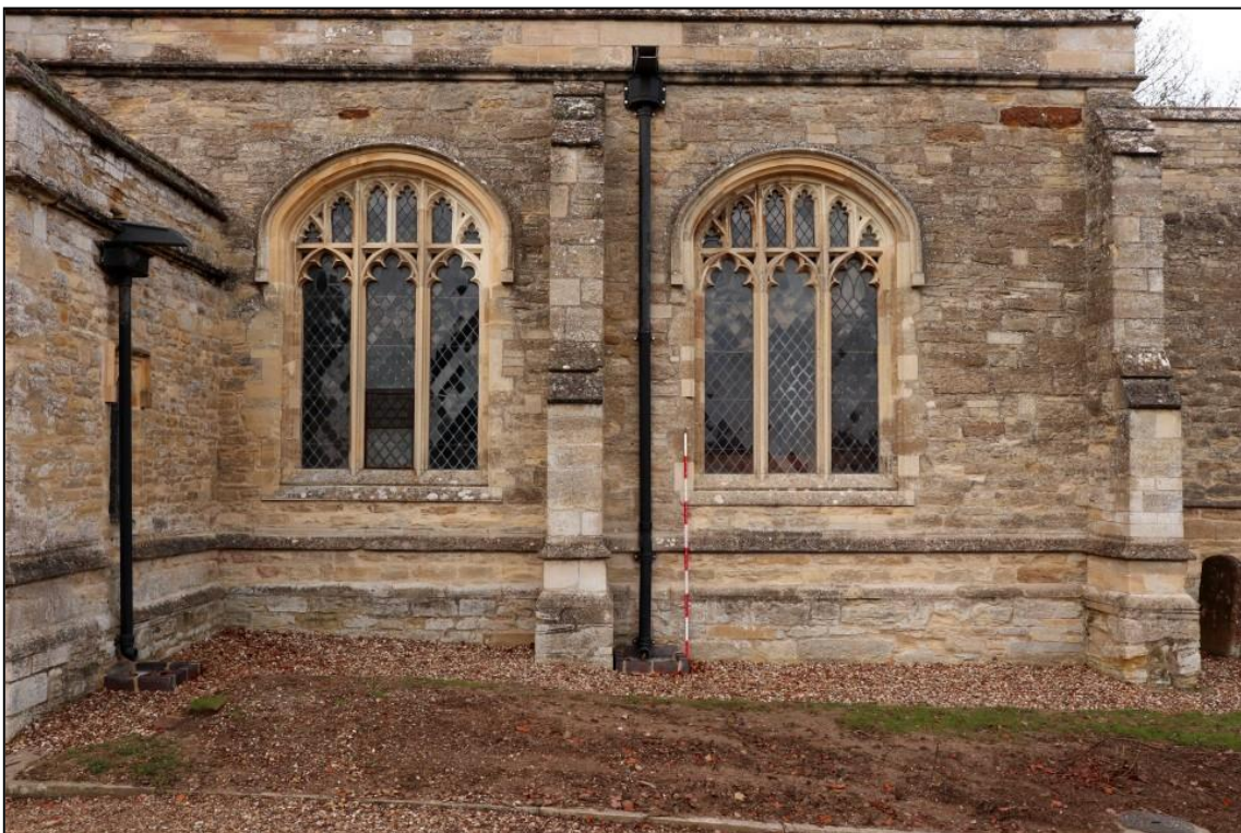
Image 4: South aisle Photographed following completion of French drain (Scale 2m)
