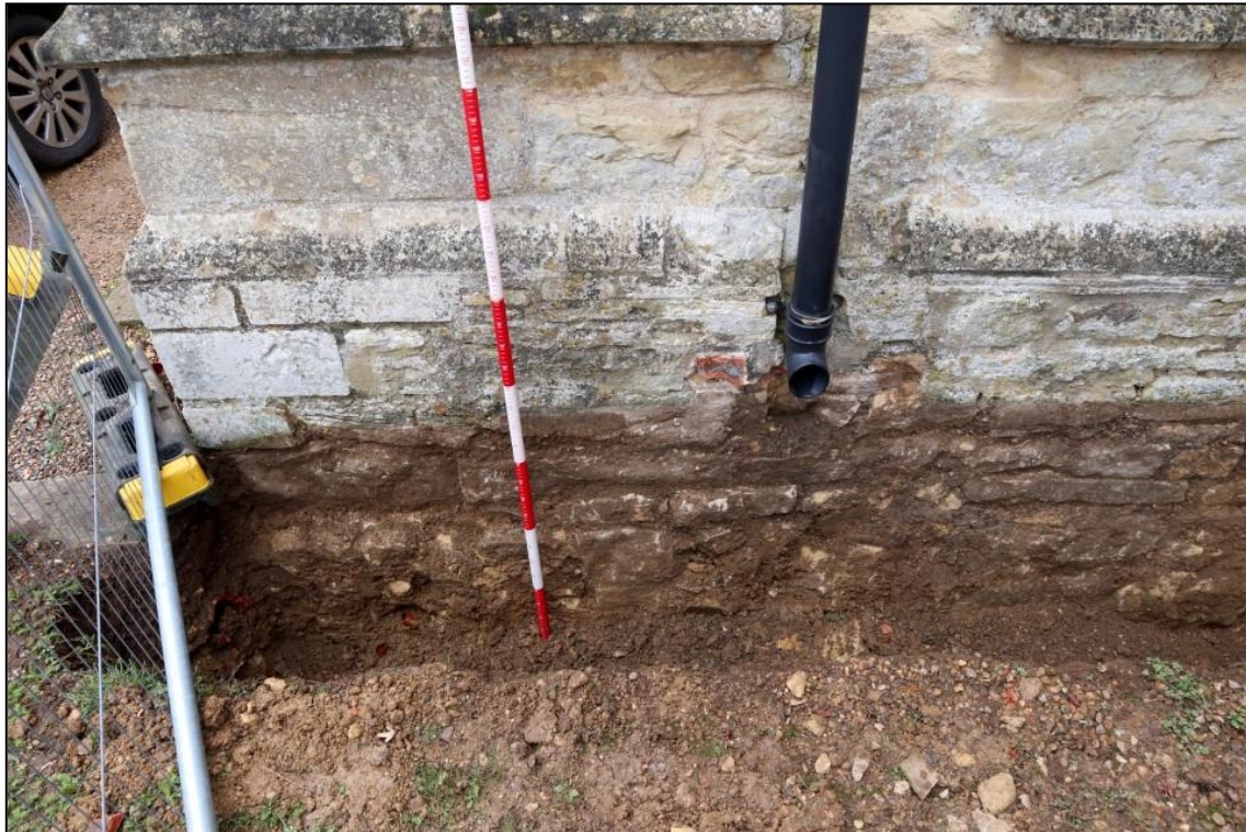
Image 2: Trench 1. East wall of south porch, left end (Scale 200mm divisions)
