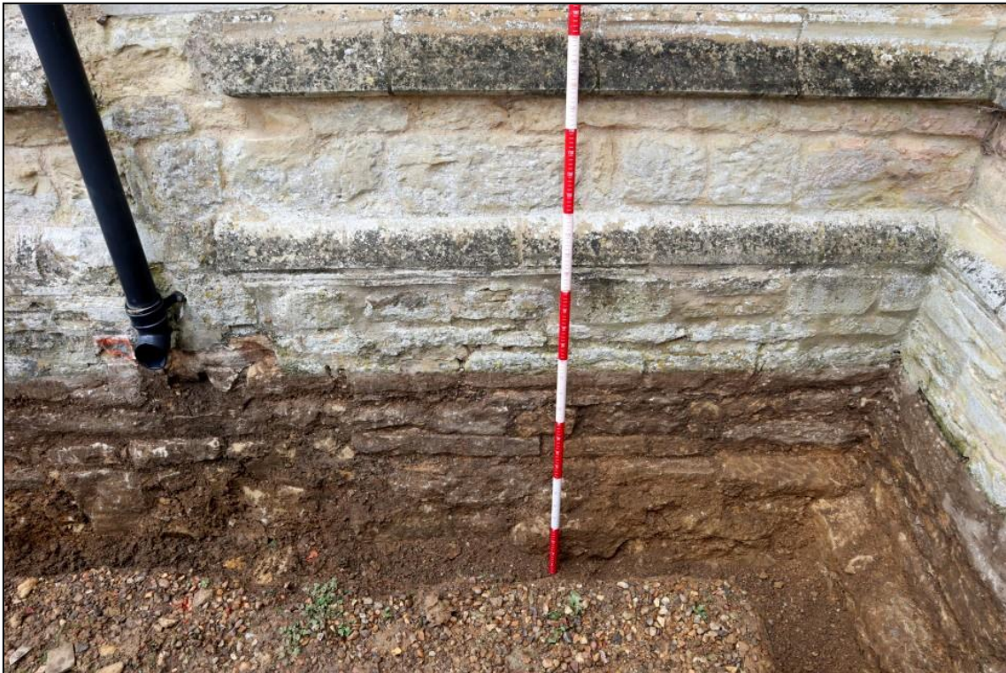
Image 3: Trench 1. East wall of south porch, right end (Scale 200mm divisions)
