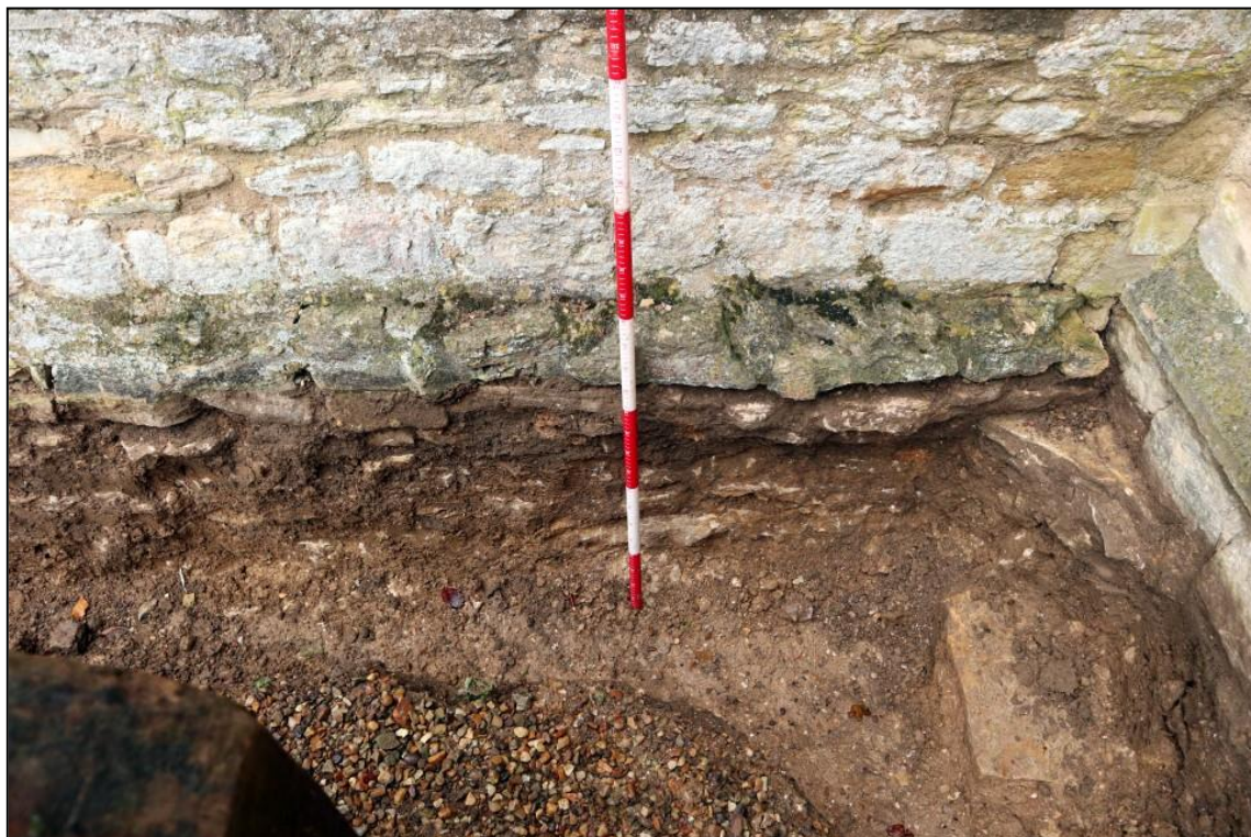
Image 14: Trench 1. East end of south aisle, right end Shows foundation offset; chancel wall at right (Scale 200mm divisions)
