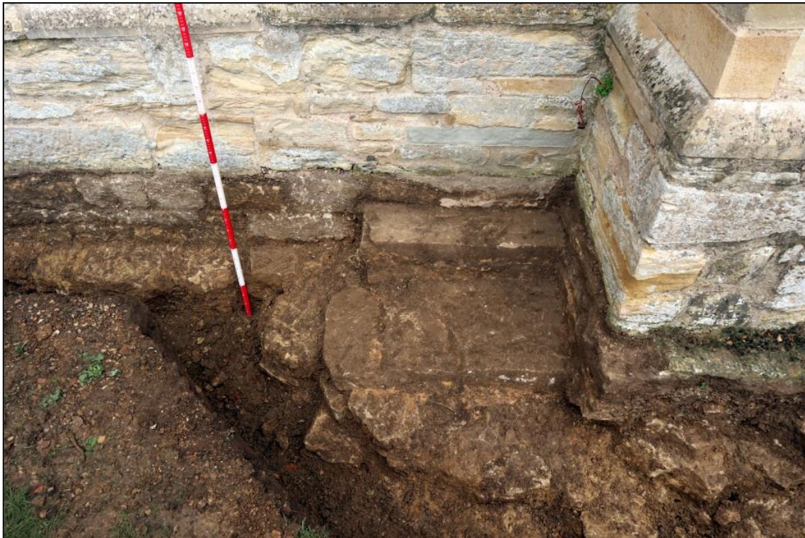
Image 9: Trench 1. South aisle, foundation pad at east end (Scale 200mm divisions)
