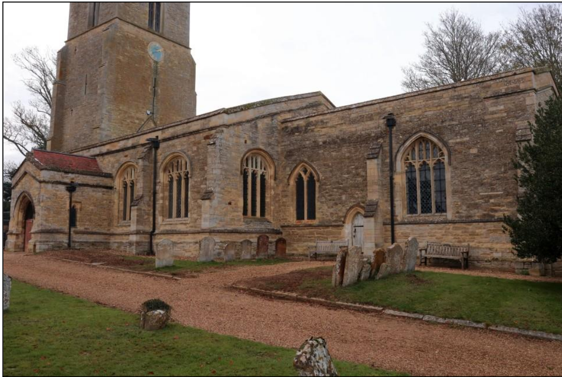
Image 1: General view of south side of church
