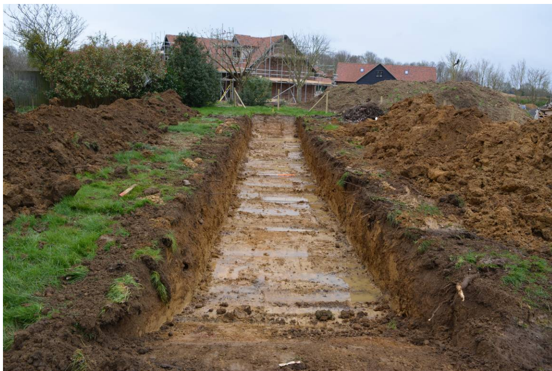
Figure 4: Photograph showing Trench 3 from the north-west
