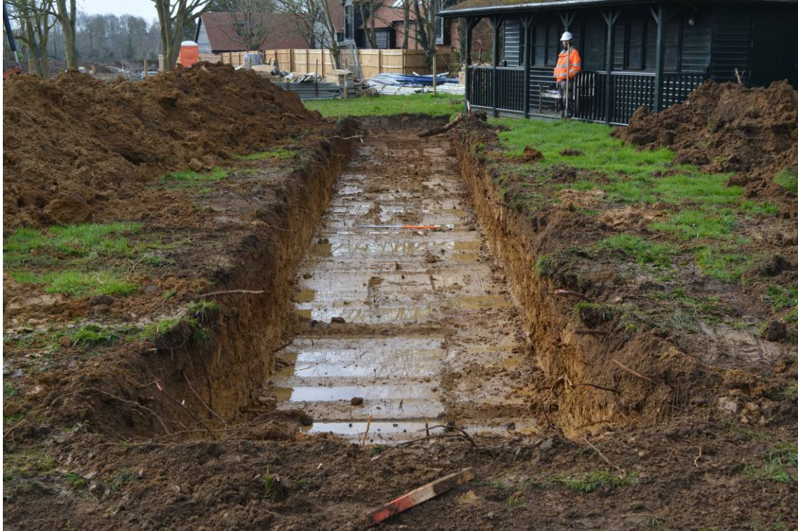
Figure 2: Photograph showing Trench 1 from the north-east
