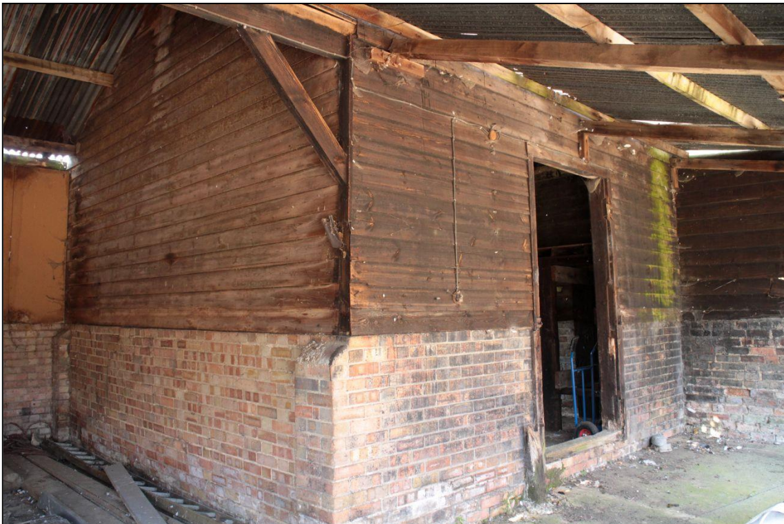
Image 28: South range, exterior of loose box
