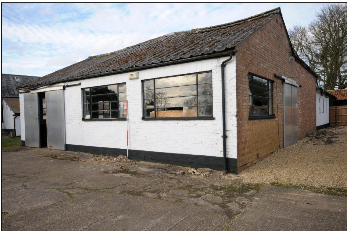
Image 34: Workshop range, south elevation Looking north-west (Scale 2m)
