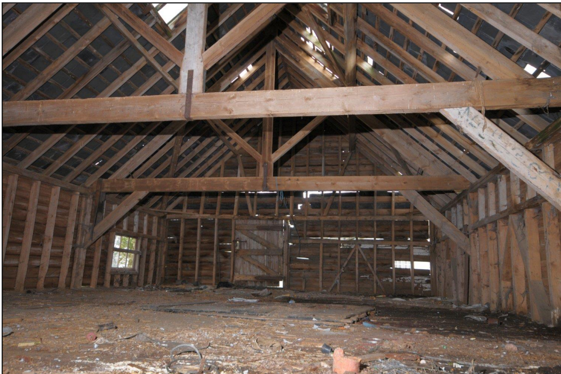
Image 24: Barn interior, loft
