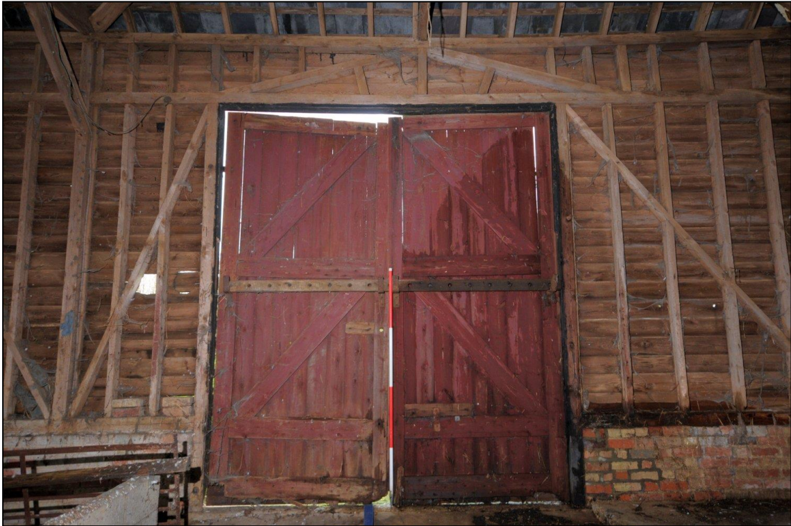
Image 13: Barn interior, double doors in west wall
