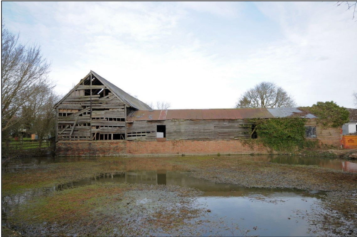
Image 3: South elevation of barn and south range
