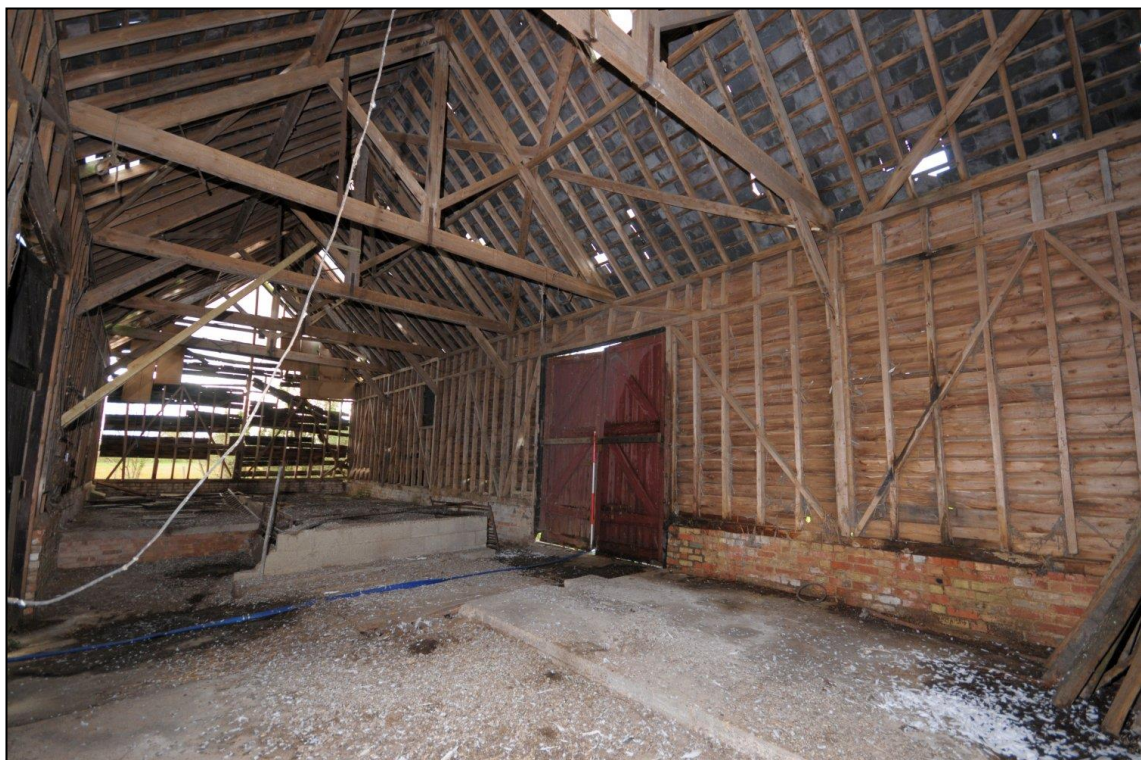
Image 10: Barn interior, looking south-west (Scale 2m)
