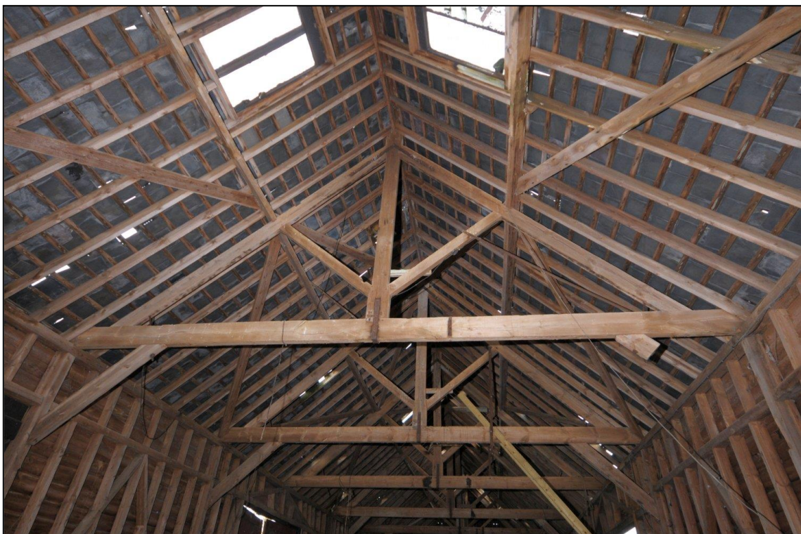
Image 16: Barn interior, roof
