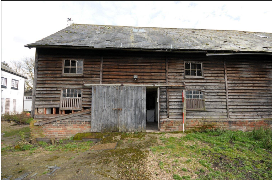
Image 5: Barn, left part of west elevation
