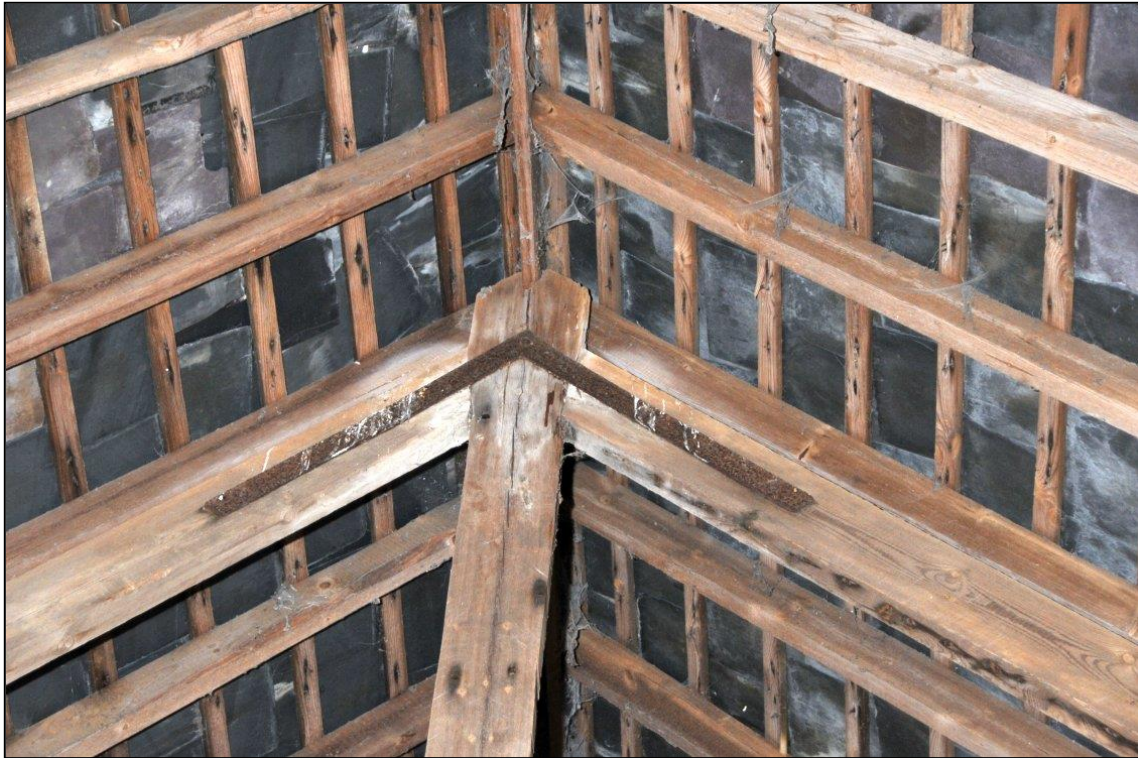
Image 19: Barn interior, detail of roof showing upper end of kingpost
