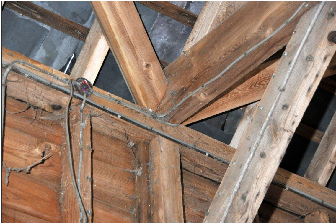
Image 15: Barn interior, detail of tie beam
