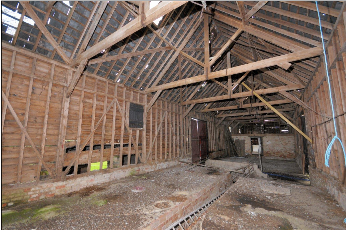
Image 11: Barn interior, looking north-west (Scale 2m)
