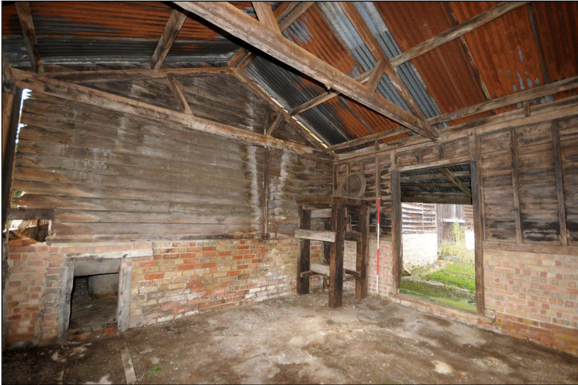
Image 29: South range, interior of loose box looking north-west Showing door at right and opening to grain-drying flue in barn wall at left (Scale 2m)
