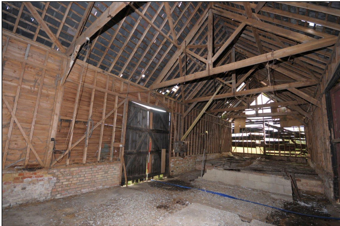
Image 9: Barn interior, looking south-east (Scale 2m)
