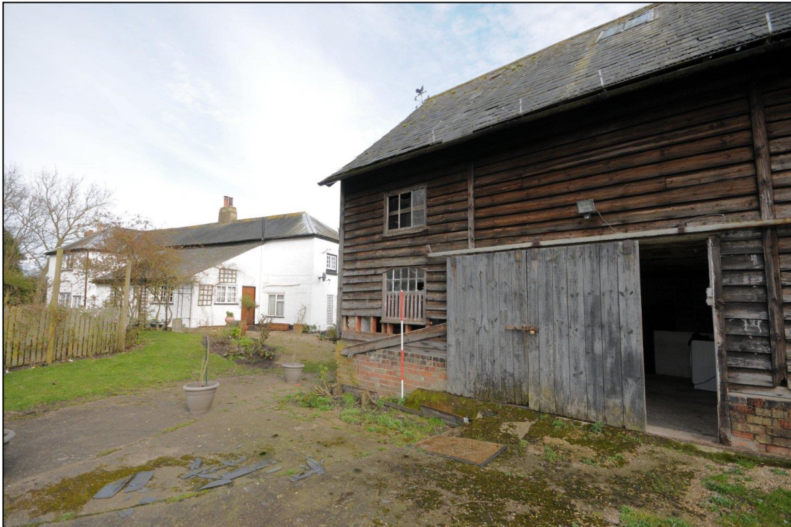
Image 1: Looking north-east showing barn and farmhouse
