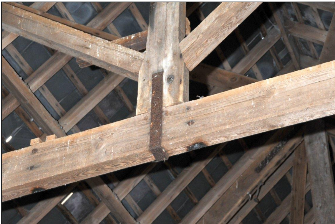
Image 18: Barn interior, detail of roof showing lower end of kingpost
