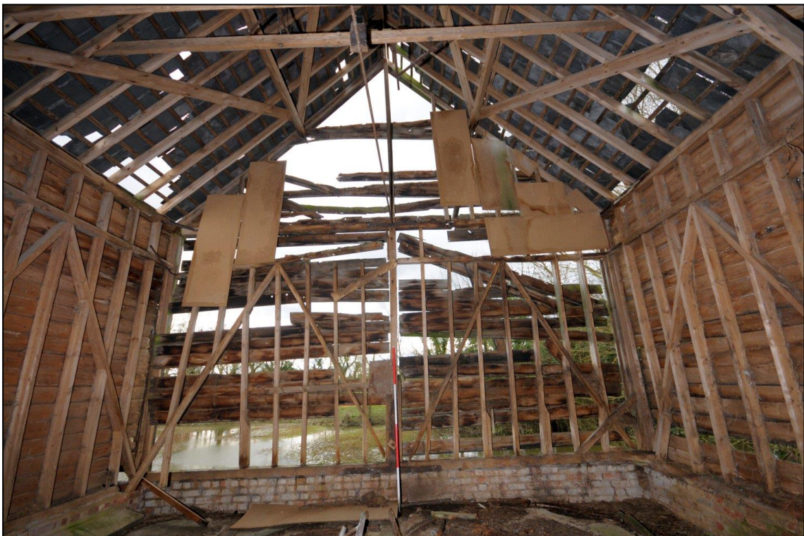
Image 14: Barn interior, south end wall
