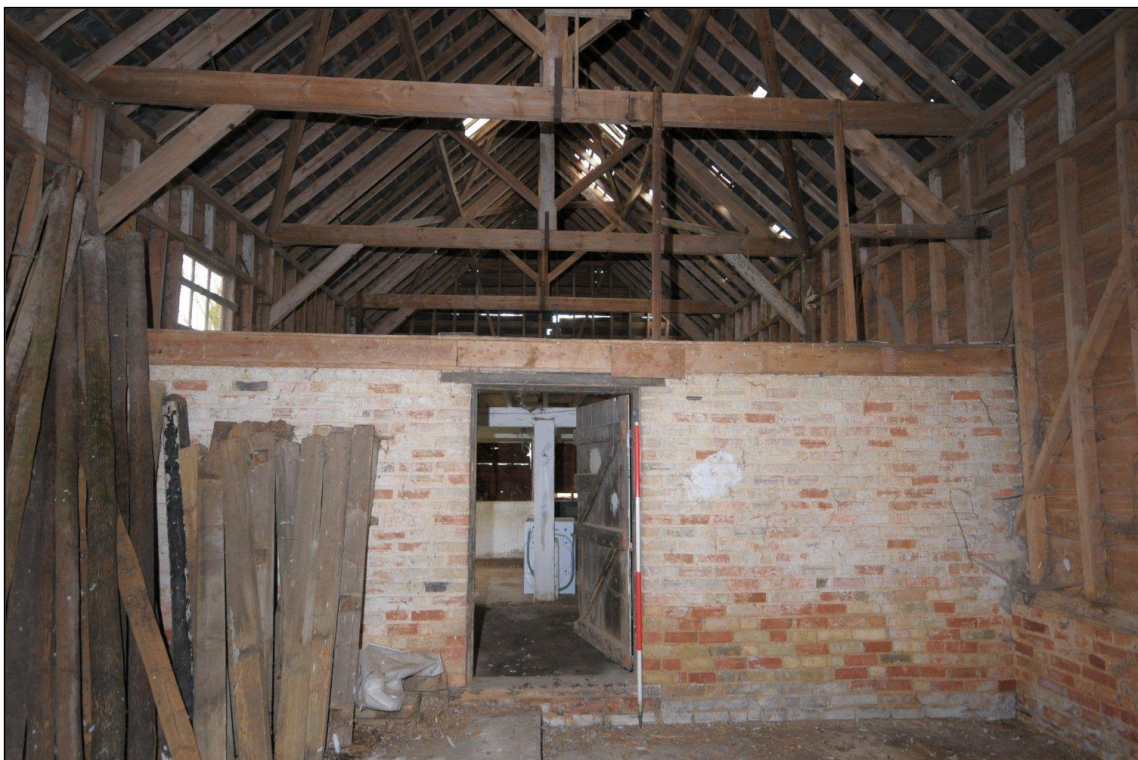
Image 20: Barn interior, brick partition wall
