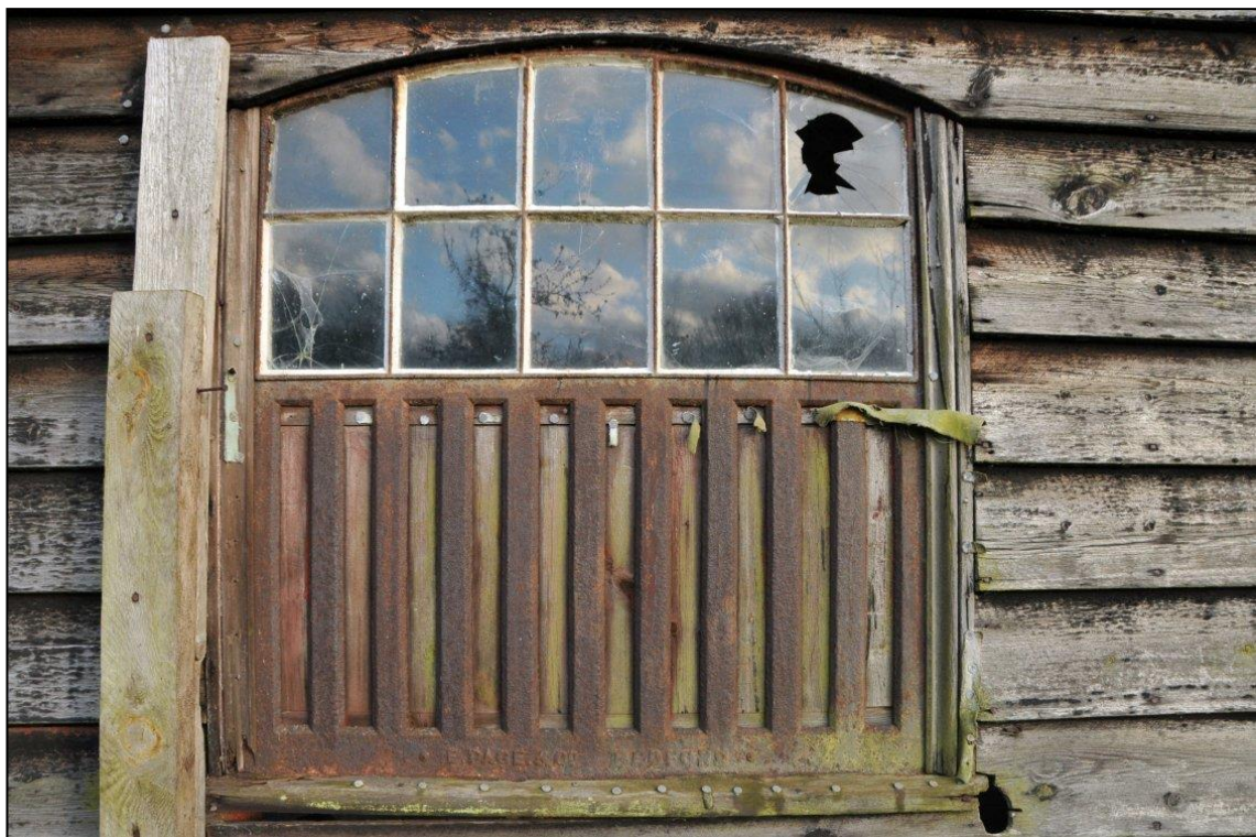
Image 6: Barn, ground-floor window in west elevation
