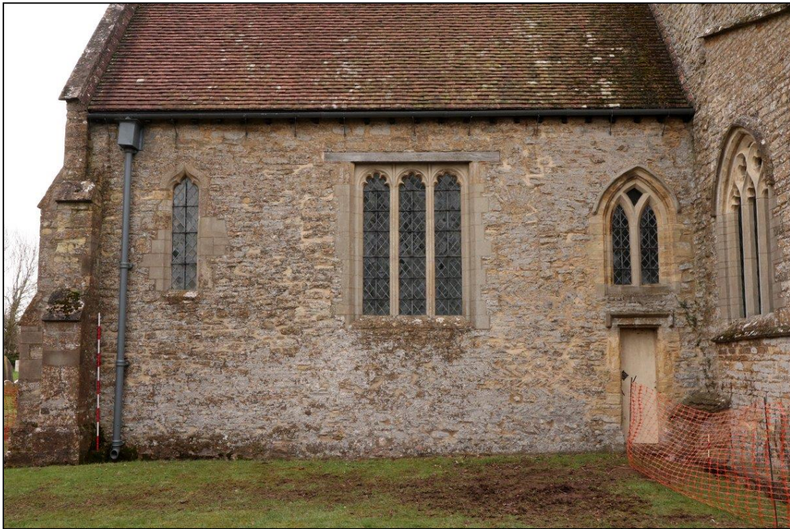
Image 9: South wall of chancel (scale 2m)
