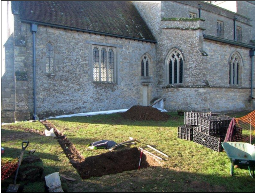
Image 25: Trench 3: general view showing trench location
