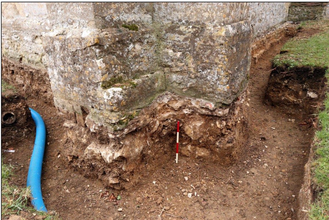
Image 8: Trench 1: north-east corner of chancel
