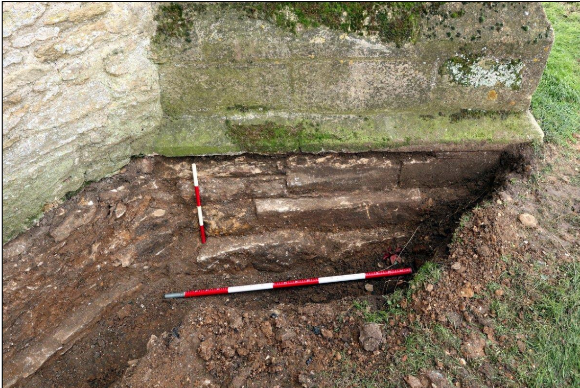
Image 21: Trench 1: north-west corner of tower Showing foundations (109) on north-east side of buttress (scales 1m and 0.4m)
