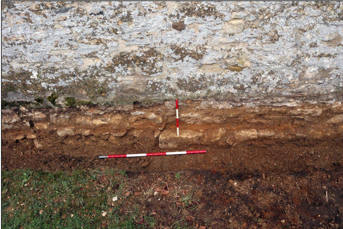
Image 11: Trench 1: south wall of chancel, eastern part
