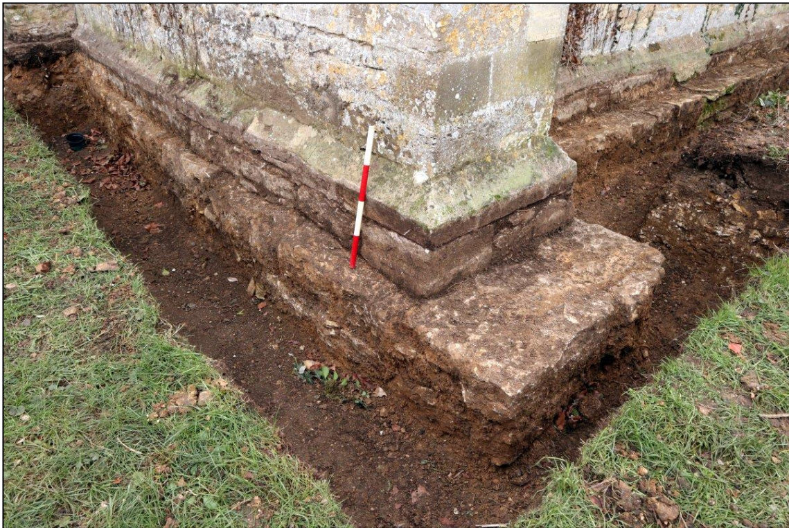
Image 14: Trench 1: north-east corner of north aisle
